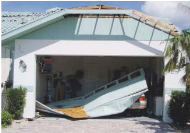
The lighter-duty garage door above succumbed to wind pressure, while the reinforced door at right held firm, despite taking a hit from flying debris.
