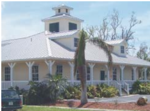
Structures built under Florida's new high-wind codes (left) fared much better than older buildings (below).
