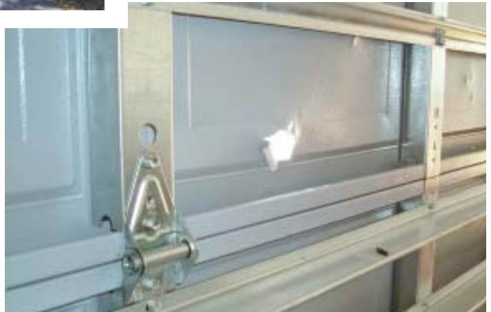
The lighter-duty garage door above succumbed to wind pressure, while the reinforced door at right held firm, despite taking a hit from flying debris.
