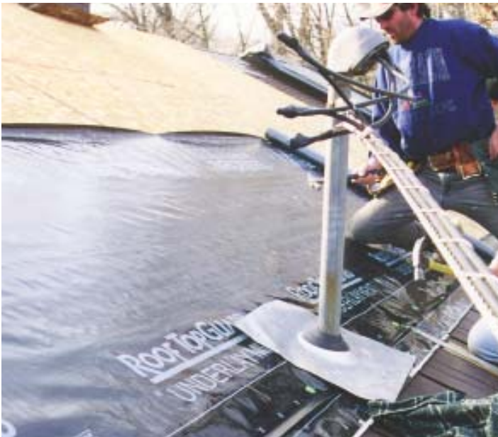
Figure 1. A proprietary underlayment is fastened to the deck with plastic-cap underlayment nails. Standard 30-pound felt also works, but the synthetic laminate is tougher, more durable, and easier to apply.
