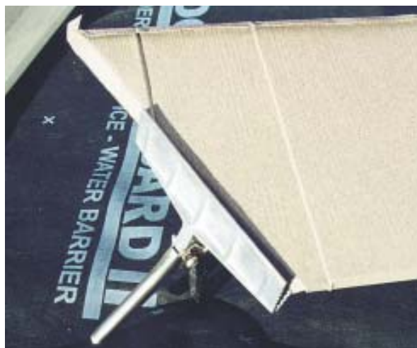
Figure 7. Shingles that adjoin a valley are cut with tin snips (above), and a flange is formed with a hand seamer or portable 2-foot brake (right). The valley flashing, like the shingles themselves, is fastened to the deck with metal clips (below).
