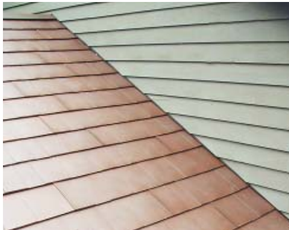
Figure 8. Like other special purpose flashings, sidewall flashing is fastened to the deck with clips; the vertical leg extends behind the siding and felt or housewrap (above). In reroofing applications, wood or vinyl siding is removed to install the flashing and replaced afterward (left). With three-coat stucco, the flashing channel, minus the vertical leg, is tucked into a slot cut in the stucco (below).
