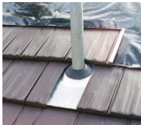
Figure 6. The edges of vent-stack flashings are turned up with a hand seamer to channel any wind-driven rain that gets past the surrounding shingles back to the outside (top left). Sometimes the vent flashing is not long enough to wrap around the bottom edge of the shingles below the stack. In that case, to effectively bond the lower edge of the vent flashing to the shingles, a site-bent piece of coil stock is hooked over the top flange of the full course below (top right). This is coated with sealant, and the flashing is pressed into place (middle). An additional sheet of underlayment adds protection. Finally, the vent flashing is covered by a notched shingle (above).
