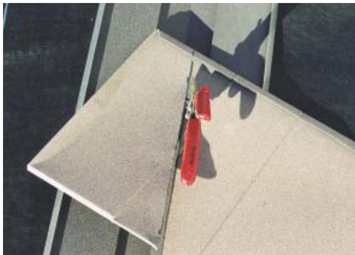
Figure 7. Shingles that adjoin a valley are cut with tin snips (above), and a flange is formed with a hand seamer or portable 2-foot brake (right). The valley flashing, like the shingles themselves, is fastened to the deck with metal clips (below).
