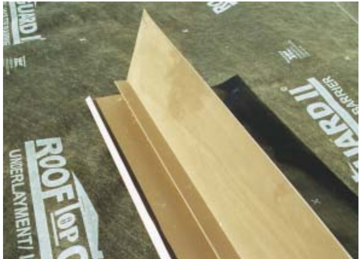
Figure 8. Like other special purpose flashings, sidewall flashing is fastened to the deck with clips; the vertical leg extends behind the siding and felt or housewrap (above). In reroofing applications, wood or vinyl siding is removed to install the flashing and replaced afterward (left). With three-coat stucco, the flashing channel, minus the vertical leg, is tucked into a slot cut in the stucco (below).
