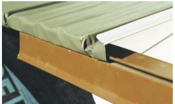
Figure 2. The first course of shingles is hooked against a combination of starter strip and drip-edge nailed to the deck.
