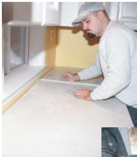
Figure 3. Sheet blanks for large or complicated countertops are scratch-marked in place on the cabinets. Complex countertop shapes are then produced in segments to be assembled and seamed in place.
