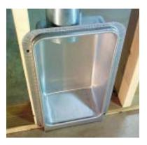
**Dryer Vent Solution.** Plastic dryer hose is a fire-hazard no-no. Flexible aluminum duct is safer but easily crumpled in the struggle to connect and position the appliance. The solution? The *Dryerbox*, an aluminized steel
