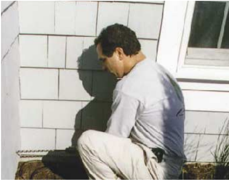
Figure 7. The author drills a hole at the base of the garage wall (above), then pulls 12-volt power supply and control wires through a watertight junction box (above right), and mounts a light-sensitive control switch on the box (right). The individual red, white, and black wires serve the photocell switch; the larger black cables entering the underside of the box carry power for the light circuits.
