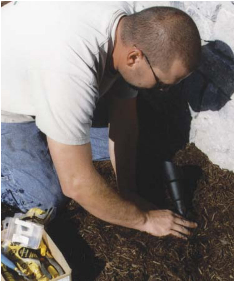
Figure 8. After pulling wire through a mounting stake and threading on the fixture (below), a worker sets the spotlight in the ground, angling it slightly to create shadows on a stone wall face.
