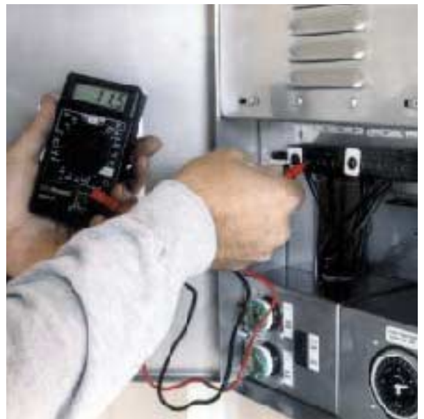
Figure 6. This 550-watt transformer box holds two 275-watt transformer banks, which the author can set independently to supply 12, 13, 14, or 15 volts. The author's control circuits typically use both a timer and a light-sensitive switch. At top left, he strips one of the wires that will link a timer mounted in the transformer box to an exterior-mounted light-sensitive switch, then mounts the timer into the box (top). After connecting the lighting circuits (above left), he runs a voltage check (above right).
