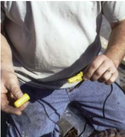
Figure 9. Landscape lighting circuits and fixtures are constantly exposed to weather and have to be able to withstand moisture. To protect wire splices, the author uses a two-piece fitting from Blazing Products (left) that uses an O-ring and a silicone-filled cap to seal out moisture. The author chooses MR (“metallic reflector”) lamps equipped with glass shields that protect the lamp from any drips of condensation that may form inside the weather-sealed lighting fixture. At right, he taps on a lamp’s glass protector shield.
