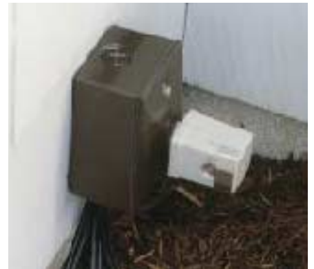
Figure 7. The author drills a hole at the base of the garage wall (above), then pulls 12-volt power supply and control wires through a watertight junction box (above right), and mounts a light-sensitive control switch on the box (right). The individual red, white, and black wires serve the photocell switch; the larger black cables entering the underside of the box carry power for the light circuits.
