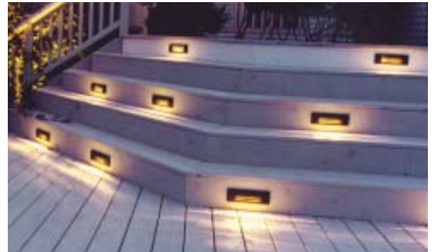
Figure 1. In the photo above right, a home's entrance is identified with canister spots that wash the base of the wall near the door, while specialty lights in the railing light the stairs. At right, recessed lights in the risers make for safer climbing.
