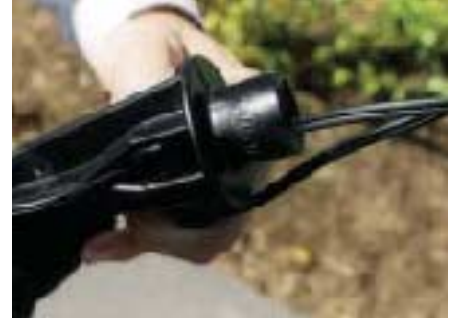
Figure 8. After pulling wire through a mounting stake and threading on the fixture (below), a worker sets the spotlight in the ground, angling it slightly to create shadows on a stone wall face.
