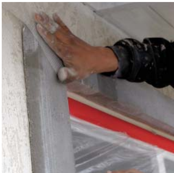
Figure 6. Joints between pieces of trim are reinforced with fiberglass mesh (left). A layer of Foam Tite is then applied over the mesh to fill voids and bond the pieces together (below).
