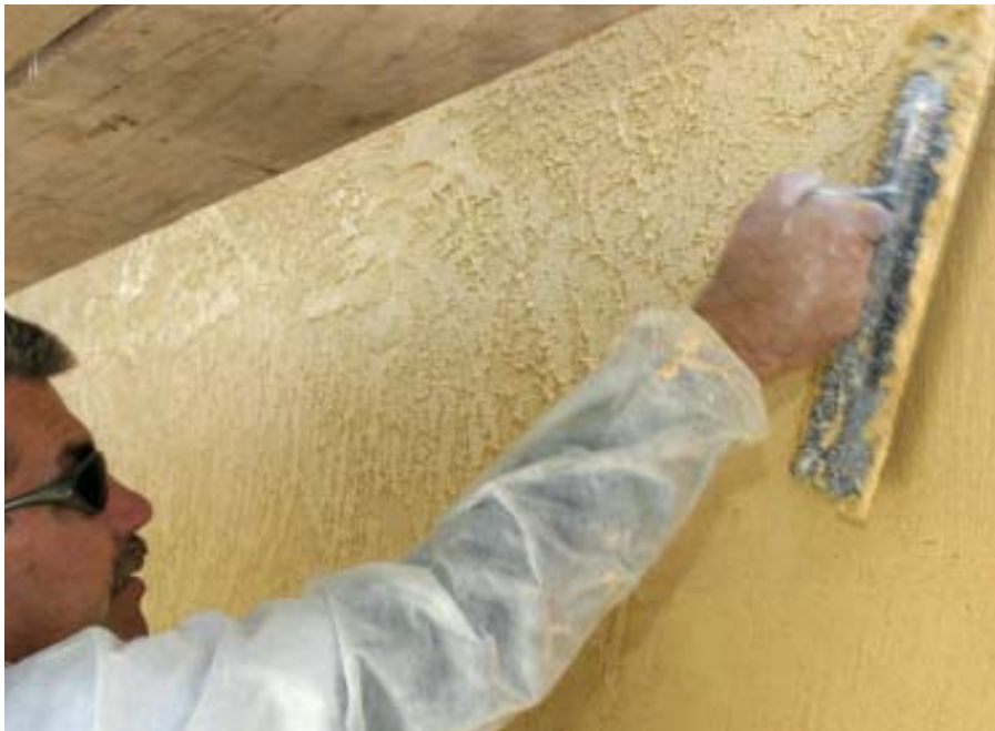
Figure 11. Here the author creates a skip-trowel finish by applying a second layer of color coat over a partially cured layer of the same material.
