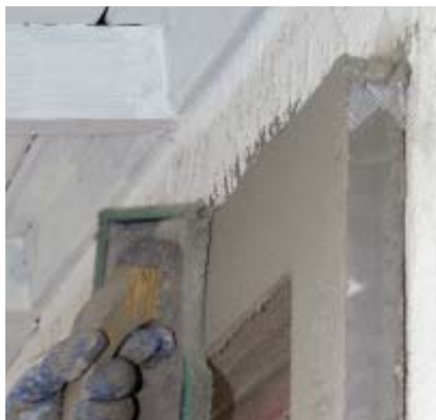
Figure 6. Joints between pieces of trim are reinforced with fiberglass mesh (left). A layer of Foam Tite is then applied over the mesh to fill voids and bond the pieces together (below).
