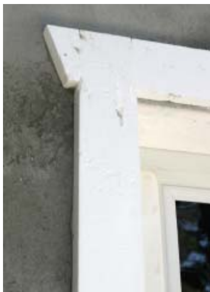
Figure 2. On this job, raw foam has been glued to the wall (left). It will be covered with fiberglass mesh and given a faux stone finish. It's faster to use precast foam; the material shown in the photo at right arrived on site with the mesh and a cementitious coating already on it.
