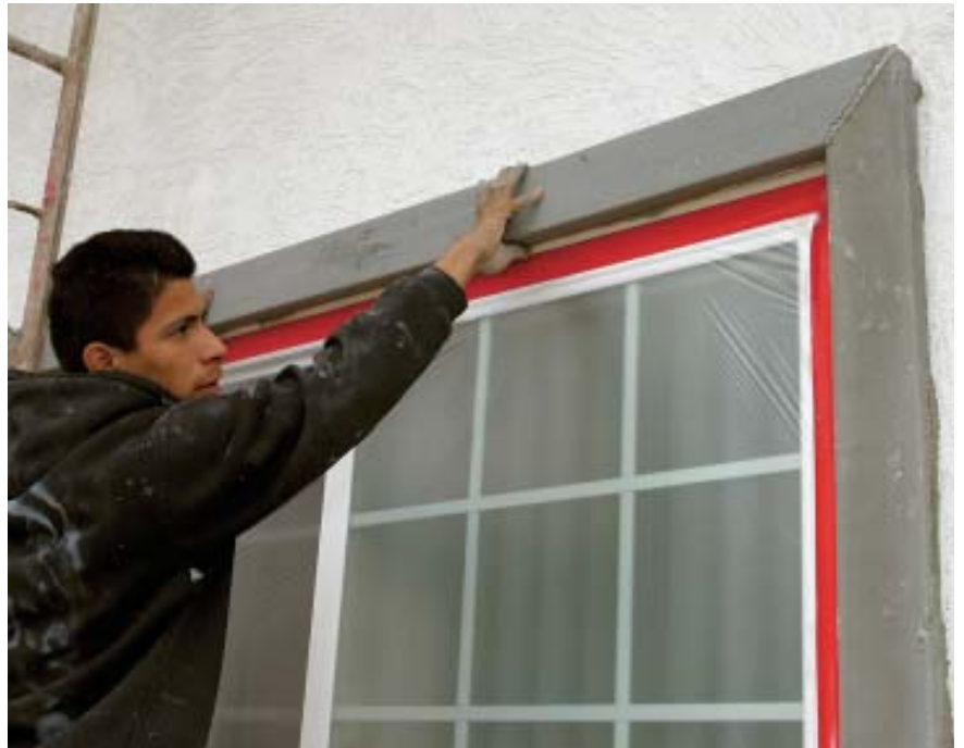
Figure 5. After cutting the precoated trim to length (top left), the plasterer applies Foam Tite to the back (top right) before pressing it onto the building (above).
