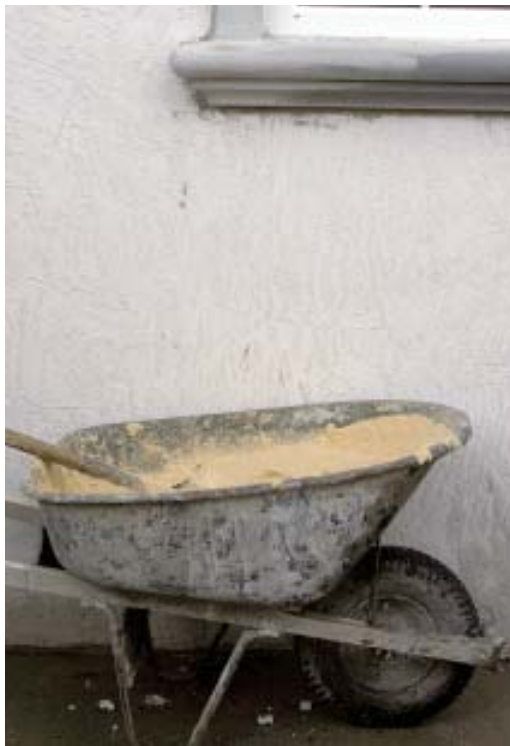
Figure 12. Each batch of the finish coat should be large enough to cover an entire section of wall. The wheelbarrow of colored material (left) will provide enough material to cover the uncoated wall to the left of the completed section in the photo below.
