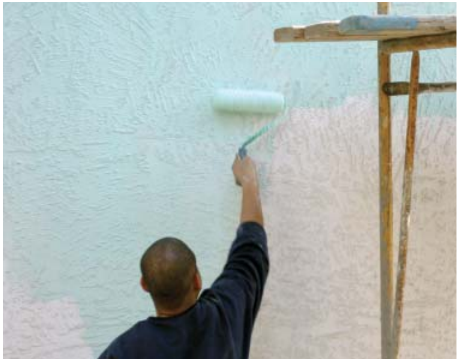
Figure 9. Painted stucco should be coated with a bonding agent before color coat is applied. This wall has never been painted, so bonding agent is not required, but the author’s crew applied it anyway as a “belt and suspenders” measure.
