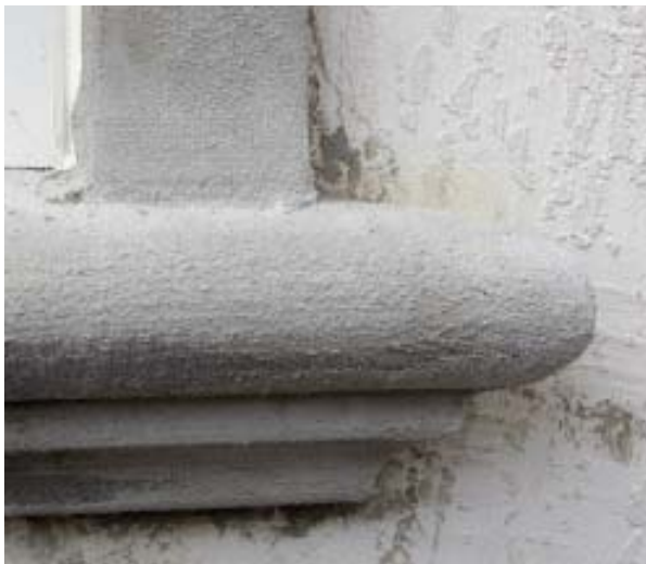
Figure 7. This sill and casing (right) have been glued to the wall and joined with mesh and Foam Tite. On this house, the trim will be the same color as the wall (below), but it could just as easily receive a different finish.
