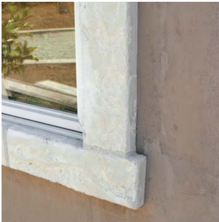
Figure 4. Though it looks like weathered stone, this casing is actually foam that was coated and textured in place. The faux limestone coating is much harder than color coat, so the trim is at least as impact-resistant as wood.
