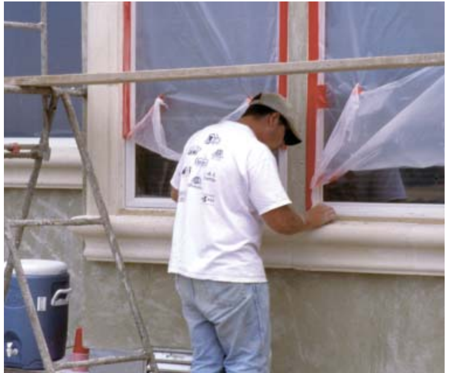
Figure 3. The author creates faux limestone in his shop by applying a polymer-concrete coating to foam profiles (left). His crew cuts the trim in the field, glues it to the building, and mortars the joints. When complete, it's hard to distinguish from real stone (below).
