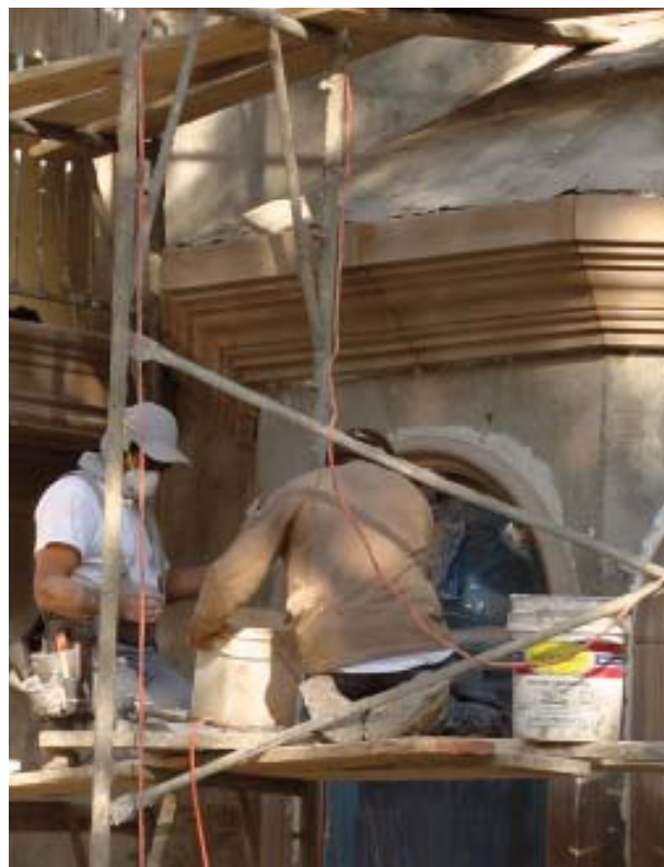
Figure 13. Cast-concrete trim is produced off site and delivered ready to install (above). It's very heavy, so it must be mechanically fastened to the wall; note the metal straps that extend from the edge of the pieces (right).
