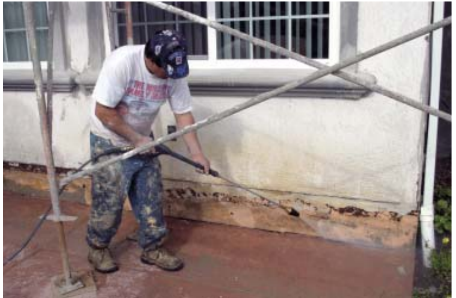
Figure 8. Color-coat stucco will readily adhere to an existing layer of the same material. This wall is being power-washed to remove dirt that would inhibit the bond.
