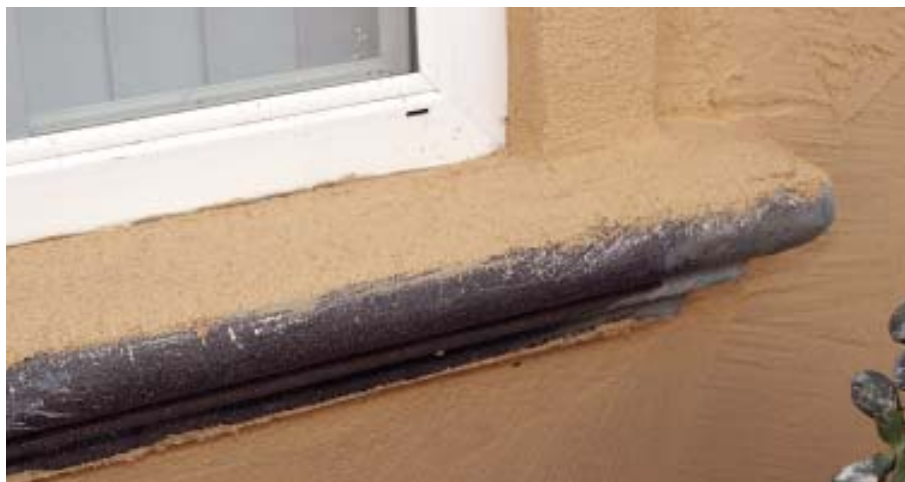
Figure 7. This sill and casing (right) have been glued to the wall and joined with mesh and Foam Tite. On this house, the trim will be the same color as the wall (below), but it could just as easily receive a different finish.
