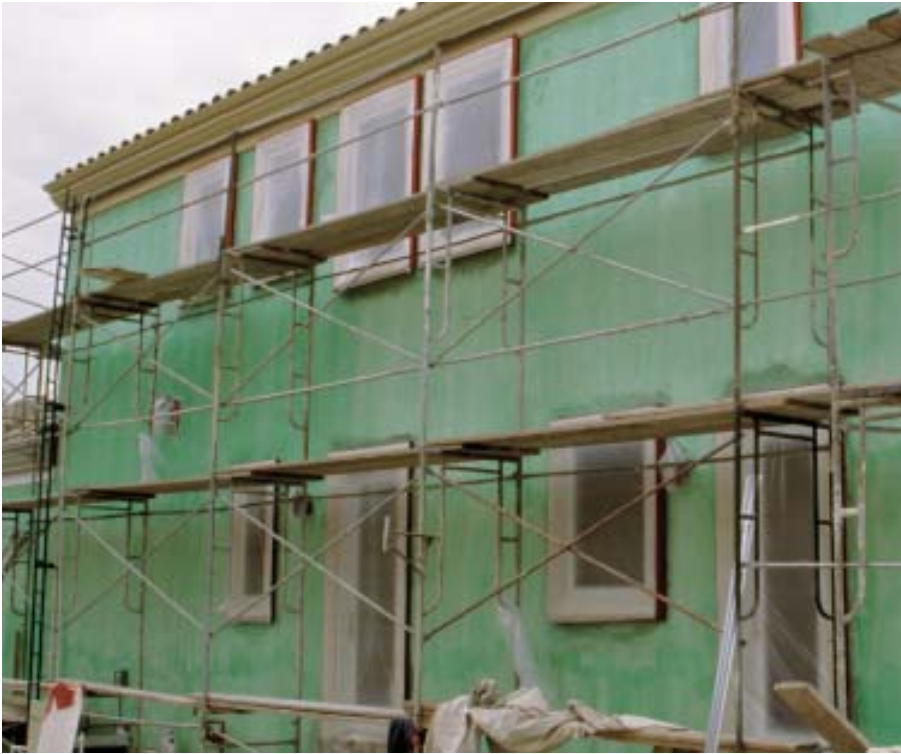
Figure 10. This wall was coated with a bonding agent to equalize the suction between the existing color coat and areas that were patched when the windows were replaced.
