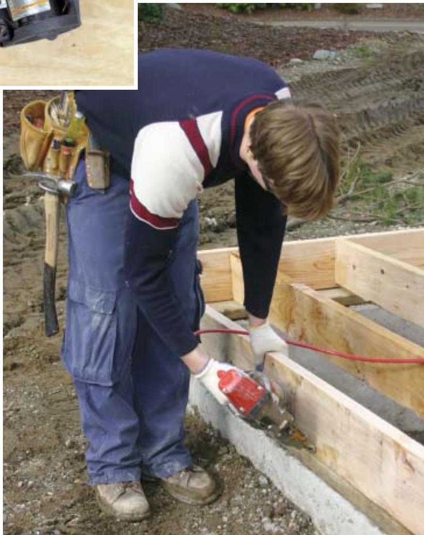
Most framers use coil guns only for sheathing, but Max's high-pressure framer is light enough for general nailing.
