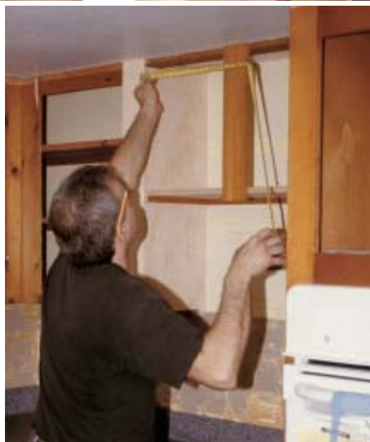
Figure 1. Despite showing their age, many older cabinets are well made, with solid plywood boxes and wood shelving well worth preserving. These are the ideal candidates for refacing.
