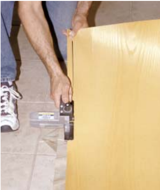
Figure 7. The authors purchase wood veneer in sheets backed with PSA (pressure-sensitive adhesive) and slice it on the job as needed. A hand-held laminate splitter speeds this work.
