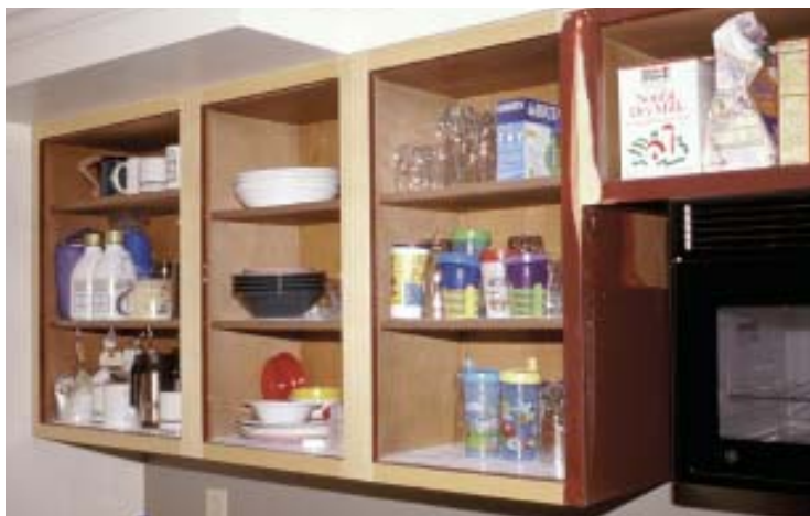
Figure 6. Face-frame irregularities between adjacent cabinets can be smoothed out by filling and sanding. The wood or plastic veneer then covers the original seams and creates the appearance of a single face frame.
