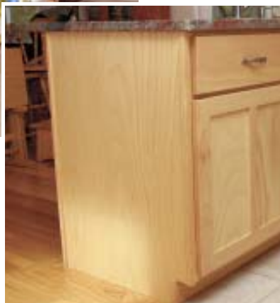
Figure 9. This exposed cabinet end (above) was covered with a 1/4-inch-thick prefinished plywood panel to match the face veneer. The stone countertop, installed first, includes an overhang allowance for the build-up.
