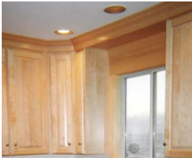
Figure 5. On this job, the original window valence (top left) was removed, exposing an unfinished exterior wall cavity (top right). Minor framing covered by a matching soffit panel and solid wood trim components tie the window in seamlessly with the new cabinet style.
