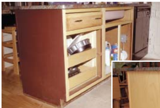
Figure 9. This exposed cabinet end (above) was covered with a 1/4-inch-thick prefinished plywood panel to match the face veneer. The stone countertop, installed first, includes an overhang allowance for the build-up.
