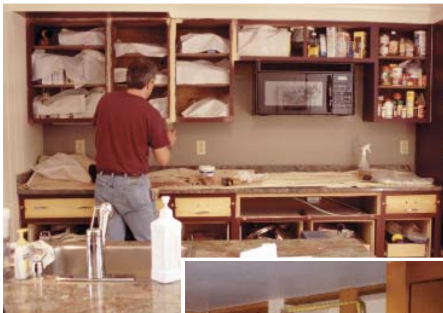
Figure 1. Despite showing their age, many older cabinets are well made, with solid plywood boxes and wood shelving well worth preserving. These are the ideal candidates for refacing.
