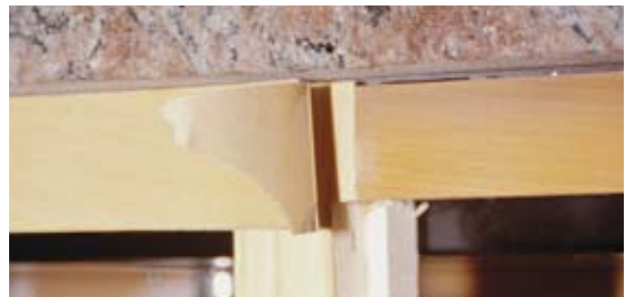
Figure 8. By leaving the tail end of the parting paper in place on the PSA-backed veneer, the installer can overlap intersecting facing strips, then cut them together to create a neat, tight-looking joint.
