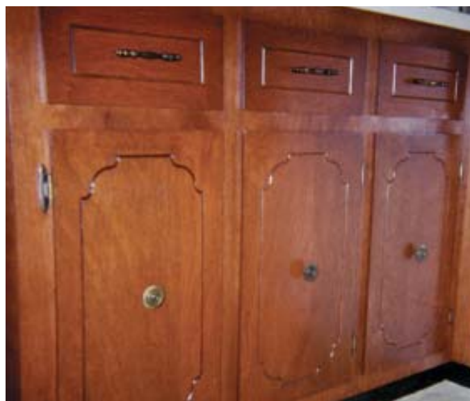
Figure 4. Wear and tear and water damage can all be reversed in a one-day tune-up process.
