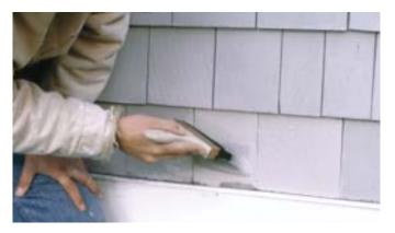
**New cold-weather paint formulas** can be used in temperatures as cold as 35°F. But their rapid drying in warm or hot weather may cause difficulties, and the finish color of touch-up work done in cool weather may vary from the color of walls painted in warmer weather using the same batch of paint.
