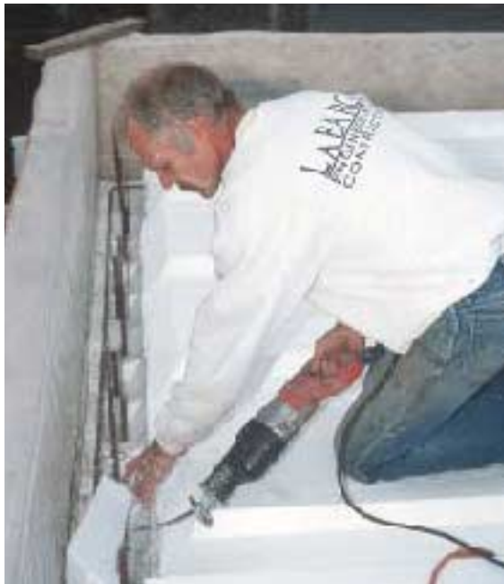
Figure 8. Form edges are eased to reduce the likelihood of a stress crack forming at the transition from horizontal to vertical concrete. The site supervisor approximated the panels' factory longitudinal bevel across the end cuts, using a reciprocating saw.
