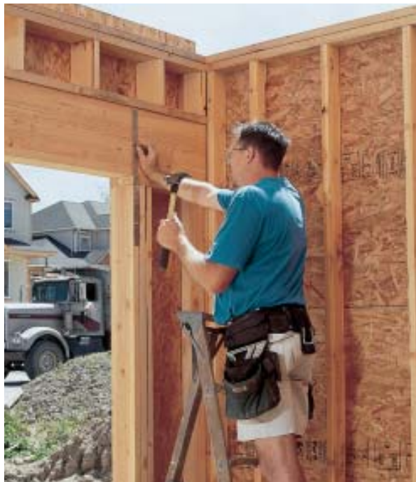
Figure 2. A 1,000-pound tension strap on the back side of the header prevents the header from rolling off the supports under load.
