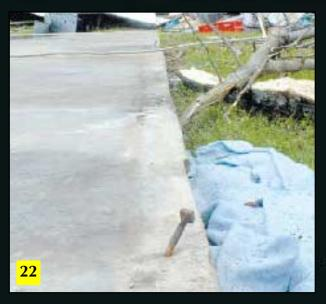
The anchor bolts in this slab-on-grade foundation were located 20 feet on-center and had no washers; none of the structure was left.
