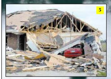
Nearly every home in the subdivision had a two-car garage (6). On about half the homes with major damage, the structural failure started with the garage. In some cases, weak garage doors were destroyed by wind and flying debris, exposing the interior of the homes to wind pressure. Inadequate wall bracing on either side of the garage opening and poor attachment between roofs, walls, and foundations also made garages vulnerable to internal pressurization.
