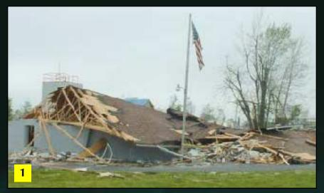
The masonry walls of this fire station (1) were inadequately reinforced to withstand the tornado forces. A lumber nailer bolted to the top of the walls supported open-web wood trusses that spanned 50 feet. Despite the enormous loads such large trusses could be subjected to in high winds, they were attached to the lumber plate with only toenails (2).
