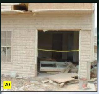
Here, in a home still under construction, a breach resulted because a pair of French doors were poorly fastened into the rough opening.
