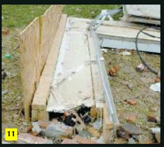
The return wall of this garage (10) was attached with only one anchor bolt. Though flat on the ground, the sheathed return wall was relatively intact, with the OSB sheathing still attached to the corner studs (11). Note the metal garage door track on the wall's inside face.
