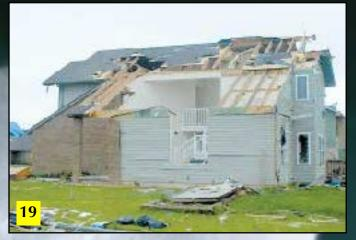
An initial breach at a large window resulted in internal pressurization and loss of the roof structure over the vaulted ceiling of this stairway. The rafters had been toenailed in place.
