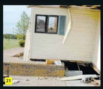
The hold-down anchors weren't adequate to keep this home from shifting 5 feet off its foundation.
