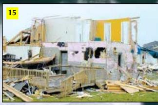
This plywood-sheathed house (1) fared much better than the home in the background (15), which was sheathed with non-structural rigid foam board. Rigid foam offers no racking resistance, and little resistance to damage from flying debris.
