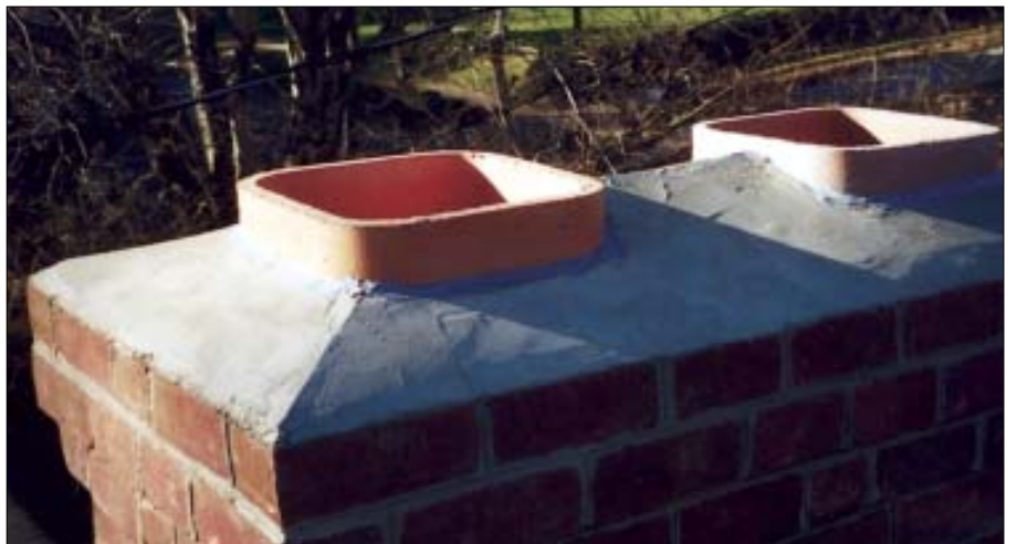
Figure 4. The completed cap rises sharply up to the flue liner and readily sheds rainwater.
