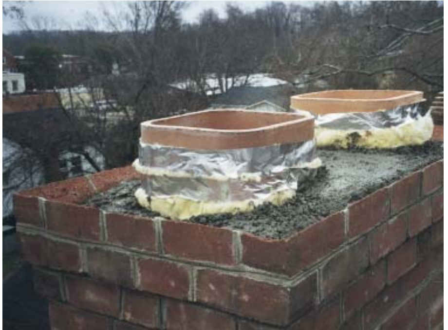
Figure 3. Wrapping the flue liner with fiberglass insulation isolates it from the cap.
