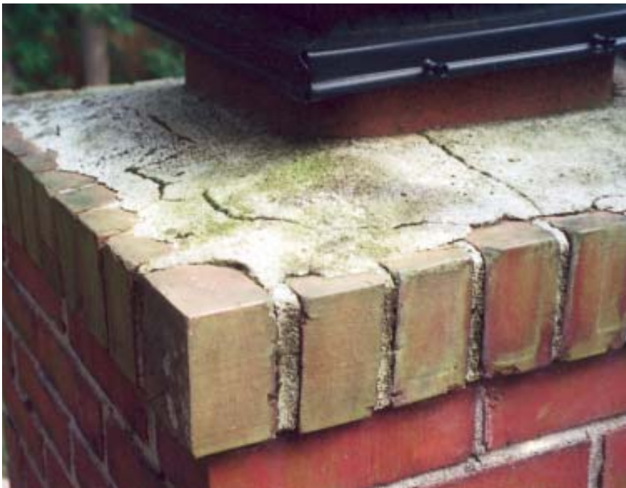
Figure 1. Weather has worn away the thin edge around the perimeter of this cap and numerous cracks have formed.
