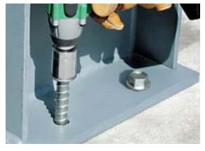
**Good Grip.** If you're looking for a strong connection to concrete, you might consider the *Titen HD* from Simpson. Available in <sup>3</sup>/8- and <sup>1</sup>/2-inch diameters from 1<sup>3</sup>/4 to 6 inches long, these heavy-duty anchors can provide over 8,000 pounds of shear strength and 12,000 pounds of tensile strength each, making them perfect for ledgers and other structural applications. You can tell the fastener's length without removing it by the code stamped on its head.
