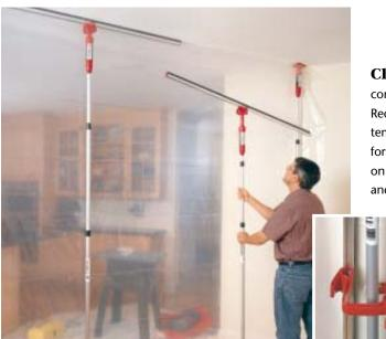
**Clean Room.** Legions of remodelers rely on the Zipwall dust containment system to protect their clients' home while they work. Recently, the company added two accessories to improve the system's dust-containment performance. The 5-foot *Foam Rail* conforms to textured ceilings or other surface irregularities and mounts on standard Zipwall poles. It holds the plastic tight to the ceiling and sets up fast. When the *Side Clamp* is combined with a Foam
