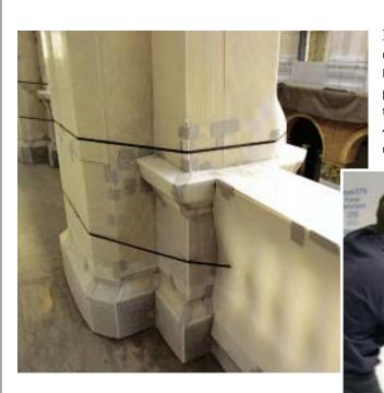
**Protective Plastic Panels.** Promising greater utility, lighter weight, and lower cost than plywood or Masonite, Cordek corrugated polypropylene is perfect for protecting surfaces, from flooring to windows. The translucent sheets won't absorb water or warp, and a 4x8-foot sheet weighs only about 2<sup>1</sup>/2 pounds. The product also folds easily and cuts with a utility knife, but the
