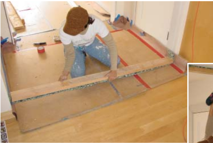
Figure 3. The top and bottom plates of temporary dust partitions are padded with strips of sill seal or carpet padding (left). Padded end studs are wedged between the plates to force the assembly tightly into the opening (below). Plates and studs are fastened together with drywall screws driven into predrilled holes (inset). The temporary wall is held in place by friction alone — no fasteners are used to secure the framing to the finished surfaces.
