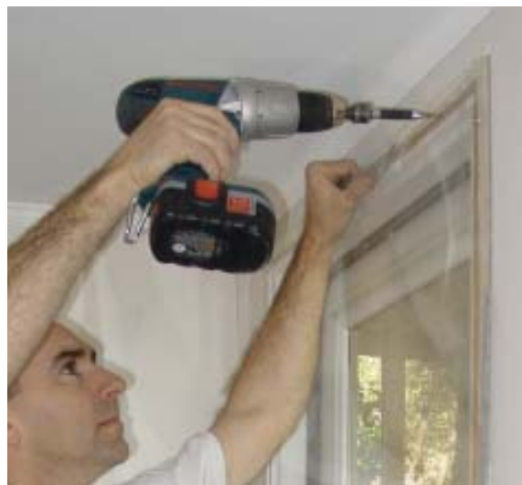
Figure 6. Protective sheets of 1/4-inch plexiglass are fastened to door or window jambs with screws driven through slightly oversized predrilled holes in the plexiglass.
