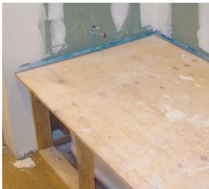
Figure 10. Two coats of Liquid Mask are brushed on to the perimeter of the tub (left), leaving a rubbery coating that prevents it from being scratched by the plywood cover. A plywood cover is duct-taped to the Liquid Mask (right).
