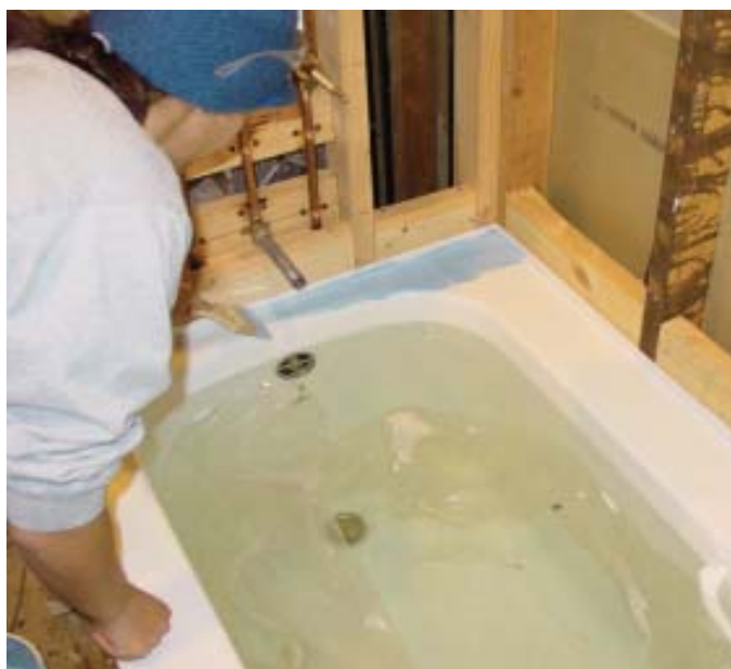
Figure 10. Two coats of Liquid Mask are brushed on to the perimeter of the tub (left), leaving a rubbery coating that prevents it from being scratched by the plywood cover. A plywood cover is duct-taped to the Liquid Mask (right).
