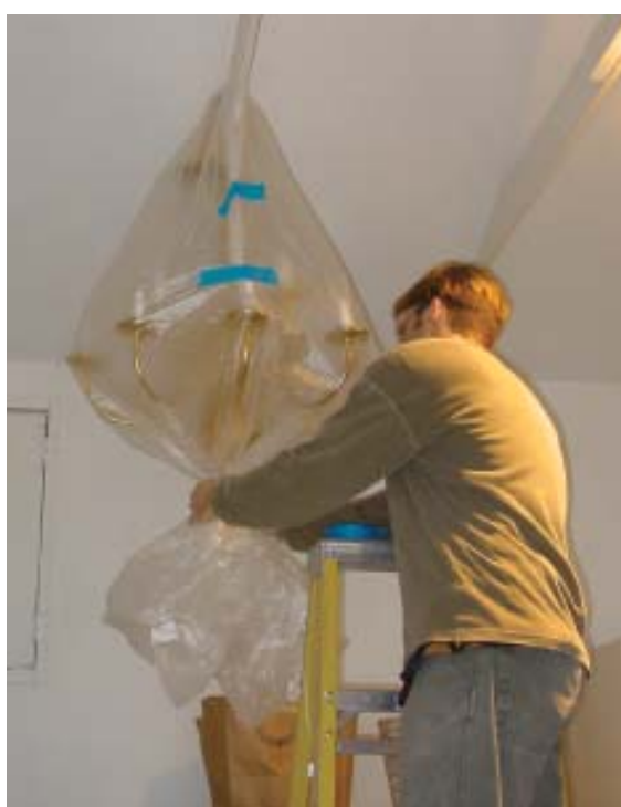
Figure 9. Fragile light fixtures are removed from the work area and hung from the garage framing to keep them out of harm's way. A sheet of plastic draped over the framing and fixture and fastened with tape keeps them free of dust.
