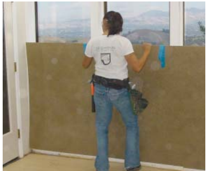
Figure 5. To protect low windows in areas where an existing floor will be demolished, the baseboards are removed and a series of screws are driven into the wall just below the height of the eventual replacement base (left). The windows are then covered with sheets of hardboard that rest on the screws at the bottom and are taped to the wall along their upper edges (right).
