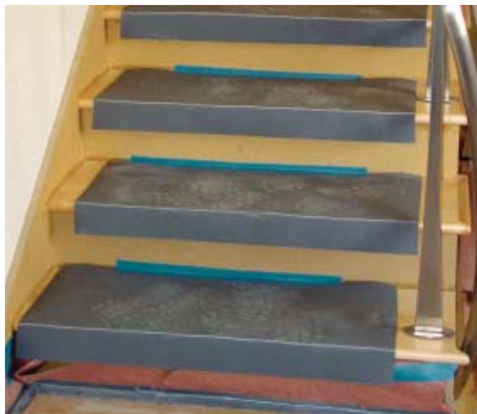
Figure 8. When protecting carpeted stairs with sticky roll plastic, it's important to cover the risers and full width of each tread, not just the portion that will get walked on (left). The landing above the steps will be covered with hardboard. The tread and nosing of hardwood stairs (right) are covered with Pro Tecta Top. The unprotected MDF risers will be painted later.
