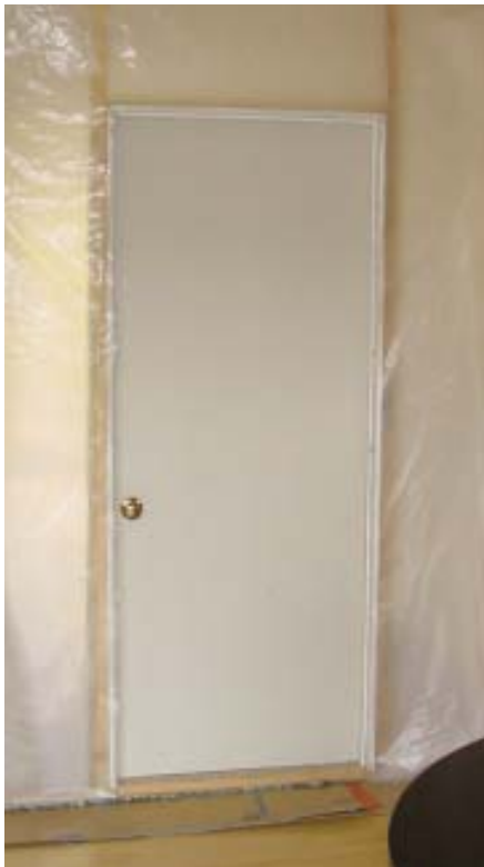
Figure 4. Stick-on zipper doors (top) aren't very durable, but they're inexpensive and easy to install, so the author uses them for lightly traveled passages. The cords taped to the poly above the zippered flap are used to tie the door in the open position. A weatherstripped hollow-core door (above) is a better choice for heavily used openings between living space and work area.
