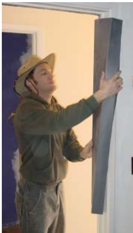
Figure 7. Proprietary jamb protectors wrap easily around openings and stay in place without fastenings.
