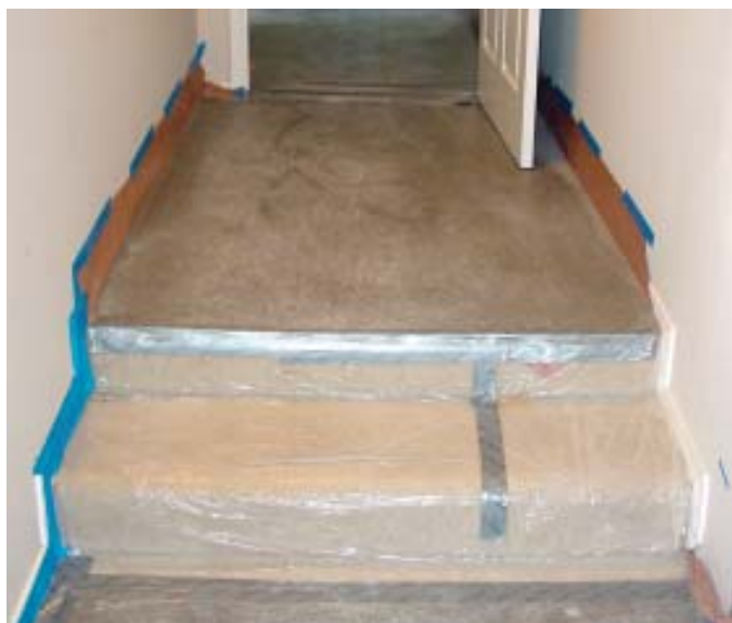
Figure 8. When protecting carpeted stairs with sticky roll plastic, it's important to cover the risers and full width of each tread, not just the portion that will get walked on (left). The landing above the steps will be covered with hardboard. The tread and nosing of hardwood stairs (right) are covered with Pro Tecta Top. The unprotected MDF risers will be painted later.
