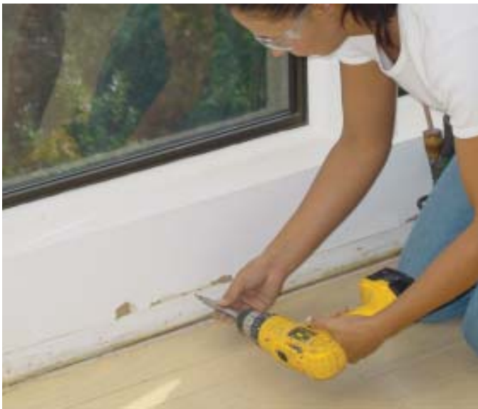
Figure 5. To protect low windows in areas where an existing floor will be demolished, the baseboards are removed and a series of screws are driven into the wall just below the height of the eventual replacement base (left). The windows are then covered with sheets of hardboard that rest on the screws at the bottom and are taped to the wall along their upper edges (right).
