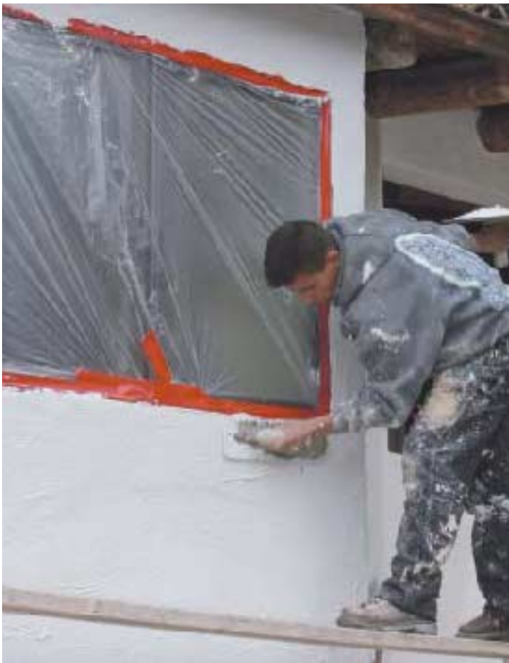
For the sand finish being applied here, the top coat is applied with a trowel (left) and feathered out with a sponge float (right), which brings the sand to the surface.
