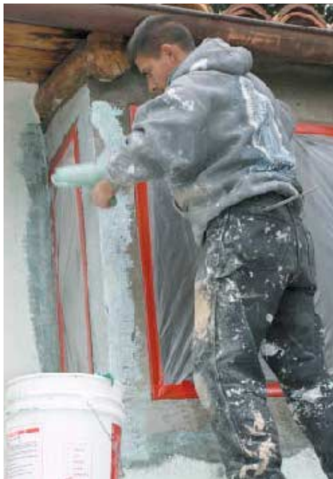
Above, the author trowels on Maxit 690, a premixed one-coat reinforced stucco that reduces the time it takes to make a patch. At right, a worker rolls on a bonding agent, which helps the stucco finish coat adhere to the painted surface of the existing stucco.
