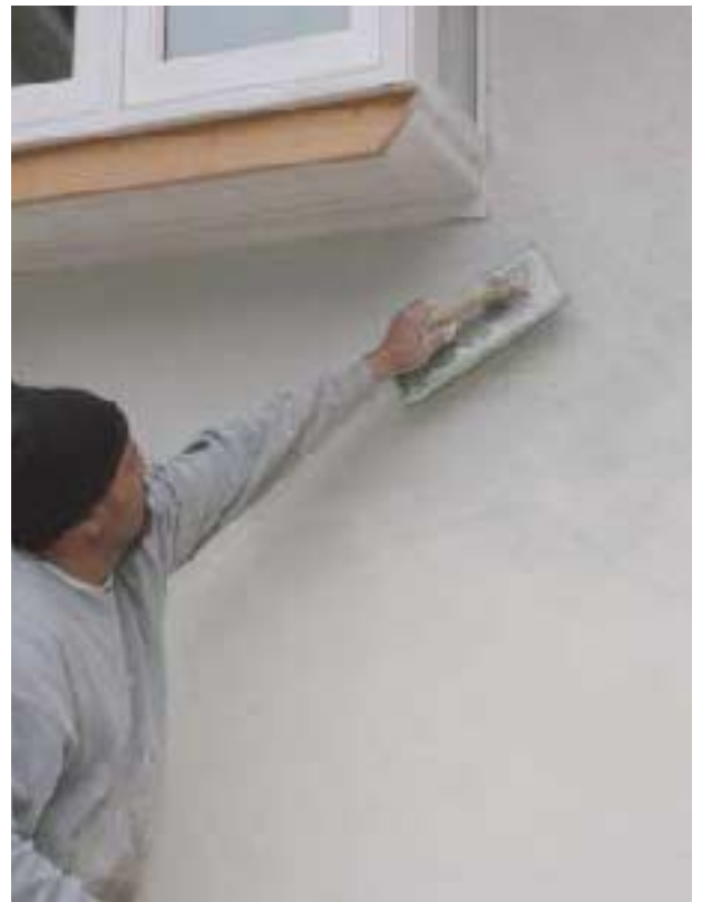
For the sand finish being applied here, the top coat is applied with a trowel (left) and feathered out with a sponge float (right), which brings the sand to the surface.
