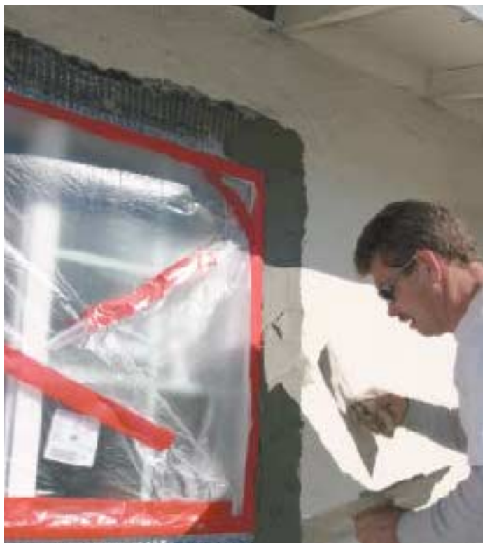
Above, the author trowels on Maxit 690, a premixed one-coat reinforced stucco that reduces the time it takes to make a patch. At right, a worker rolls on a bonding agent, which helps the stucco finish coat adhere to the painted surface of the existing stucco.
