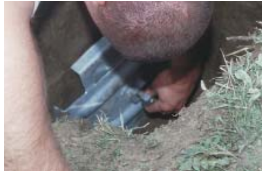
Figure 8. To bring the bulging wall back into line, the author uses a wall plate and an earth anchor connected by a threaded rod — the wall plate goes against the inside face of the wall; the earth anchor goes in a hole in the ground outside (below right). A hardened point screwed on to the end protects against thread damage as the rod is driven (left).
