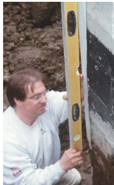
Figure 1. Soil pressure pushed this block foundation to the point of near collapse. Inside, the wall bows in a little more than 3 inches at the center, pushing the electrical panel with it. Note the sunken wall next to the garage door.
