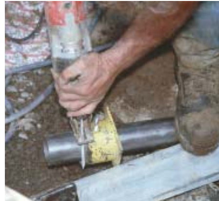
Figure 6. A reciprocating saw with a heavy-duty blade cuts the last section of pipe to length. A saw guide provided by the pier manufacturer ensures a square cut so there's no settling later. With the post cut to length, a steel insert is also cut to length using the same saw guide. The insert is slipped inside the top of the pier for additional reinforcement.
