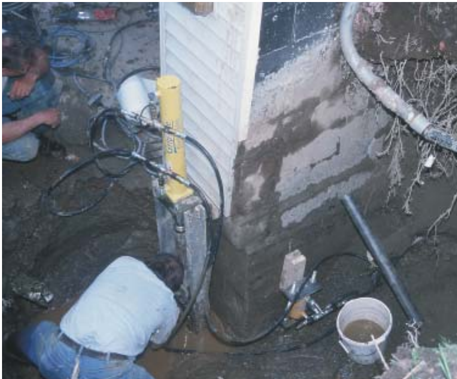
Figure 7. After both piers are in place, a second small hydraulic ram is attached to the hydraulic pump and attached to the first post (right). With both rams connected, pressure is applied to equalize the loading on the two posts (below). Once the bolts are tightened with a pair of adjustable wrenches, the hydraulic cylinders are removed (bottom right).
