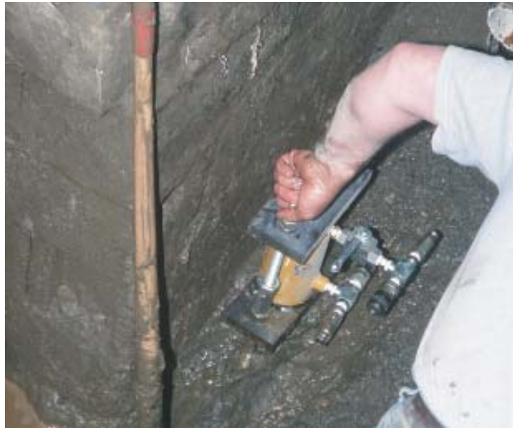
Figure 7. After both piers are in place, a second small hydraulic ram is attached to the hydraulic pump and attached to the first post (right). With both rams connected, pressure is applied to equalize the loading on the two posts (below). Once the bolts are tightened with a pair of adjustable wrenches, the hydraulic cylinders are removed (bottom right).
