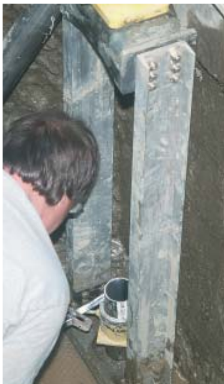
Figure 6. A reciprocating saw with a heavy-duty blade cuts the last section of pipe to length. A saw guide provided by the pier manufacturer ensures a square cut so there's no settling later. With the post cut to length, a steel insert is also cut to length using the same saw guide. The insert is slipped inside the top of the pier for additional reinforcement.
