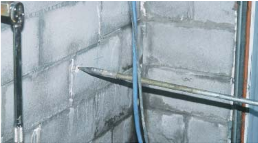
Figure 8. To bring the bulging wall back into line, the author uses a wall plate and an earth anchor connected by a threaded rod — the wall plate goes against the inside face of the wall; the earth anchor goes in a hole in the ground outside (below right). A hardened point screwed on to the end protects against thread damage as the rod is driven (left).
