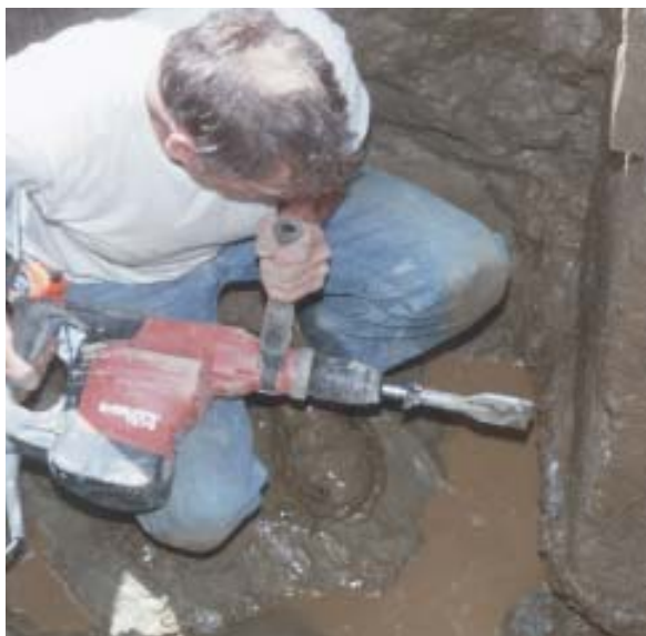
Figure 3. It's important that the footing rest squarely on the angled bracket; otherwise, the concrete could crack while it's lifted. Here, a rotary hammer with a 3-inch chisel is used to square up the sides and bottom of the footing. In extreme cases where one side of the footing is thicker than the other, steel shims are used to level the bottom.
