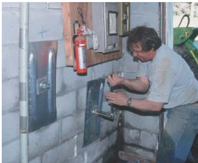
Figure 9. A plastic sleeve over the end of the rod (right) prevents the threads from catching on the block instead of transferring the force to the wall anchor. The three bolts are tightened incrementally with a torque wrench (below) to gradually move the wall back in line without breaking the block. After the bolts are tightened, the soil in the hole outside is compacted (bottom) to prevent water from collecting there and causing frost movement.
