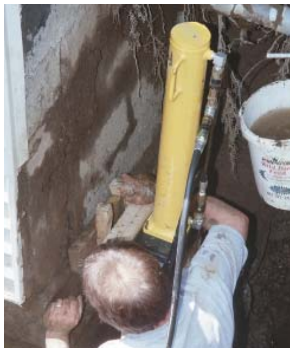
Figure 4. After the bracket and steel pipe are in place (top left and right), the author uses a magnetic angle finder to ensure that the hydraulic ram is pushing the pipe at the proper angle (above). Once everything is in the proper position, the ram is brought into the trench and hooked over the support bracket. Once again, the angle is checked and wood wedges and shims are placed between the house and the ram to ensure everything stays in the correct position (right).
