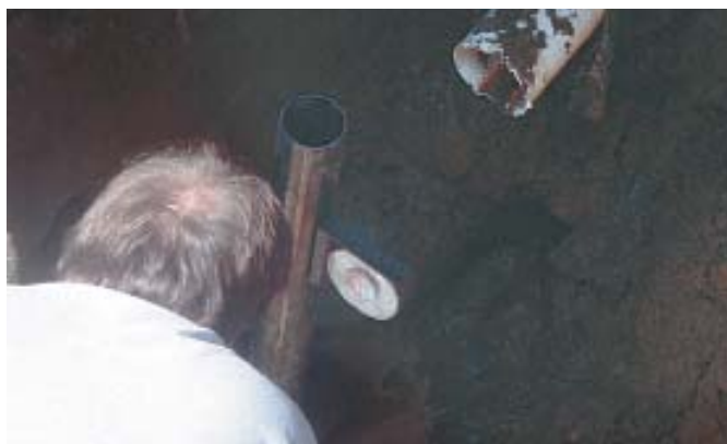
Figure 4. After the bracket and steel pipe are in place (top left and right), the author uses a magnetic angle finder to ensure that the hydraulic ram is pushing the pipe at the proper angle (above). Once everything is in the proper position, the ram is brought into the trench and hooked over the support bracket. Once again, the angle is checked and wood wedges and shims are placed between the house and the ram to ensure everything stays in the correct position (right).
