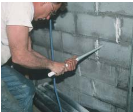
Figure 9. A plastic sleeve over the end of the rod (right) prevents the threads from catching on the block instead of transferring the force to the wall anchor. The three bolts are tightened incrementally with a torque wrench (below) to gradually move the wall back in line without breaking the block. After the bolts are tightened, the soil in the hole outside is compacted (bottom) to prevent water from collecting there and causing frost movement.
