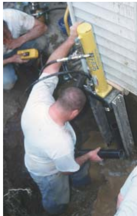
Figure 5. When the hydraulic ram bottoms out, it's retracted and a 15-inch section of pipe is inserted to finish driving the steel post. Driving a post all the way into the ground takes about five minutes. This particular project required four pipe sections per pier.
