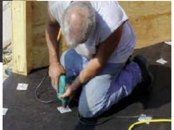
Figure 4. A roofer lays out the specified fasteners for the rigid-foam underlayment (left). After the screws are driven in (below), the EPDM is adhered to the deck (bottom).
