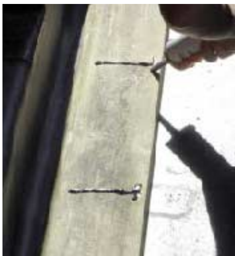
Figure 7. A heavy bead of sealant keeps water from getting behind the ledger (right). The crew also puts sealant on the back of the ledger (below) before screwing it into place. Depending on the loads, lag screws driven into predrilled, precaulked holes may be added for structural support.
