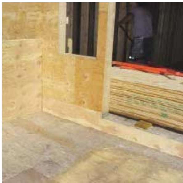
Figure 3. Half-height parapet walls framed on top of the sheathed roof (below) enclose most of the deck area, with just a small front panel left open (above). The front opening will receive a cedar railing and will be provided with roof-edge flashing, draining into a painted and copper-lined wood gutter.
