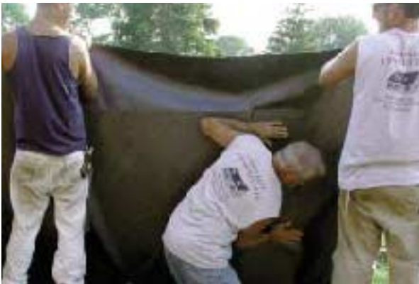
Figure 5. At right, the roofing contractor rolls adhesive onto the back of the EPDM in preparation for covering the parapet walls. Lapping and seaming the rubber into wall openings and at intersections and transitions creates a continuous watertight drainage plane capable of protecting vulnerable points in the building envelope against brutal oceanfront weather.
