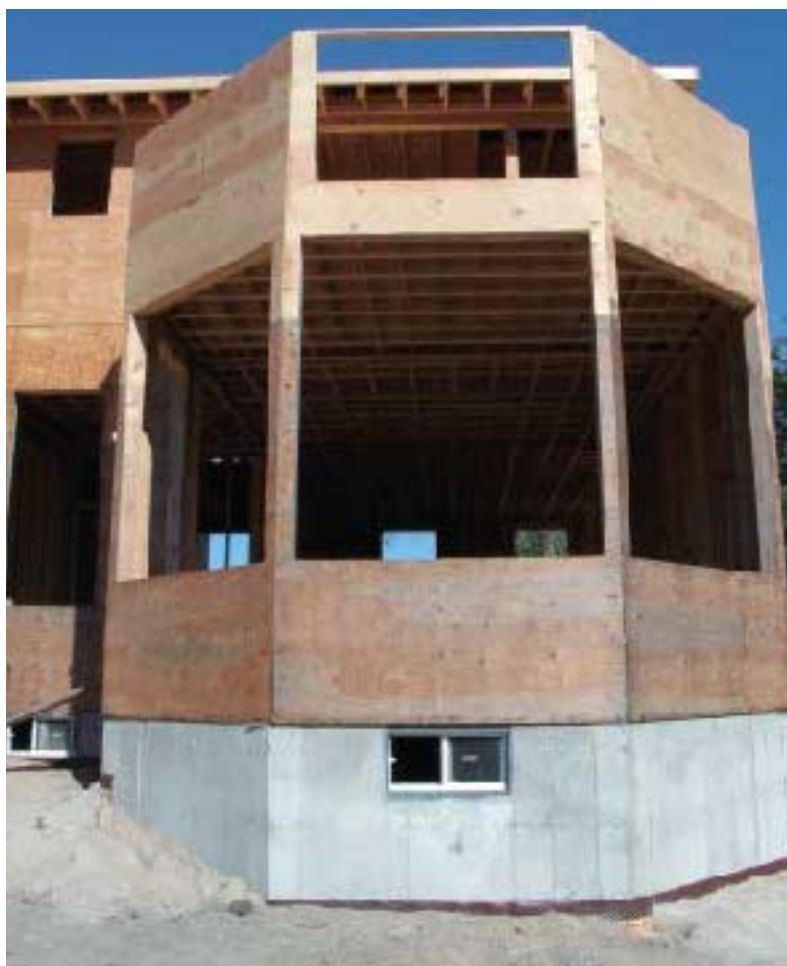
Figure 3. Half-height parapet walls framed on top of the sheathed roof (below) enclose most of the deck area, with just a small front panel left open (above). The front opening will receive a cedar railing and will be provided with roof-edge flashing, draining into a painted and copper-lined wood gutter.
