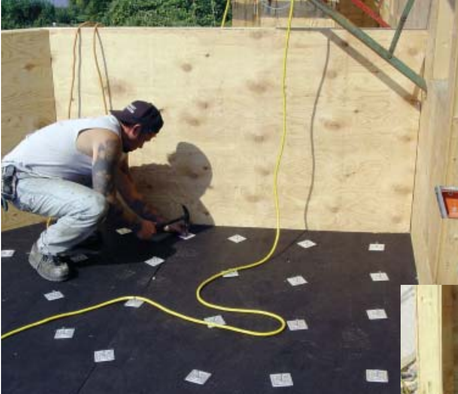
Figure 4. A roofer lays out the specified fasteners for the rigid-foam underlayment (left). After the screws are driven in (below), the EPDM is adhered to the deck (bottom).
