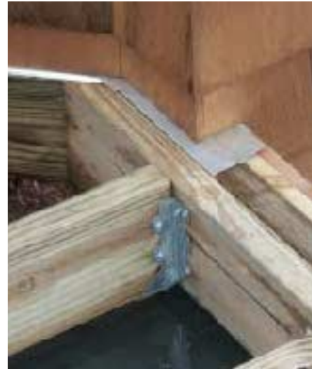
Figure 8. Deck joists are first screwed into place, with hangers added after.
