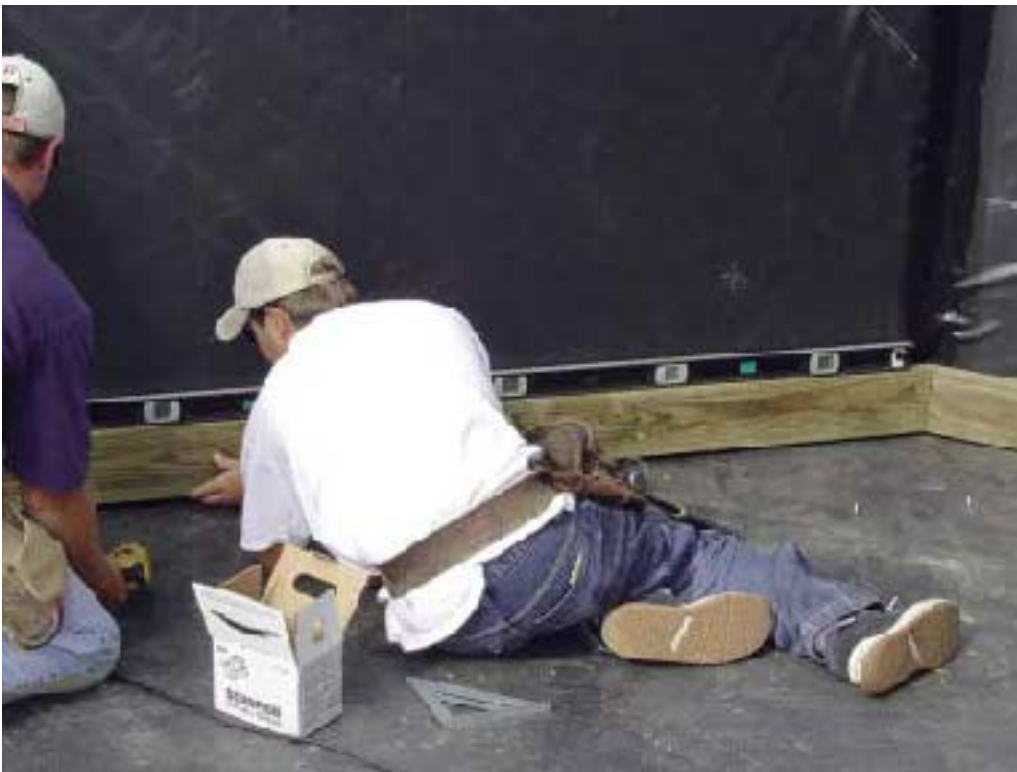
Figure 6. The crew first bevels the back of the ledger (below) to promote free drainage around the edges of the deck. Because the roof surface slopes, the ledger board has to be leveled — the drainage space gets wider toward the front of the roof.
