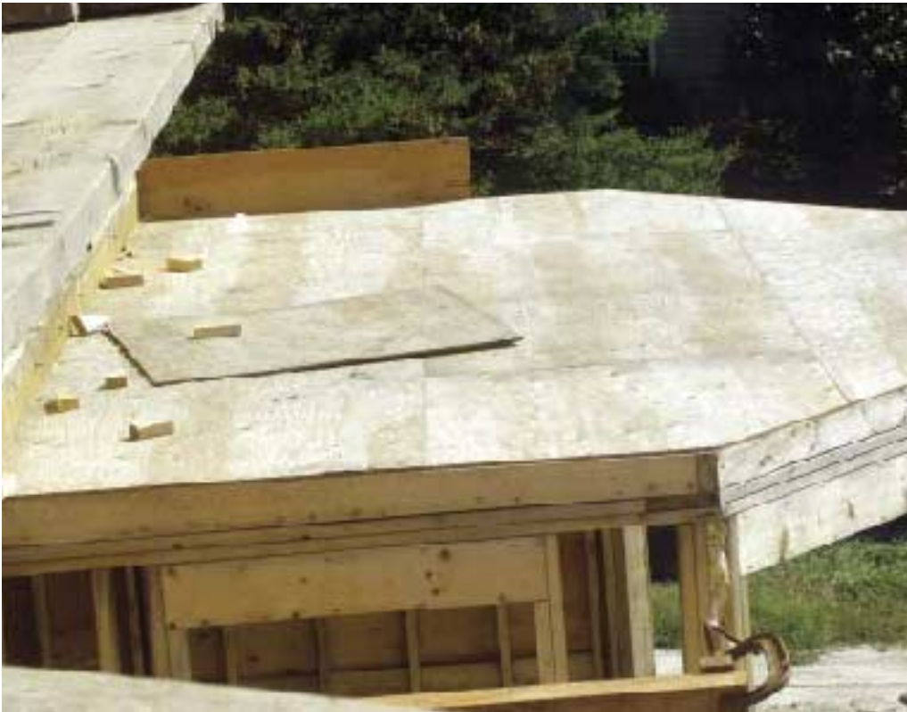
Figure 2. The ceiling joists of the room below the deck are ripped to provide a slight pitch away from the house, then sheathed with 1/2-inch plywood (left). Strapping helps ensure a flat drywall ceiling (below).
