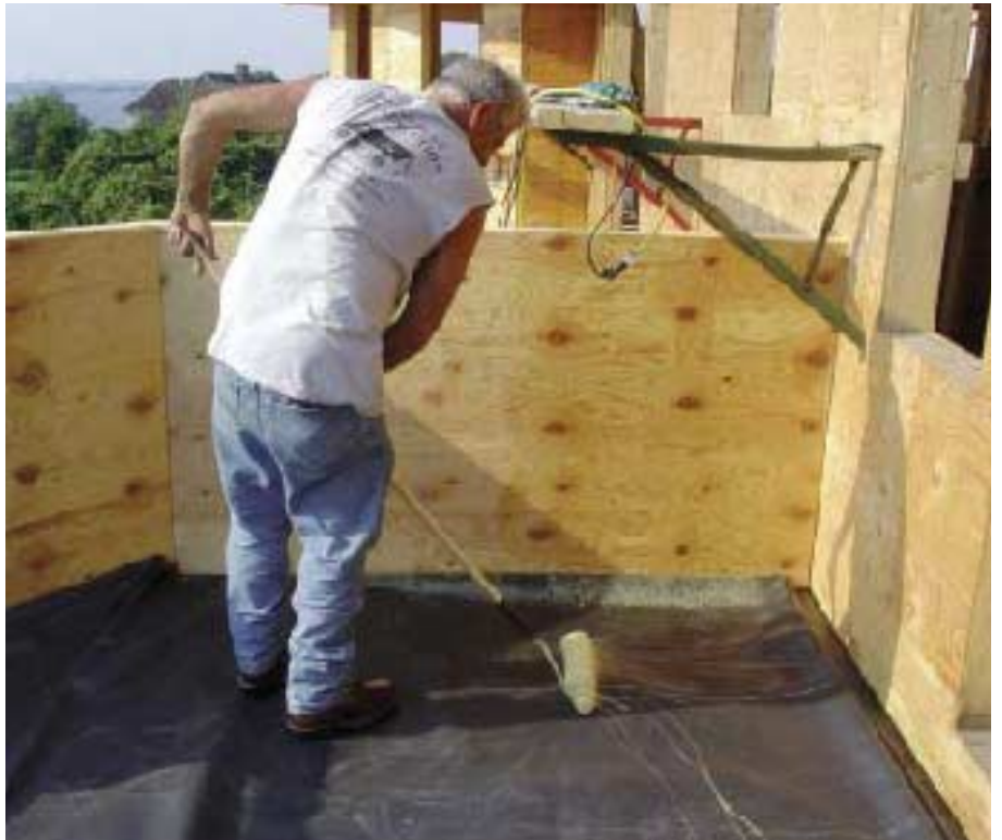
Figure 5. At right, the roofing contractor rolls adhesive onto the back of the EPDM in preparation for covering the parapet walls. Lapping and seaming the rubber into wall openings and at intersections and transitions creates a continuous watertight drainage plane capable of protecting vulnerable points in the building envelope against brutal oceanfront weather.
