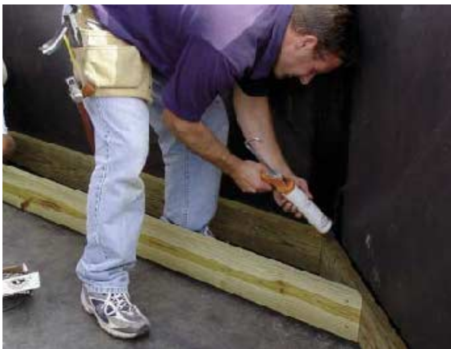
Figure 7. A heavy bead of sealant keeps water from getting behind the ledger (right). The crew also puts sealant on the back of the ledger (below) before screwing it into place. Depending on the loads, lag screws driven into predrilled, precaulked holes may be added for structural support.
