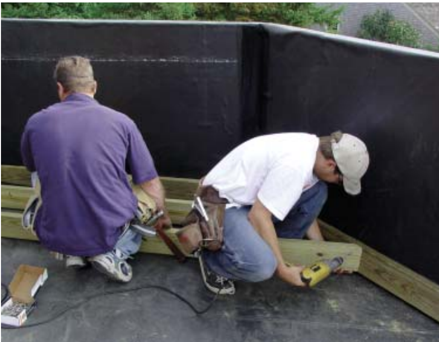
Figure 8. Deck joists are first screwed into place, with hangers added after.
