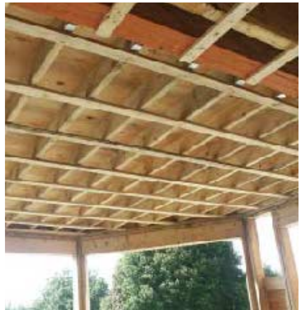
Figure 2. The ceiling joists of the room below the deck are ripped to provide a slight pitch away from the house, then sheathed with 1/2-inch plywood (left). Strapping helps ensure a flat drywall ceiling (below).
