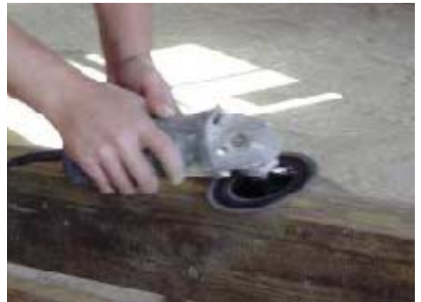
Figure 6. The crew first bevels the back of the ledger (below) to promote free drainage around the edges of the deck. Because the roof surface slopes, the ledger board has to be leveled — the drainage space gets wider toward the front of the roof.
