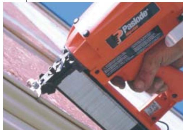
For foam insulation and other soft sheathing, the manufacturer includes a "handlebar" work element. The aluminum bar rides on the siding and provides a solid surface for depressing the contact foot.
