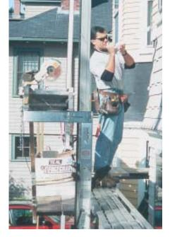
Working safely and efficiently two stories up requires plenty of room for workers, tools, and material. Alum-A-Pole's Pro-Bench provides a comfortable work table that doubles as a safety rail. The author added a small storage area below to hold a box or two of cedar shingles.
