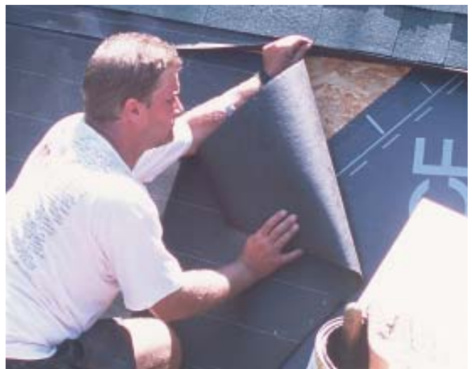
Figure 5. The roofing felt for each successive lift easily slips beneath the last course above, which is not stapled in the bottom 8 inches.
