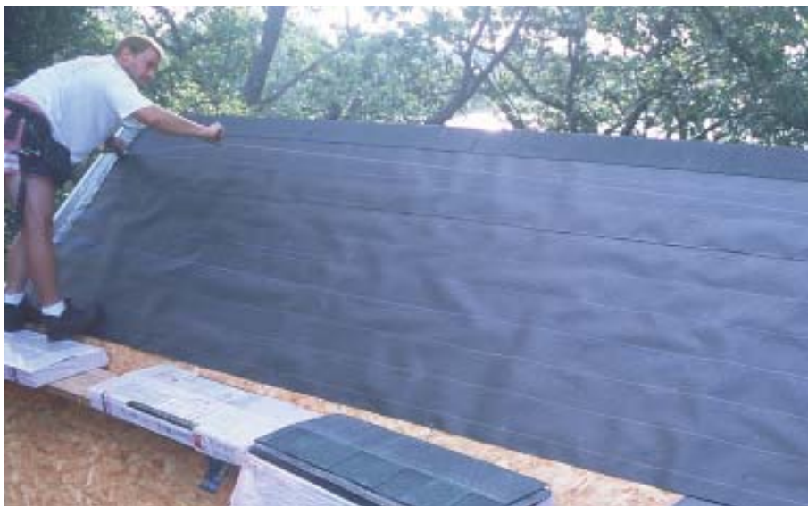
Figure 2. Working from a carefully placed starter shingle, a carpenter snaps control lines in 5-inch increments starting from the top of the roof.
