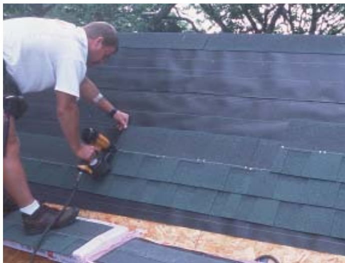
Figure 4. Once the lowest course in each lift is installed, the rest of the shingles in that lift follow.
