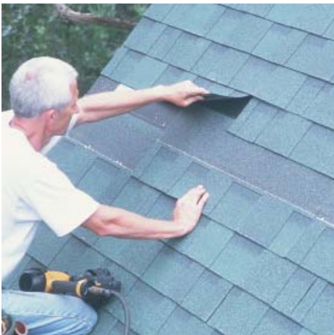
Figure 7. The next-to-last (left) and last (right) rows of each lift slide under the bottom course above. Finally, the bottom course gets permanently nailed off.
