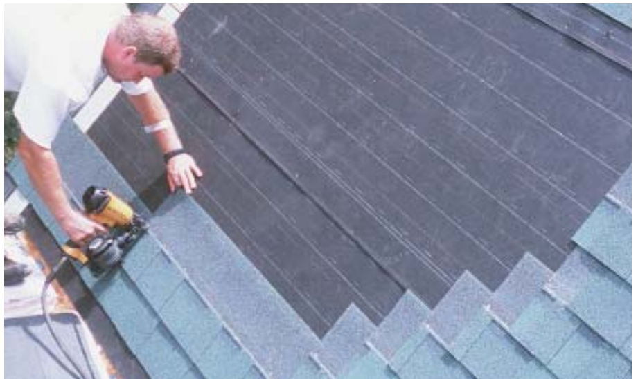
Figure 6. The process repeats itself down the roof. Control lines are snapped, and the bottom row gets nailed on the top corners only.
