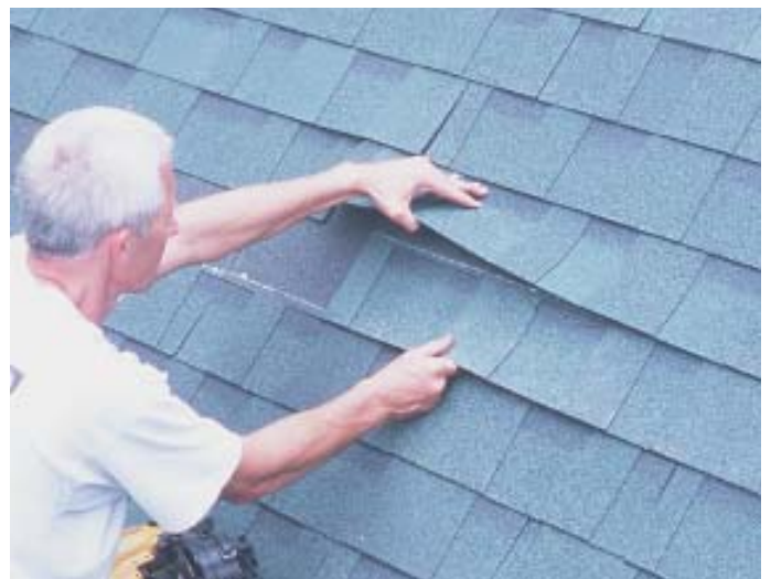
Figure 7. The next-to-last (left) and last (right) rows of each lift slide under the bottom course above. Finally, the bottom course gets permanently nailed off.
