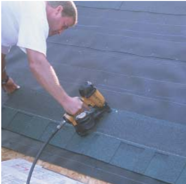
Figure 3. The first row of shingles in each lift gets nailed in the top corners only so shingles from the lift below can be slipped underneath later.
