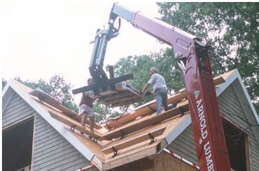
Figure 1. After staging is in place, shingles are boomed up and spread on the planks.
