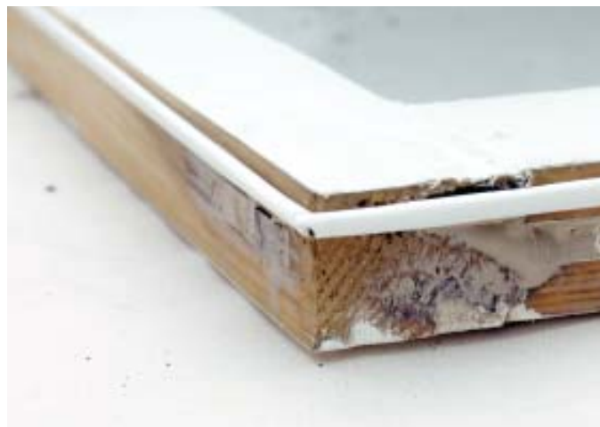
Figure 6. The pieces of weatherstrip are snipped to form mitered corners.
