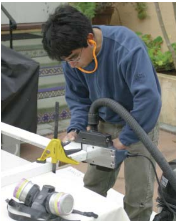
Figure 4. We used a power planer to refit the sash to the openings. The vacuum and dust collection hose captured nearly all of the chips.
