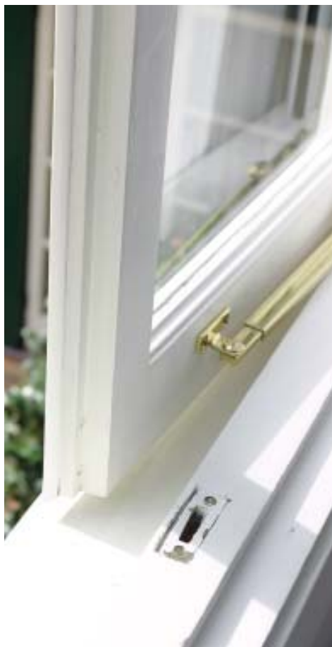
Figure 8. The new weatherstripping is unobtrusive but significantly cuts down on the amount of air and sound that comes through this window.
