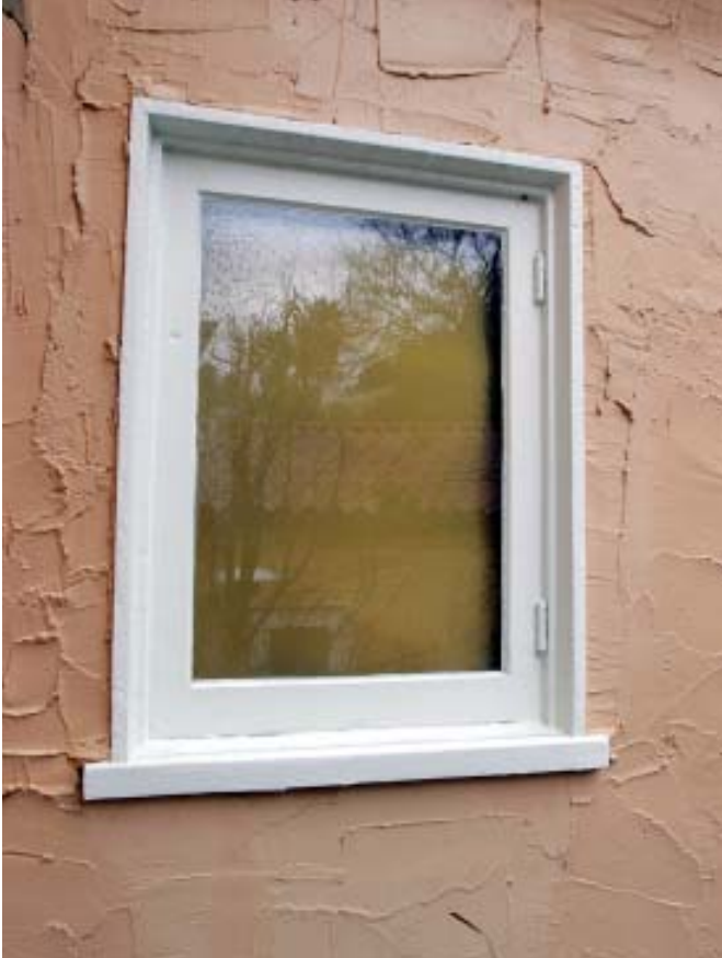
Figure 1. Replacing this window would require tearing out stucco, and it would be nearly impossible to blend a patch into such a highly textured surface.
