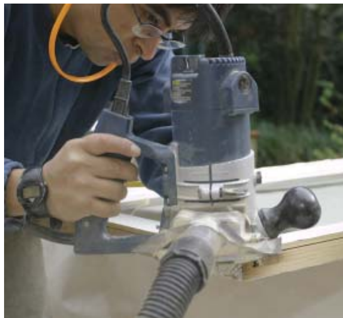
Figure 5. The slots for the weatherstripping were cut along the edge of the sash just in from the outside face.
