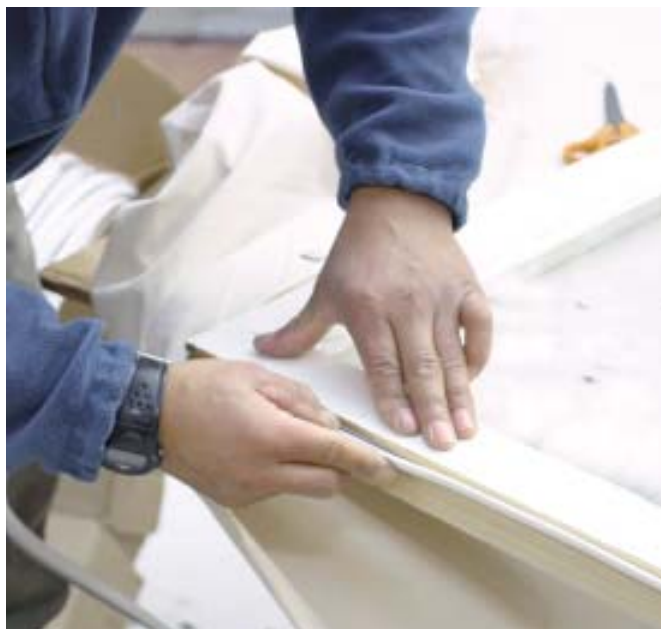
Figure 7. The weatherstrip is pressed into the kerf and held in place by barbs on the fin. This piece will be removed when it's time to paint the edge of the sash.
