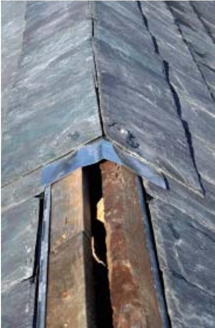
Figure 7. Rough-cut 1x4s nailed on top of the strapping at the ridge serve as backers for the ridge flashing and cap slates. The author uses Lexel sealant to seal the nail holes.
