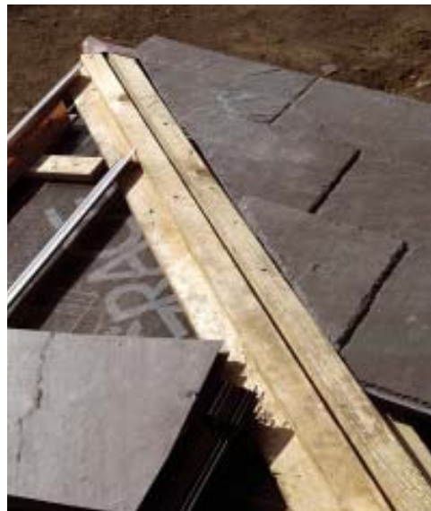
Figure 10. Like valley slates, hip slates are cut from full-size pieces. To provide support at the narrow edge of the triangular slate, the top of the link channels can be cut down to fit between the top batten and the wooden nailer that runs along the hip.
