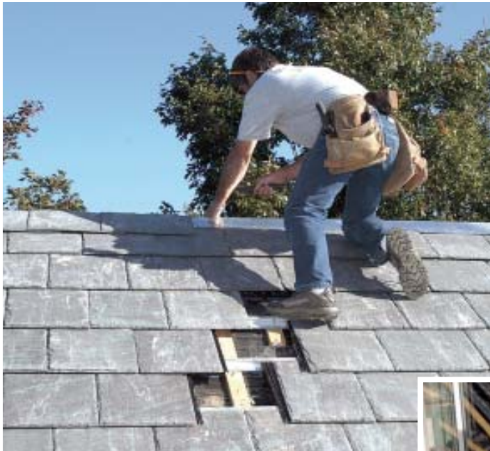
Figure 2. Because slates slip in and out easily on a Nu-lok roof, it's a simple matter to leave a “walking path” to access a work area (above). To remove a slate, you slip the support clip to one side (above right) and slide the slate out (right).
