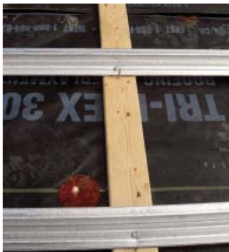
Figure 6. The metal battens are installed at 12 \frac{1}{8} inches on-center. To speed layout, the author's crew uses layout sticks drilled with holes, then drives small finish nails at every batten location. When final chalk lines are snapped from end to end of the roof, the nails serve as a cross-check that the overall layout is square and parallel to the eaves.
