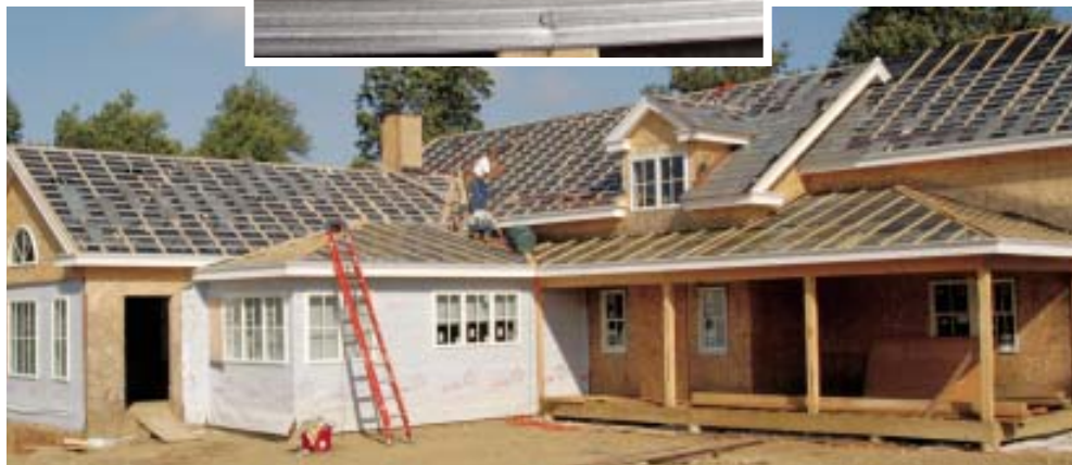
Figure 6. The metal battens are installed at 12 \frac{1}{8} inches on-center. To speed layout, the author's crew uses layout sticks drilled with holes, then drives small finish nails at every batten location. When final chalk lines are snapped from end to end of the roof, the nails serve as a cross-check that the overall layout is square and parallel to the eaves.
