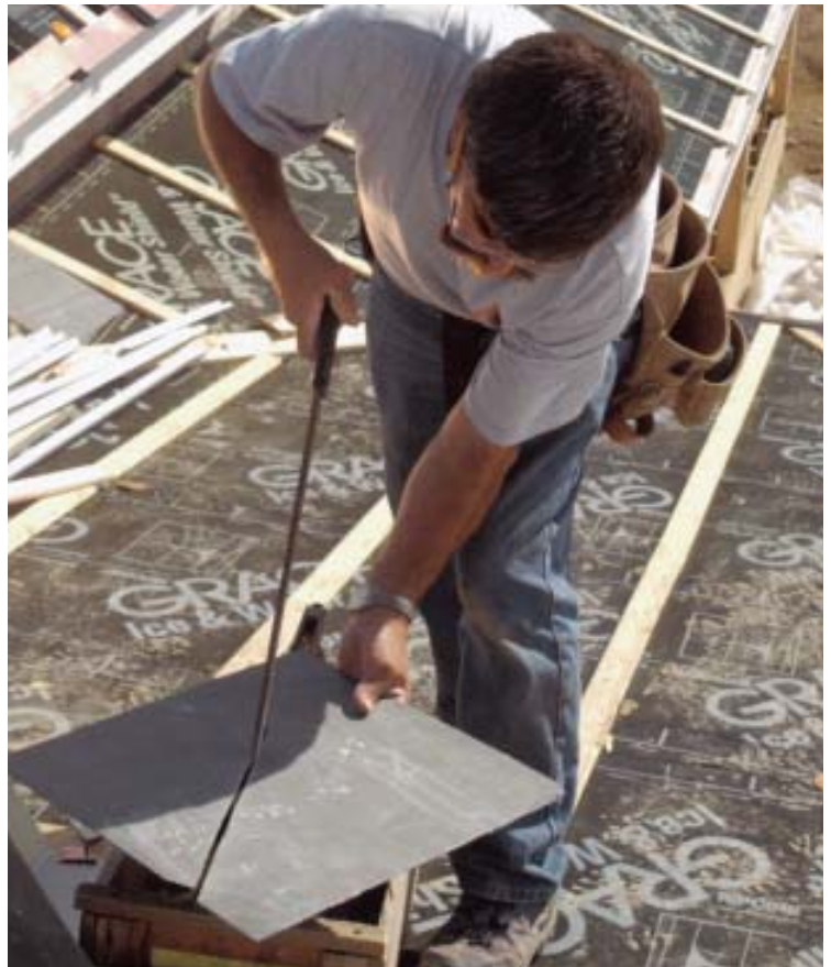
Figure 8. Using full-size 16-by-16-inch slates for the valleys gives maximum coverage without a lot of small triangular pieces.
