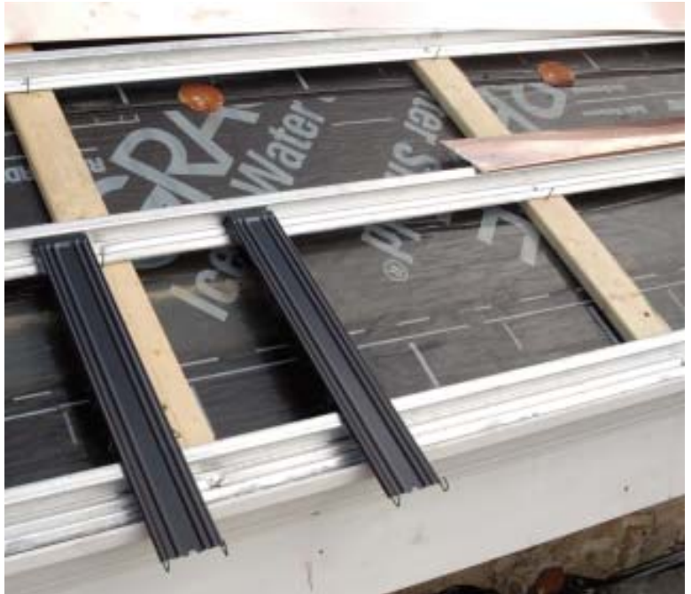
Figure 3. Horizontal galvalume battens support and retain the link channels that shed water between slates. Stainless clips, which spring-fit into the link channels, support the slate. According to a Nu-lok representative, the metal parts have been successfully tested for corrosion resistance in coastal environments.
