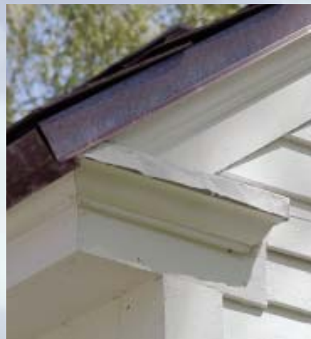
Figure 1. A Nu-lok slate roof looks virtually identical to a conventional slate roof. One slight difference is the extra height of the copper edge flashings (below). In the photo at bottom, the front building has a nearly completed Nu-lok roof; the two buildings in the background have traditional slate roofs.
