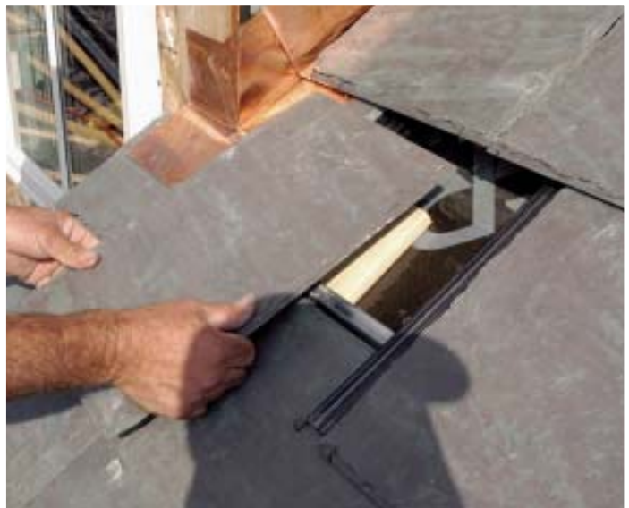
Figure 2. Because slates slip in and out easily on a Nu-lok roof, it's a simple matter to leave a “walking path” to access a work area (above). To remove a slate, you slip the support clip to one side (above right) and slide the slate out (right).
