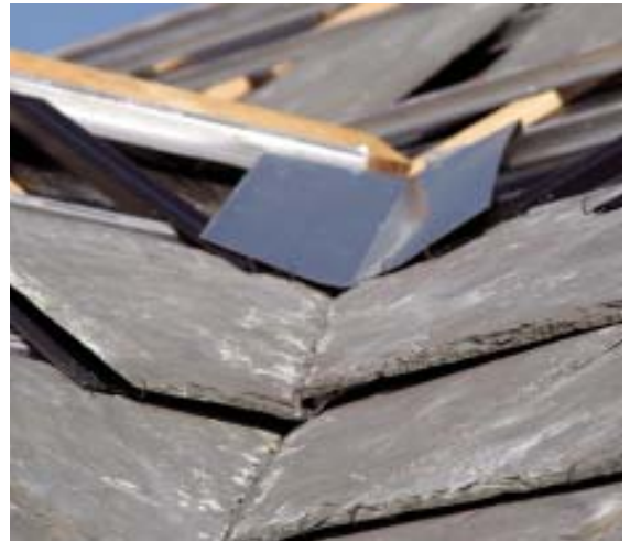
Figure 9. Galvanized steel counter flashings supported by the slate clips supply extra water protection at the valleys. The metal is cut with hand shears to match the horizontal course lines.
