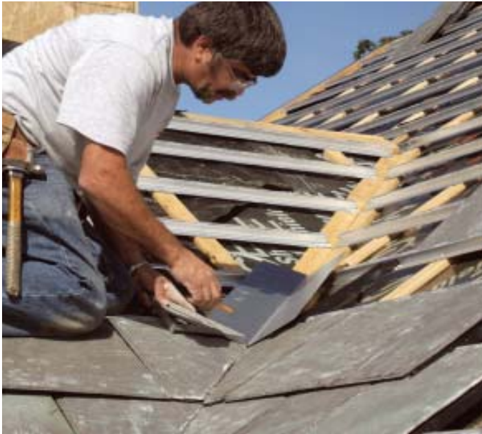
Figure 9. Galvanized steel counter flashings supported by the slate clips supply extra water protection at the valleys. The metal is cut with hand shears to match the horizontal course lines.
