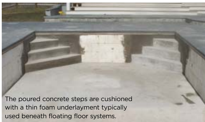
ICFs form the pool's walls and provide a resilient layer beneath the vinyl liner.
