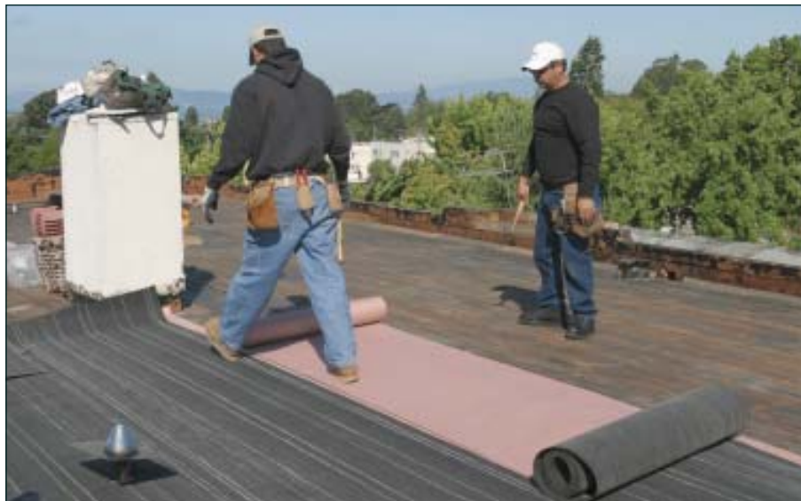
Figure 3. The base sheet goes over rosin paper and has 2-inch laps.
