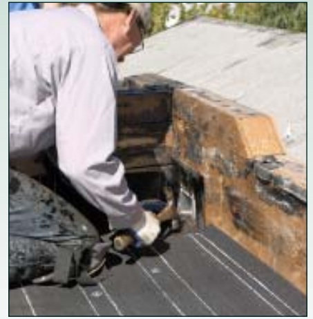
Figure 4. A roofer beds a scupper flashing in roofing cement (left) before fastening it over the base sheet (right).
