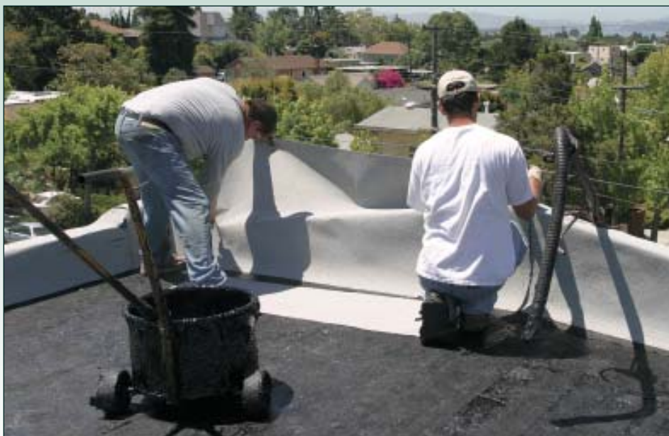
Figure 14. Loose aggregate will not stick to vertical surfaces, so the crew covers parapets with cap-sheet material. The roofers mopped hot asphalt onto the back of the sheet and are flipping it into position.
