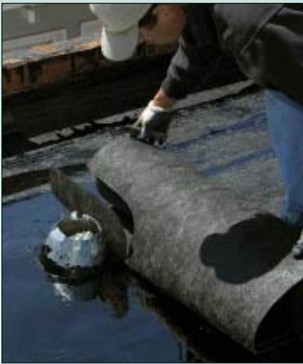
Figure 12. It's possible to flash penetrations after the bulk of the roof is done, but this roofer is laying the roof over the flashings, an approach that creates fewer seams.
