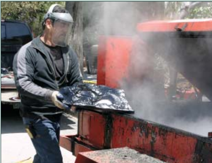
Figure 7. A roofer carefully slips another chunk of asphalt into the kettle. Splashed asphalt can cause serious burns, which is why he is wearing gloves, long sleeves, and face protection.
