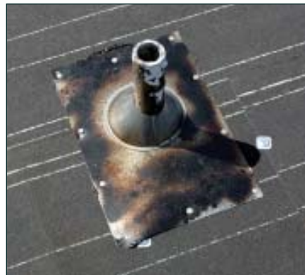
Figure 5. Flashings are primed to make the hot asphalt stick better. Note the caps under the nails that hold the base sheet to the roof.
