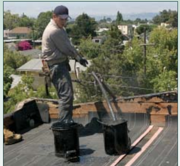
Figure 8. On small jobs, the hot asphalt is carried to the roof in buckets. This job was large enough that it made sense to pump the asphalt up in temporary pipes before transferring it to buckets or wheeled carts.
