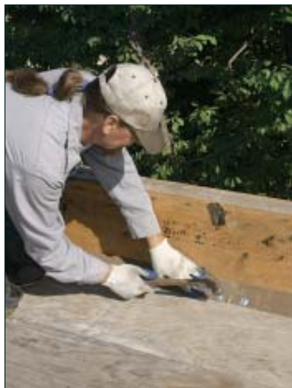
Figure 2. Fiberglass felts will not take tight bends, so the crew installs cant strips at inside corners.
