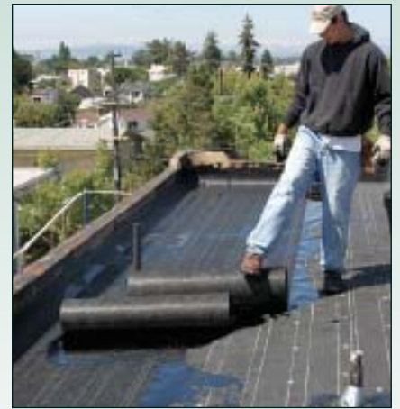
Figure 11. The roofers apply successive layers of felt over hot asphalt. On this roof, full sheets lap \frac{2}{3} onto the sheets below, which means there will be at least three layers of felt plus one layer of base sheet at any given point.
