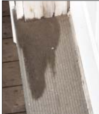
FIGURE 7. Doors and hardware take a beating on the beach. A steel door shows rust (below) and its pine jamb has deteriorated (near right), while a hardware-store storm-door closer is rusting badly (far right). Standard brass door hardware is tarnished and pitted (bottom center and right). For beach construction, the author recommends ordering special hardware designed for extreme exposures.
