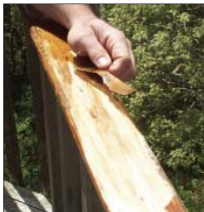
FIGURE 6. Periodic cleaning and re-staining is the only finish solution for these deck railings and parapet caps: Although the bare wood holds up, no film-forming clear finish can last long under coastal weather conditions.
