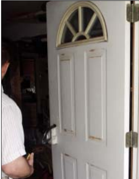
FIGURE 7. Doors and hardware take a beating on the beach. A steel door shows rust (below) and its pine jamb has deteriorated (near right), while a hardware-store storm-door closer is rusting badly (far right). Standard brass door hardware is tarnished and pitted (bottom center and right). For beach construction, the author recommends ordering special hardware designed for extreme exposures.
