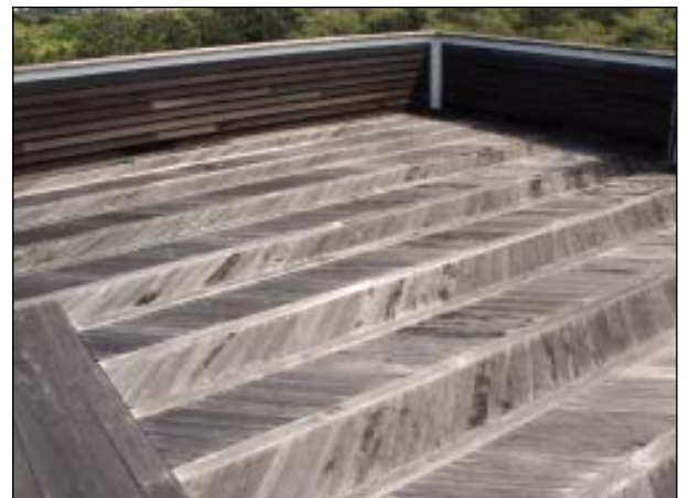
FIGURE 4. Naturally rot-resistant cedar rails (above) and mahogany decking (right) have performed well, but the author notes mahogany can be inconsistent, depending on the variety and on the presence of sapwood rather than heartwood boards in the shipment.
