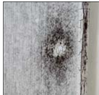
FIGURE 5. The author has gotten good performance from Cabot oil-based primer and acrylic solid stain (far left, above). In a few places, staining from galvanized nails has bled through (middle and right, above), and the underside of one clogged Douglas fir gutter has lost its paint (left).
