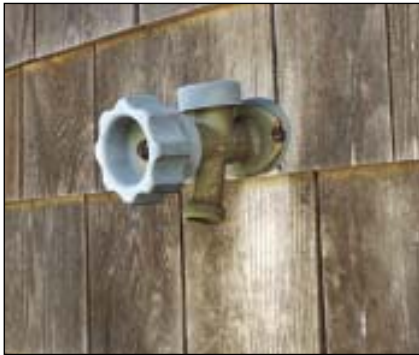
FIGURE 8. Recessed lighting fixtures tough enough for the beach are scarce, so the author uses “remodeling” fixtures that are easily replaced (top left). Replacement may also be the only option for this rusting vent cap (top right) or for rusting screws on a hose bibb (above). Galvanized caps terminating metal-and-asbestos fireplace vents have also rusted (right), but a stainless-steel boiler-vent cap is in good shape.
