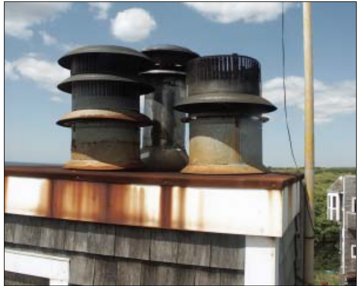
FIGURE 8. Recessed lighting fixtures tough enough for the beach are scarce, so the author uses “remodeling” fixtures that are easily replaced (top left). Replacement may also be the only option for this rusting vent cap (top right) or for rusting screws on a hose bibb (above). Galvanized caps terminating metal-and-asbestos fireplace vents have also rusted (right), but a stainless-steel boiler-vent cap is in good shape.
