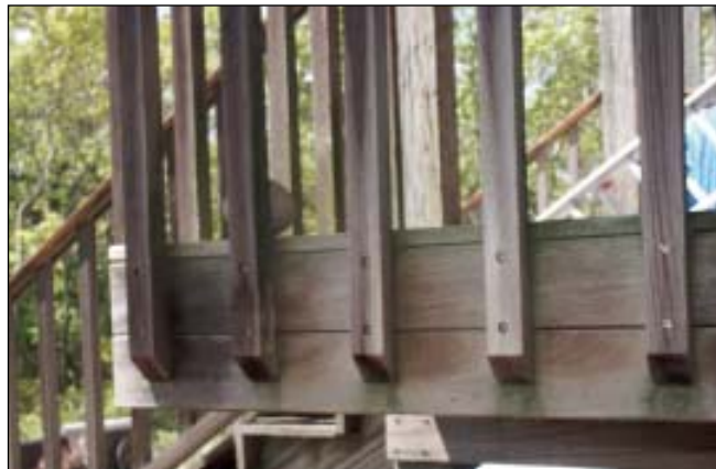
FIGURE 4. Naturally rot-resistant cedar rails (above) and mahogany decking (right) have performed well, but the author notes mahogany can be inconsistent, depending on the variety and on the presence of sapwood rather than heartwood boards in the shipment.
