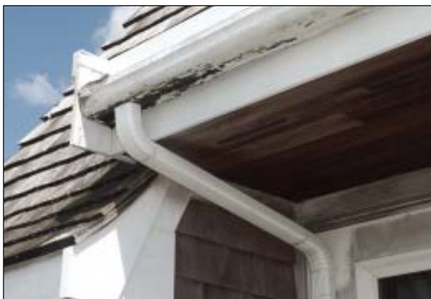
FIGURE 5. The author has gotten good performance from Cabot oil-based primer and acrylic solid stain (far left, above). In a few places, staining from galvanized nails has bled through (middle and right, above), and the underside of one clogged Douglas fir gutter has lost its paint (left).
