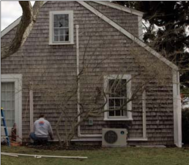
Outdoor condenser units can handle up to three zones. Although a mini-split system saves the expense of installing ductwork, the channels carrying the refrigerant lines and condensate drains are quite conspicuous.
