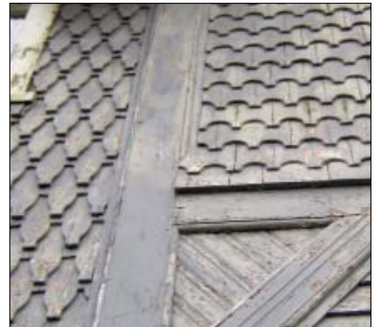
FIGURE 1. A striking example of the decorative use of pattern shingles is seen at Idlemoor — a home constructed on Nantucket Island in 1884. Most of original sidewall material (above) remains intact today.
