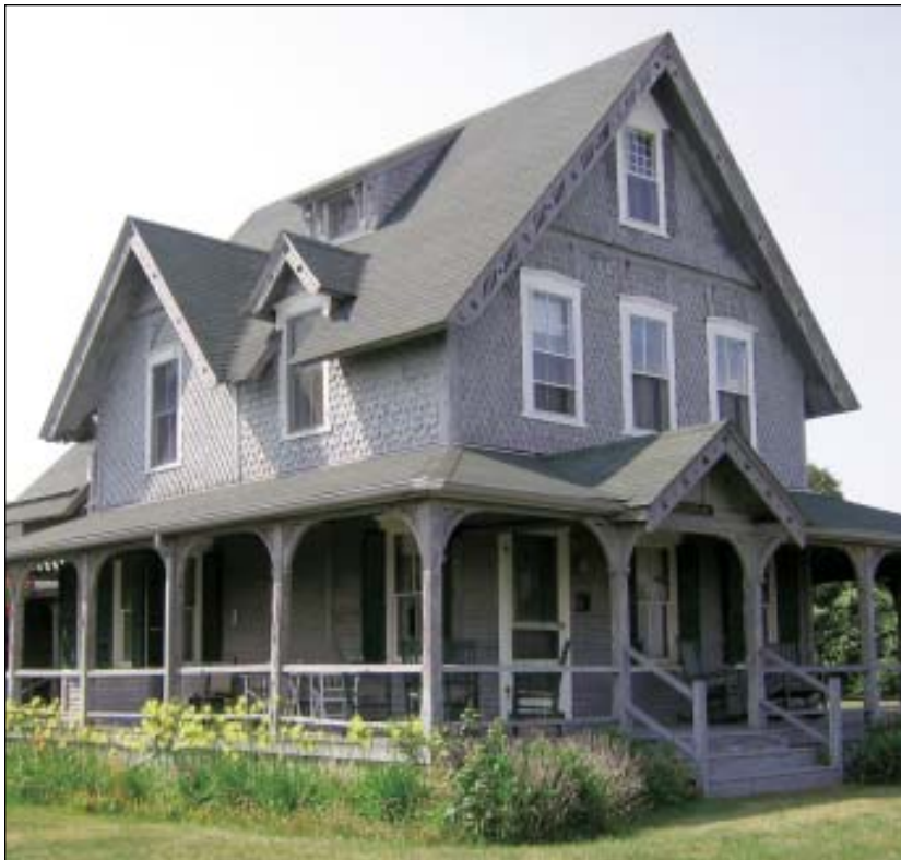
FIGURE 1. A striking example of the decorative use of pattern shingles is seen at Idlemoor — a home constructed on Nantucket Island in 1884. Most of original sidewall material (above) remains intact today.
