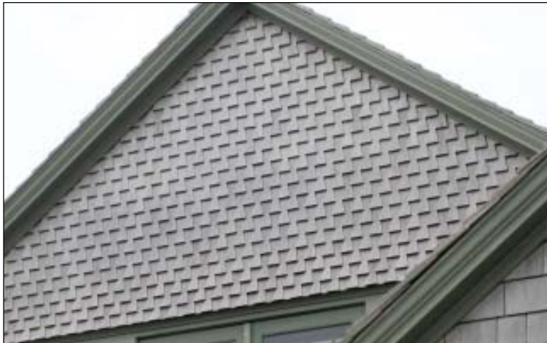
FIGURE 3. Similar to its use in the waterside gable at Idlemoor, this custom dovetail pattern creates a striking geometric effect. It requires extra effort to produce, however, so the authors limited it to the most prominent end of the house.
