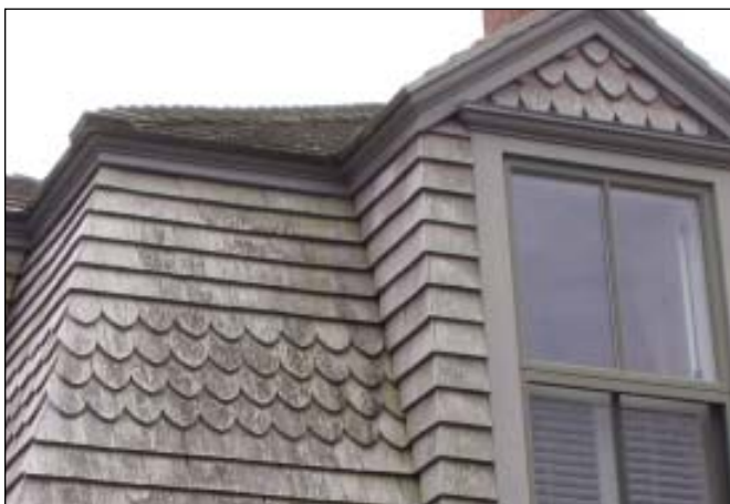
FIGURE 4. To complete the exterior restoration of Flaggship, circa 1890, the authors consulted historic photographs that revealed a decorative band of "fish scale" shingles on the home's mansard roof and inside the gable end of 12 dormers. The restoration work on this roof was completed by John Rex.
