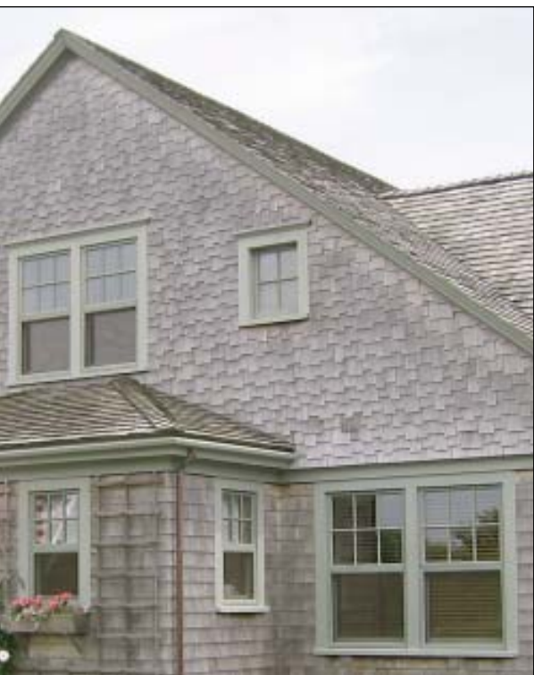
FIGURE 2. In a new house built by Edward O'Brien of Nantucket (left), the authors' design called for gable ends with a staggered pattern over a standard random-width pattern below. The patterns are separated by a continuous frieze of flared shingles and bed molding that wraps the first-floor plate line (illustration, below).
