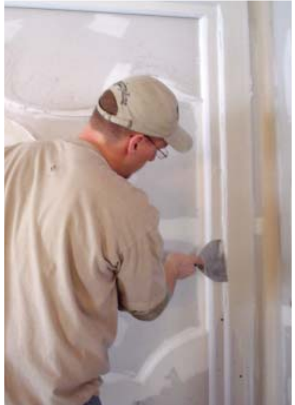
Figure 4. Except for mudding the edges of the cutouts, taping the mural is the same as for any wall (above). Sanding is more difficult. Here, the author uses a sanding sponge to smooth near an edge (left).
