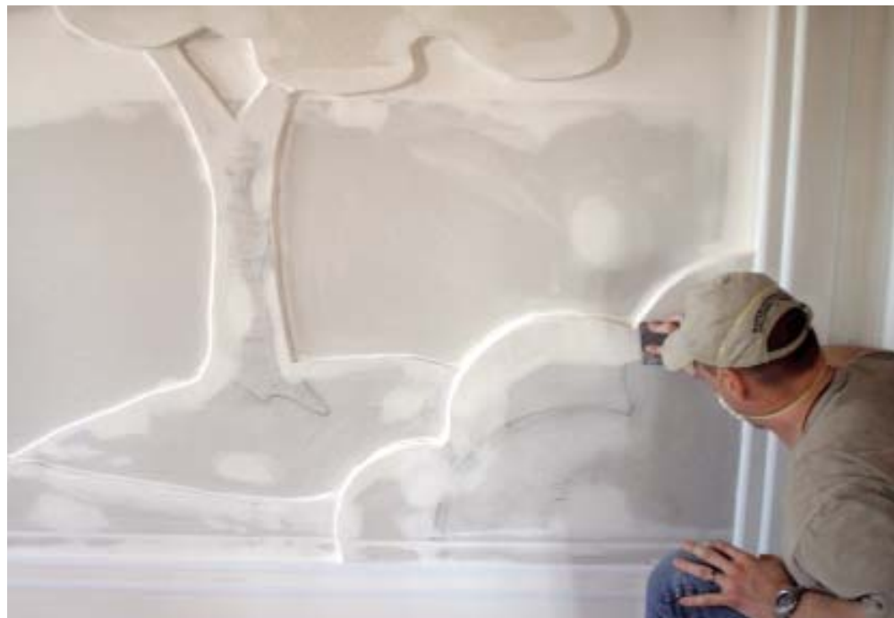
Figure 4. Except for mudding the edges of the cutouts, taping the mural is the same as for any wall (above). Sanding is more difficult. Here, the author uses a sanding sponge to smooth near an edge (left).
