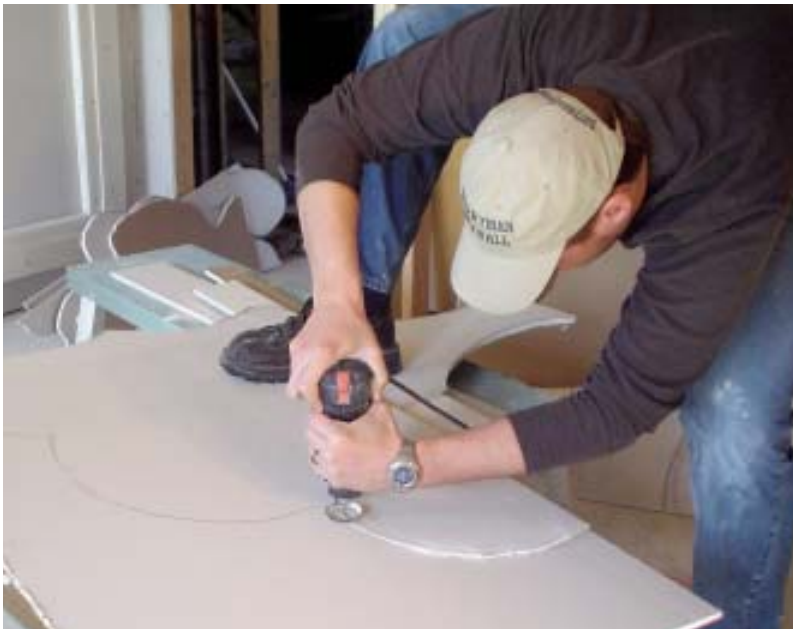
Figure 2. A spiral saw with a drywall bit is the best tool for cutting out irregular pieces.
