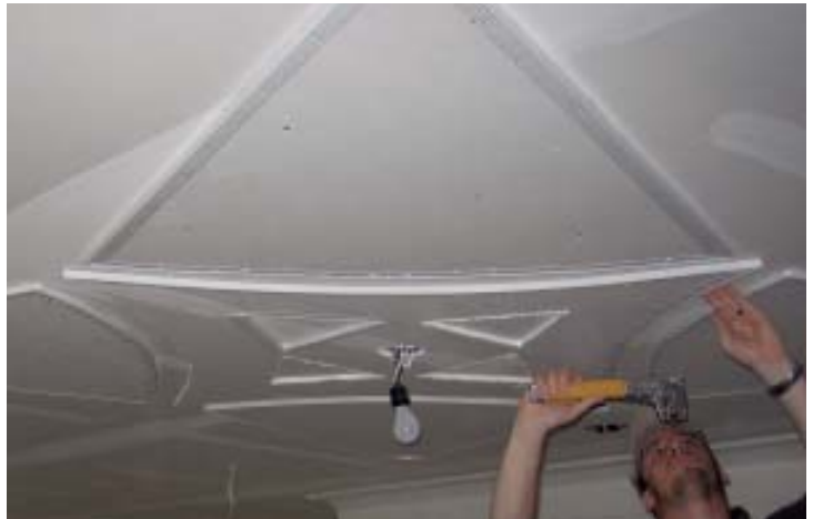
Figure 5. On the job featured in this story, the finished mural was painted shades of gray (left). A more subtle effect can be achieved by painting the raised areas the same color as the rest of the room (below left). On another job, the author applies vinyl bead to an abstract pattern on the ceiling (below).
