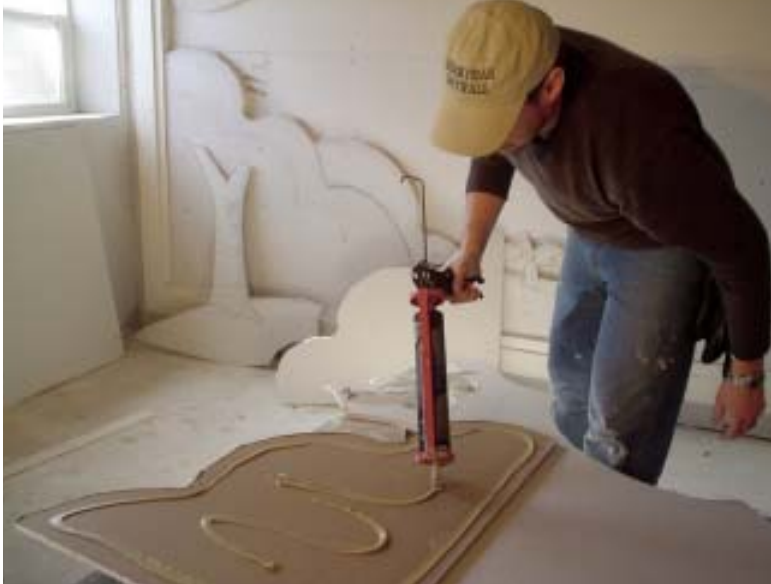
Figure 3. The author applies drywall adhesive to the back of a piece (left) before applying it to the wall (below left). At first, the layers are only roughly aligned; once all the pieces are up, the author trims and smooths edges with a utility knife. He uses drywall screws to catch whatever framing he can (bottom).
