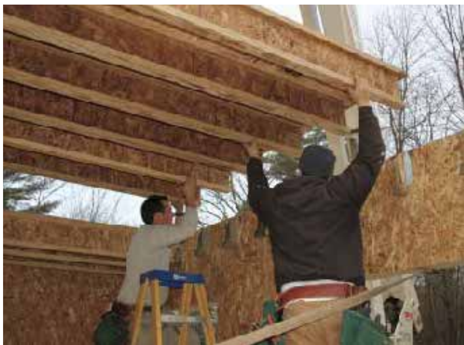
Figure 8. Just like the first-story SIP floors, the pre-assembled I-joist floor sections are flown into place with the crane (left). Previously installed joist hangers receive the I-joist ends as the floor sections drop into position (below).
