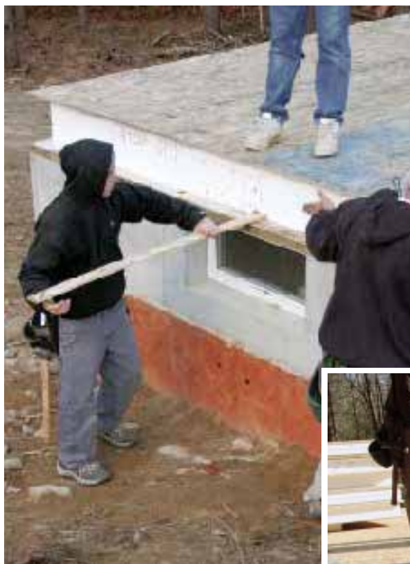
Figure 4. Prerouted grooves at panel edges receive 1/2-inch plywood splines (left), which the crew then staples at 4 inches on-center to stitch the panels together. At the perimeter, carpenters install full-height LVL rim joists (below), using 2.5-inch pneumatic nails. The LVL perimeter members are overkill in structural terms, but sawn lumber would shrink away from the panels and compromise the integrity of the joints.
