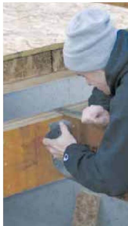
Figure 2. Larger and more complicated SIP floors need underfloor support. Parallam (left) and LVL (below left) beams match up well with SIPs because of their engineered strength, limited shrinkage, and dimensional consistency. A pneumatic palm nailer helps for driving hanger nails into the hard engineered beams (below).
