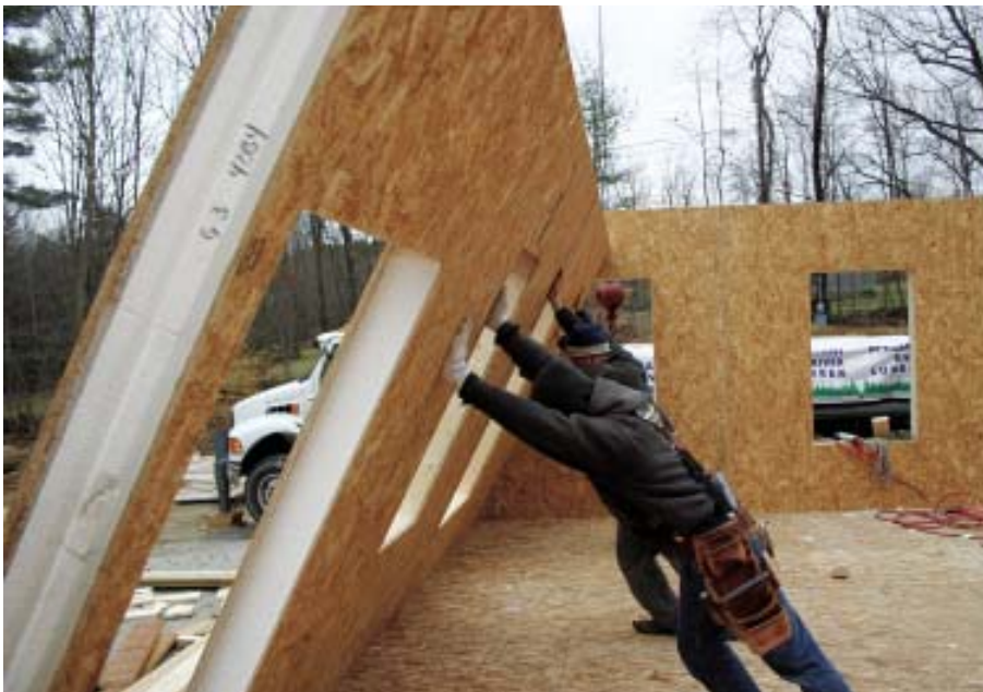
Figure 6. Where a beam end meets the wall above a window, foam is routed out of the panel at the opening edge of the window, allowing the crew to insert jack posts into the recess (above left). A built-up LVL header, sized to carry the load from the beam, is slipped into the panel above the window opening (above). The wall is then stitched together and raised (left).
