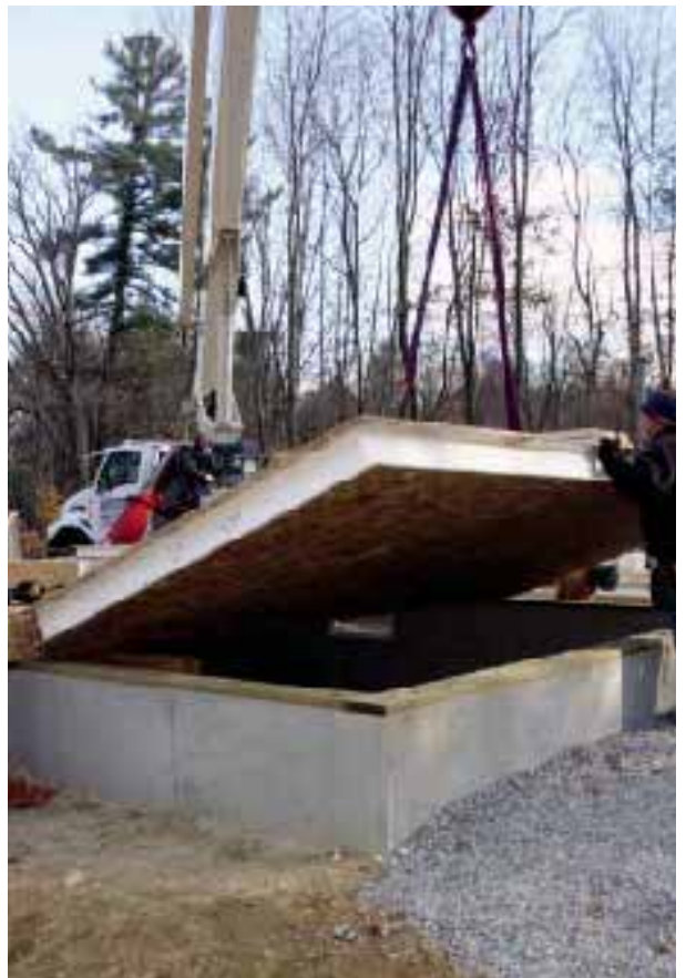
Figure 1. In preparation for the SIP floor for this 8-by-16-foot sunroom addition, the crew fastens an LVL ledger beam to the edge of the conventionally framed main floor (top left), leaving a shimmed space below the ledger to receive the bottom edge of the panel. The crane's straps attach to a steel plate that's screwed directly to the SIP (top right). While the floor panel is suspended from the crane, one crew member drills holes at anchor-bolt locations while another applies adhesive sealant to the treated-wood sill (above). Finally, the crane lowers the panel into place (right), where it will be nailed to the sill.
