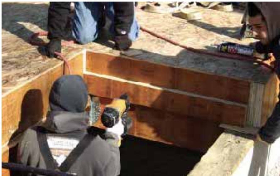
Figure 5. Where the plans call for a stepped-down entryway floor, a 6-inch panel is used to create the lower level. Here, the crew attaches an LVL ledger to the side of the main beam to catch the edges of the thinner panel (right). The 12-inch floor panel was a tight fit and required some persuasion from a come-along (below), but the 6-inch entryway panel slides easily into place with no argument (bottom).
