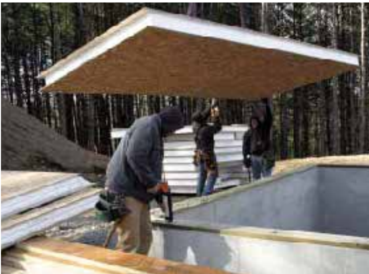
Figure 1. In preparation for the SIP floor for this 8-by-16-foot sunroom addition, the crew fastens an LVL ledger beam to the edge of the conventionally framed main floor (top left), leaving a shimmed space below the ledger to receive the bottom edge of the panel. The crane's straps attach to a steel plate that's screwed directly to the SIP (top right). While the floor panel is suspended from the crane, one crew member drills holes at anchor-bolt locations while another applies adhesive sealant to the treated-wood sill (above). Finally, the crane lowers the panel into place (right), where it will be nailed to the sill.
