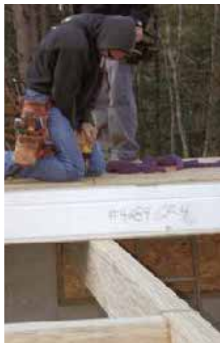
Figure 3. With the girders in place, the crane drops four 8-by-24-foot 12-inch-thick floor panels into position (above left). The perimeters are nailed to the pressure-treated sill (left), and panels are fastened to bearing beams with epoxy-coated self-tapping screws (above).
