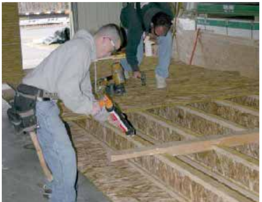
Figure 7. For this project, the crew preassembled second-story floor frames in the shop in 8-foot-wide sections (above). A simple 2x4 jig helps to keep floor joists aligned as floor sheathing is placed and fastened (right).
