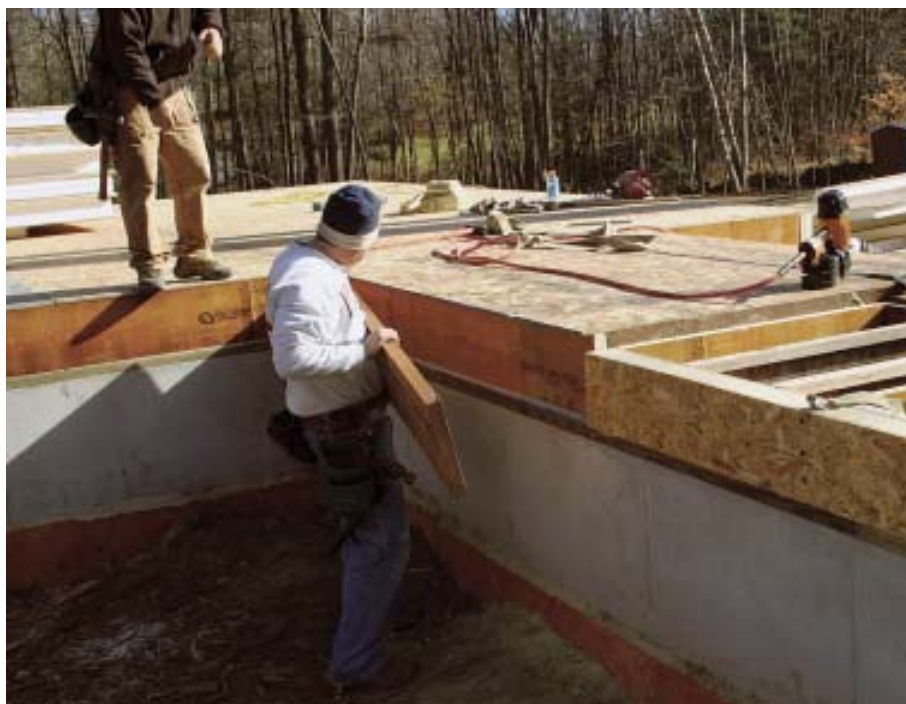
Figure 4. Prerouted grooves at panel edges receive 1/2-inch plywood splines (left), which the crew then staples at 4 inches on-center to stitch the panels together. At the perimeter, carpenters install full-height LVL rim joists (below), using 2.5-inch pneumatic nails. The LVL perimeter members are overkill in structural terms, but sawn lumber would shrink away from the panels and compromise the integrity of the joints.
