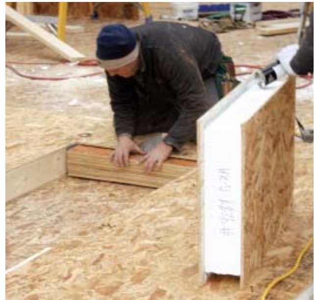
Figure 6. Where a beam end meets the wall above a window, foam is routed out of the panel at the opening edge of the window, allowing the crew to insert jack posts into the recess (above left). A built-up LVL header, sized to carry the load from the beam, is slipped into the panel above the window opening (above). The wall is then stitched together and raised (left).
