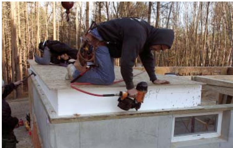
Figure 3. With the girders in place, the crane drops four 8-by-24-foot 12-inch-thick floor panels into position (above left). The perimeters are nailed to the pressure-treated sill (left), and panels are fastened to bearing beams with epoxy-coated self-tapping screws (above).
