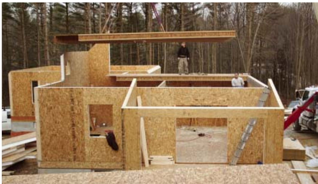
Figure 8. Just like the first-story SIP floors, the pre-assembled I-joist floor sections are flown into place with the crane (left). Previously installed joist hangers receive the I-joist ends as the floor sections drop into position (below).
