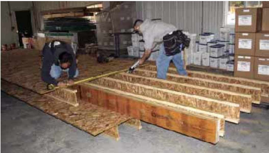
Figure 7. For this project, the crew preassembled second-story floor frames in the shop in 8-foot-wide sections (above). A simple 2x4 jig helps to keep floor joists aligned as floor sheathing is placed and fastened (right).
