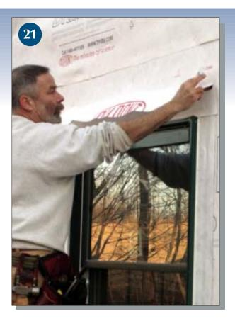
flange, coupled with the sloped sill, will provide a weep area for water to escape.
