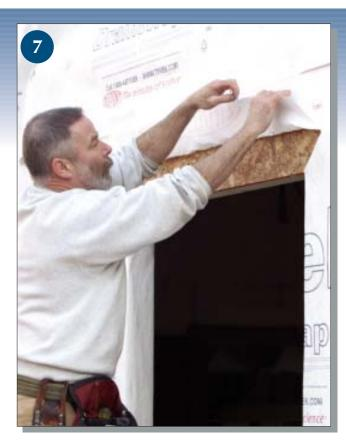
to install a window, my first step is to cut the wrapped window opening. I start by making a level head cut (1), then two 45-degree cuts upward from the lower corners (2). I finish with a vertical cut (3).
