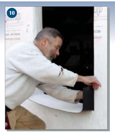
the sill flashing. I prefer to use Tyvek FlexWrap, a butyl-based self-healing flashing product I call "peel-and-stick on steroids." It has all the self-healing characteristics of generic peel-and-stick, but it also can be stretched to form seamless sill corners.
