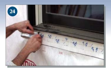
and "skip-tape" (apply short pieces of tape with gaps in between) the lower edge of the flap in place **(23)**. I also skip-tape the bottom (uncaulked) sill flange **(24)**. These skip-taped gaps at the lower edges act as weeps, giving any moisture that gets to the window head a way to escape. Skip-taping also limits air leaks, though it's not entirely airtight. (For my money, I'd take an air leak over a moisture problem any day.)
