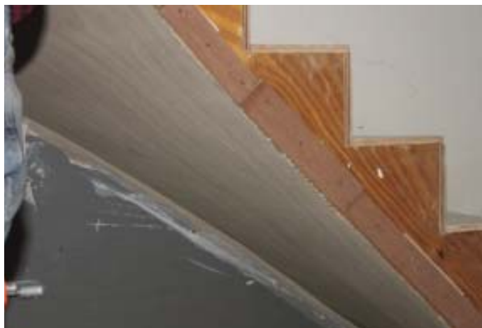
Figure 9. A plaster scratch coat establishes a rough plane against which the face skirtboards can be scribed (left). The author cleans up the skirt's curving profile before gluing on a decorative edge bead (above left). After the face skirt is installed (above), the final plaster coat will fill any gaps and provide a smooth surface that flows between ceiling levels.
