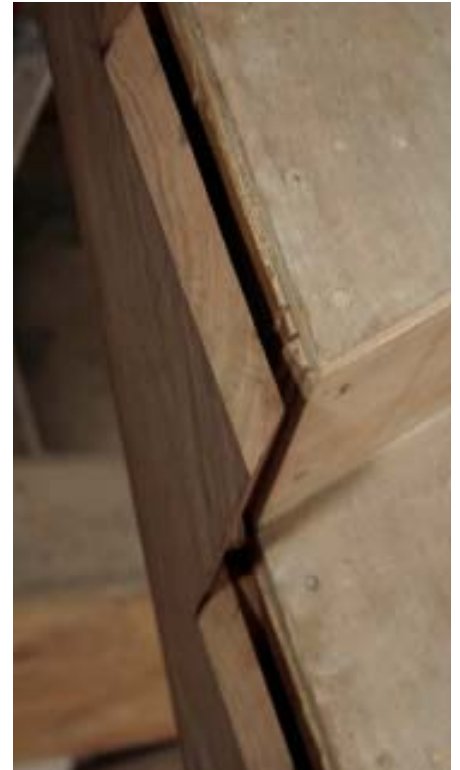
Figure 10. The author uses a 45-degree default angle for the vertical skirt cuts and adjusts the finished riser angles individually. The shim space behind the skirt allows the miter joints to be adjusted plumb and tight.
