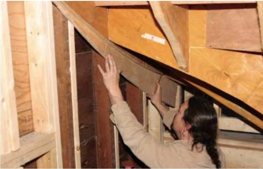
Figure 6. Carpenter Mike Kennedy adds a plywood batten beneath the wall stringer to create a visually fair line for the plaster furring to follow.
