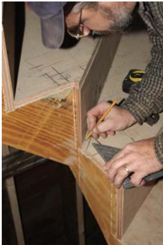
Figure 8. The author lays out the newel notch directly on the winders (left), then transfers the information to the post. After notching, the post is positioned (below left), then shimmed plumb and bolted from the back (below). Plugged bolts are added later through the face for reinforcement.
