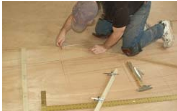
Figure 4. By laying the story pole perpendicular to the plan and snapping out riser lines, the author can project full-scale templates for the rough stringers.
