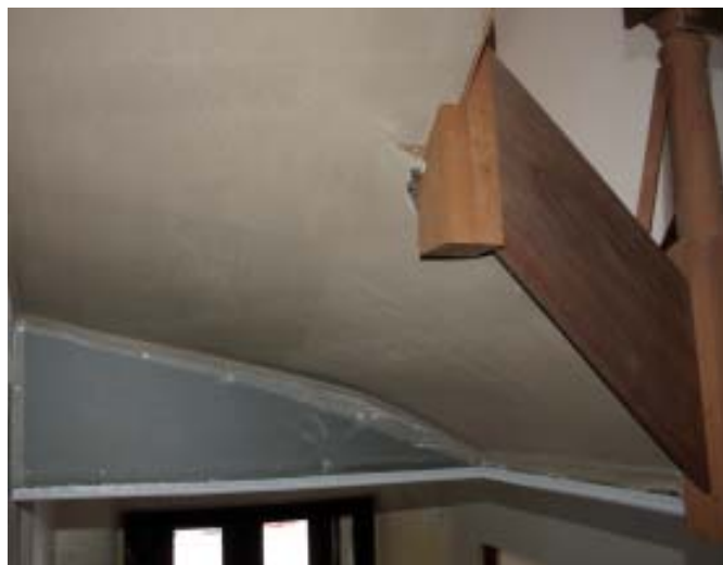
Figure 9. A plaster scratch coat establishes a rough plane against which the face skirtboards can be scribed (left). The author cleans up the skirt's curving profile before gluing on a decorative edge bead (above left). After the face skirt is installed (above), the final plaster coat will fill any gaps and provide a smooth surface that flows between ceiling levels.
