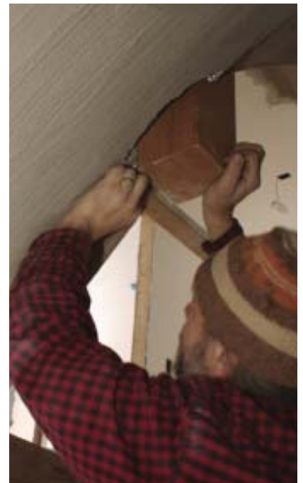
Figure 8. The author lays out the newel notch directly on the winders (left), then transfers the information to the post. After notching, the post is positioned (below left), then shimmed plumb and bolted from the back (below). Plugged bolts are added later through the face for reinforcement.
