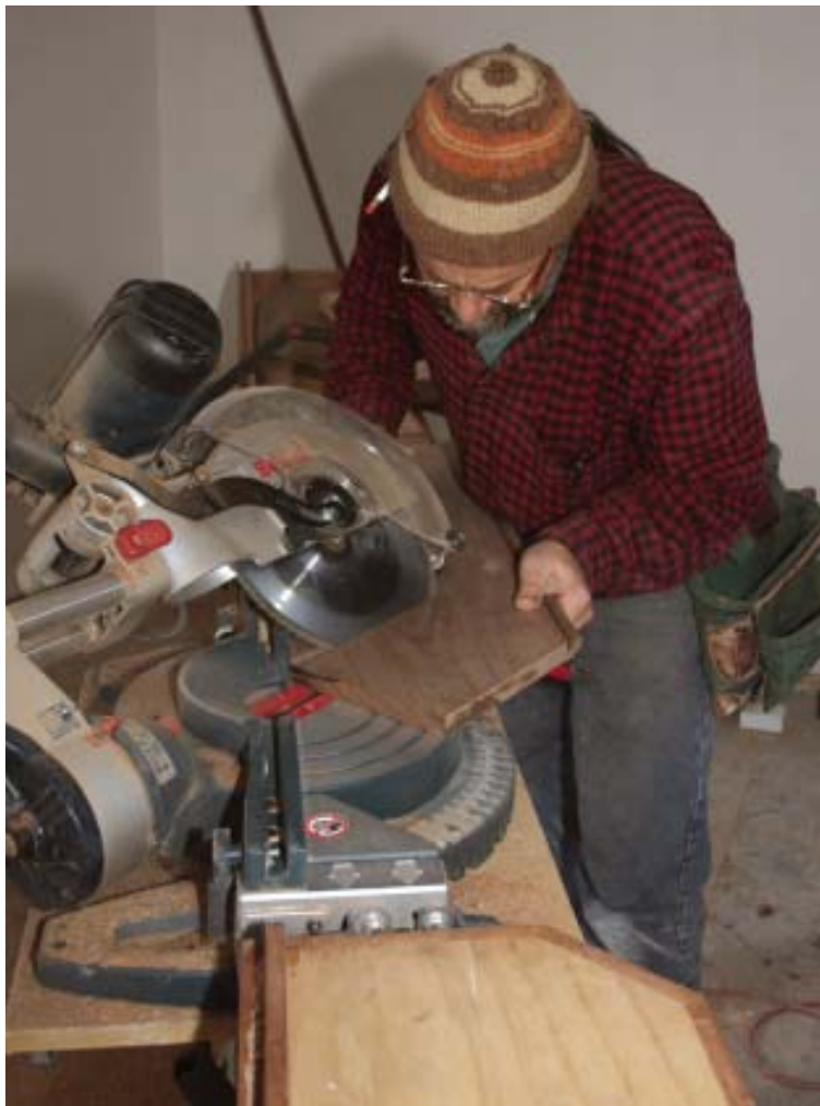
Figure 10. The author uses a 45-degree default angle for the vertical skirt cuts and adjusts the finished riser angles individually. The shim space behind the skirt allows the miter joints to be adjusted plumb and tight.
