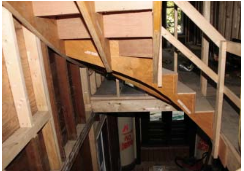
Figure 5. Shear-rated lag screws connect intersecting stringers and fasten the inside members to the walls. Plywood subrisers and treads, installed with screws and construction adhesive, convert the individual stringers into a strong monolithic structure. Temporary, 2x4 guardrails, screwed together for easy removal, provide fall protection for workers using the rough stair.
