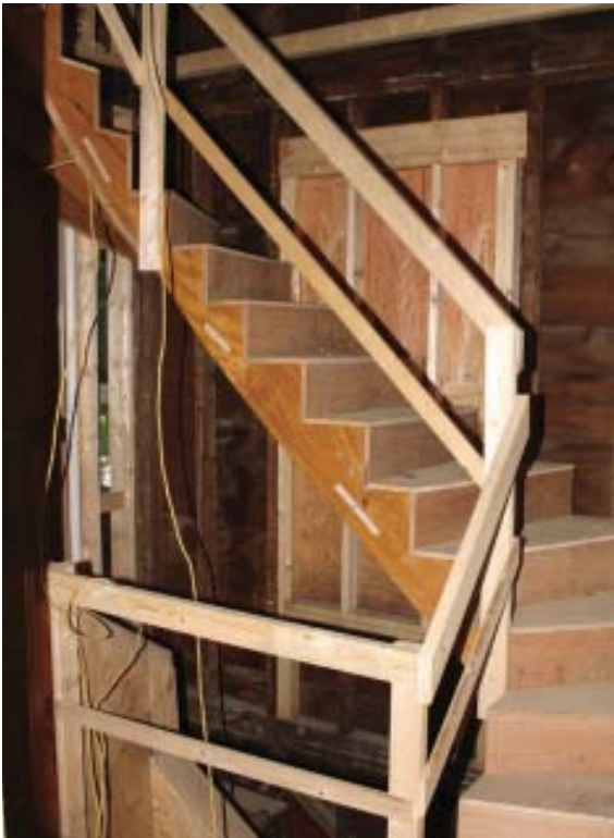
Figure 5. Shear-rated lag screws connect intersecting stringers and fasten the inside members to the walls. Plywood subrisers and treads, installed with screws and construction adhesive, convert the individual stringers into a strong monolithic structure. Temporary, 2x4 guardrails, screwed together for easy removal, provide fall protection for workers using the rough stair.
