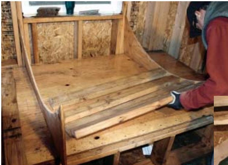
Figure 7. The barrel portion — or the arch — is framed like an arched door opening with flat 2x4 purlins sandwiched between curved plywood pieces (left). This barrel was small enough to be lifted into place by two men (below).
