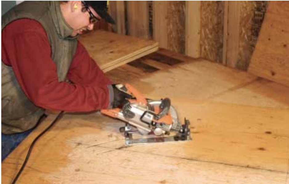
Figure 6. In this case, the elliptical curve is shallow enough to be cut with a circular saw. Only the top 12 inches of the ellipse — the height of the barrel — is needed.
