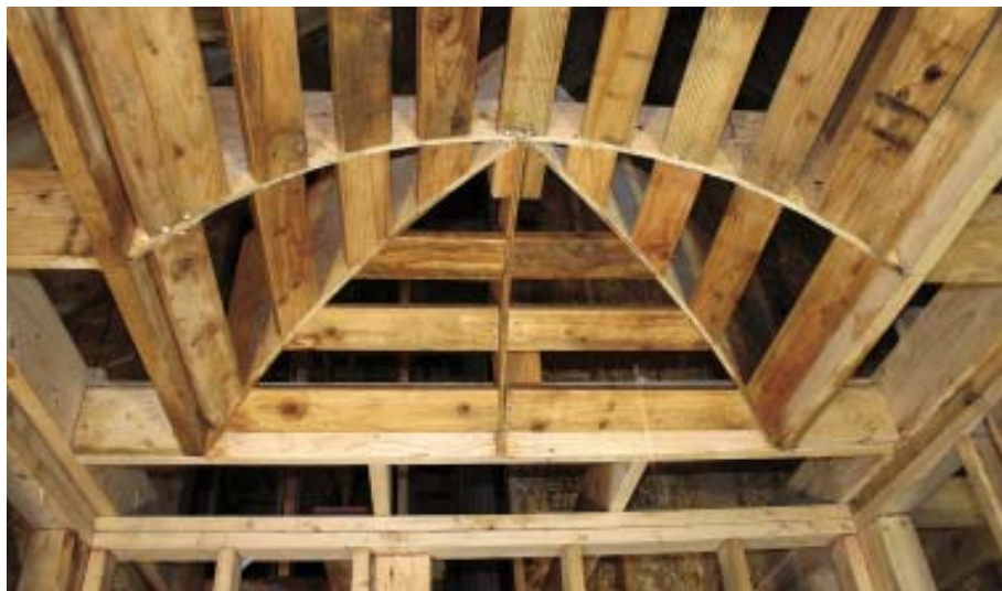
Figure 9. The purlins at the ends of the vault have straight cuts on one end and compound miters on the other.
