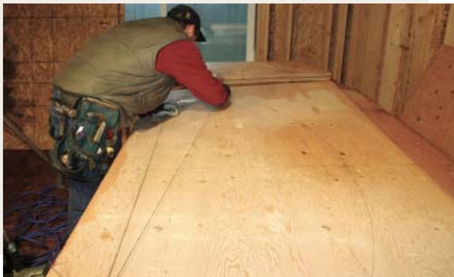
Figure 5. After pulling the temporary tack, a carpenter inserts a pencil where the picture wire passes over the top of the minor axis (left). He then scribes the ellipse by sliding the pencil firmly against the wire, which he is careful to keep taut (below).
