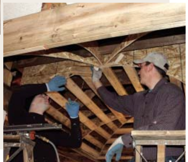
Figure 2. On upper floors, the opening for a barrel vault can be created by heading off ceiling joists (left). In rooms with high ceilings, the vault may fit in a dropped soffit (below).
