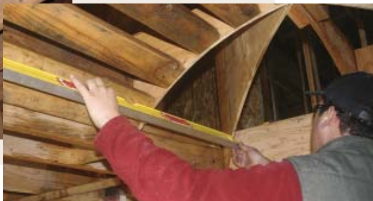
Figure 8. After the barrel is positioned (left), the king common and the elliptical “hip” are installed. Here, a carpenter uses a straightedge to verify that the barrel surfaces are in the same plane as the hip end (below).
