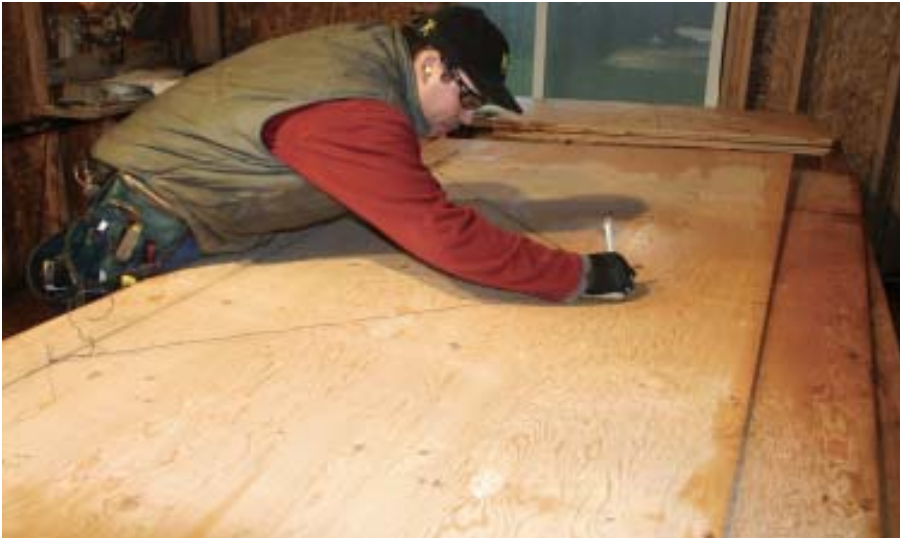
Figure 5. After pulling the temporary tack, a carpenter inserts a pencil where the picture wire passes over the top of the minor axis (left). He then scribes the ellipse by sliding the pencil firmly against the wire, which he is careful to keep taut (below).
