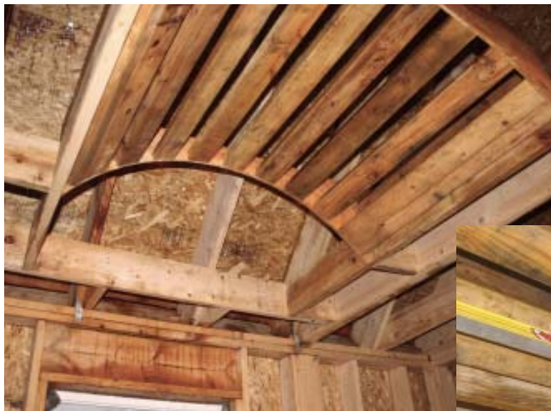
Figure 8. After the barrel is positioned (left), the king common and the elliptical “hip” are installed. Here, a carpenter uses a straightedge to verify that the barrel surfaces are in the same plane as the hip end (below).
