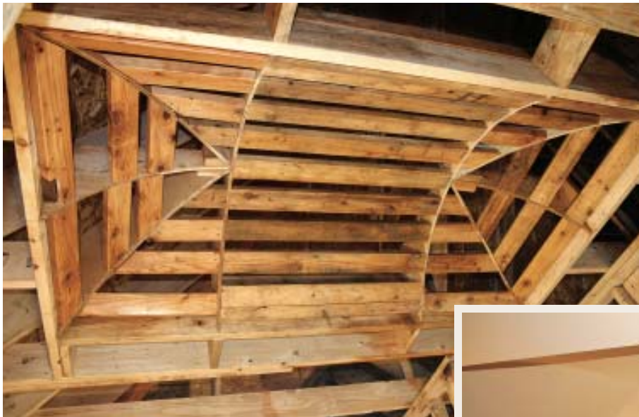
Figure 1. The vault framing (left) consists of radiused plywood “rafters” at the sides and ends, and elliptical plywood “hips” at the corners (drawing, bottom). Two-by-four “purlins” run between the plywood pieces. The surface is finished later with a double layer of \frac{1}{4} -inch drywall (below).
