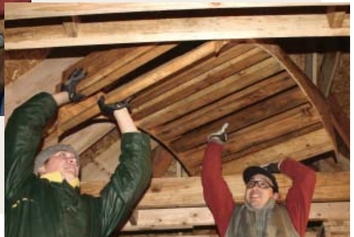
Figure 7. The barrel portion — or the arch — is framed like an arched door opening with flat 2x4 purlins sandwiched between curved plywood pieces (left). This barrel was small enough to be lifted into place by two men (below).
