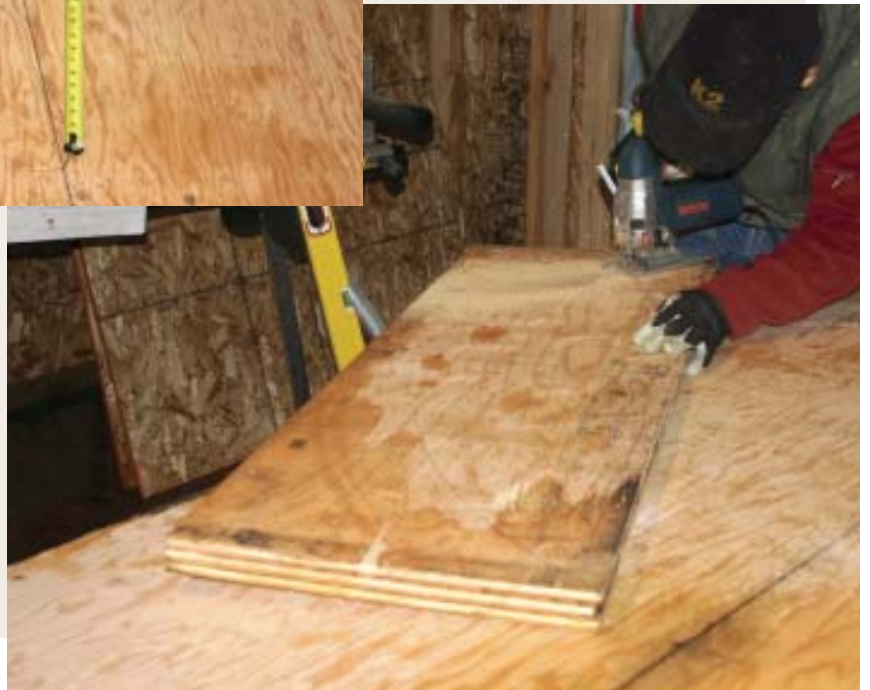
Figure 4. The blanks for the arc segments are as long as the opening is wide. After marking the radius on the top piece (left), a carpenter cuts three arcs at once (below).
