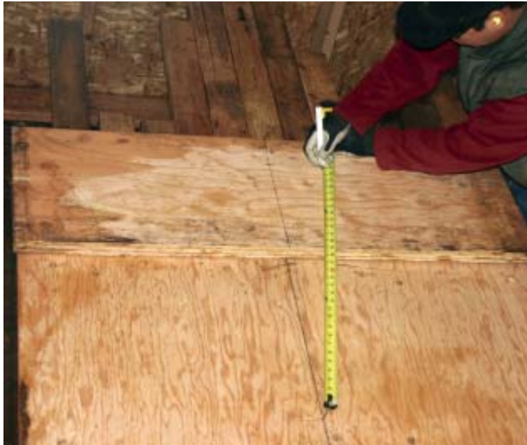
Figure 4. The blanks for the arc segments are as long as the opening is wide. After marking the radius on the top piece (left), a carpenter cuts three arcs at once (below).
