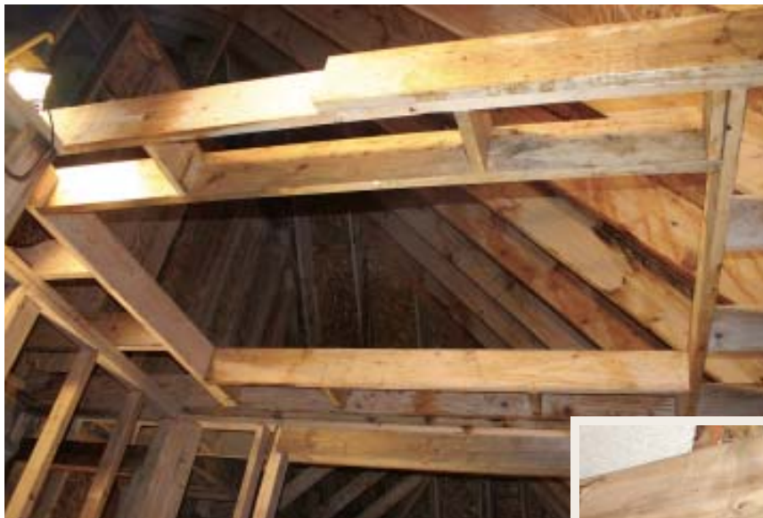
Figure 2. On upper floors, the opening for a barrel vault can be created by heading off ceiling joists (left). In rooms with high ceilings, the vault may fit in a dropped soffit (below).
