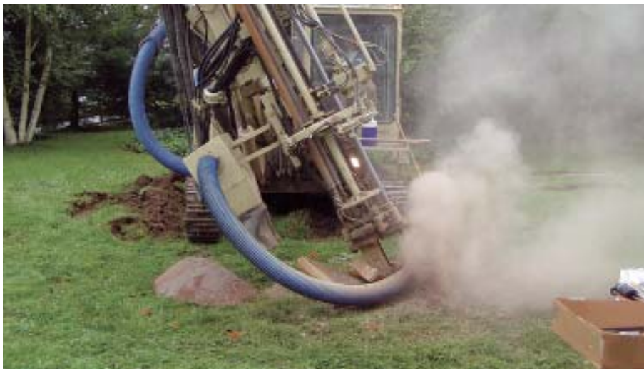
Figure 1. Because direct-exchange technology is so efficient at collecting the heat of the earth, installations are possible even on small lots. While trenches or pits are less expensive, drilling — either vertically or at an angle — makes it possible to work around ledge or in tight quarters.
