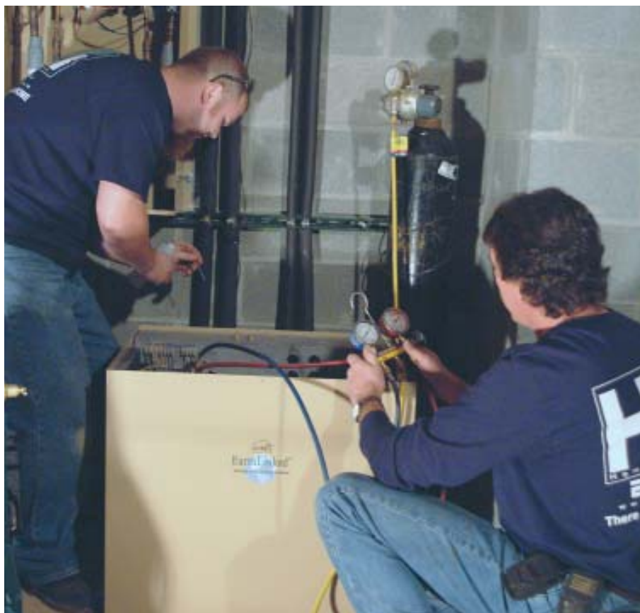
Figure 4. Unlike standard air-source heat pumps, geothermal condensers do not require air circulation, so they can be installed in a basement or utility room, which lengthens service life.
