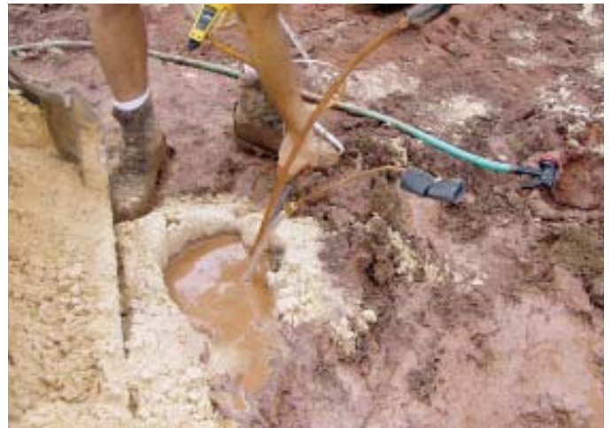
Figure 2. Rather than PEX tubing, which is used in conventional geothermal heating, direct-exchange systems use copper for a highly efficient heat transfer. (In some cases, corrosive soils may prevent installation.) Normally, the copper is protected by sand, which is installed in a slurry to ensure good coverage and optimum heat transfer. In areas where excessive groundwater might pipe away the sand, a special grout is used instead.
