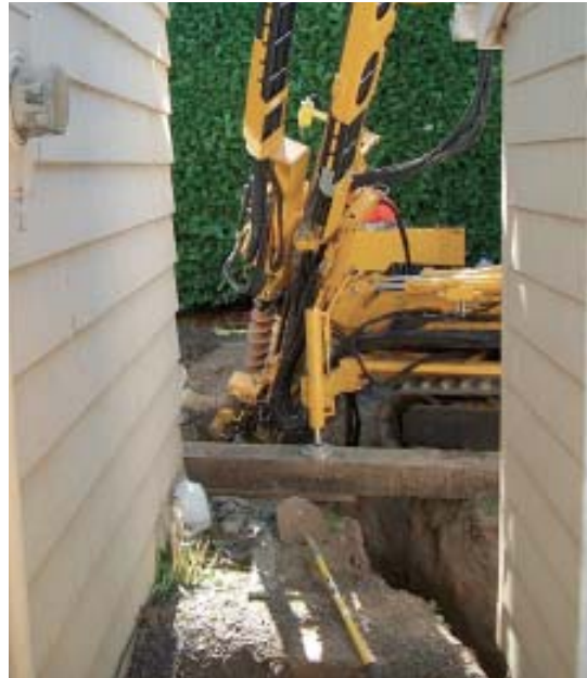
Figure 1. Because direct-exchange technology is so efficient at collecting the heat of the earth, installations are possible even on small lots. While trenches or pits are less expensive, drilling — either vertically or at an angle — makes it possible to work around ledge or in tight quarters.
