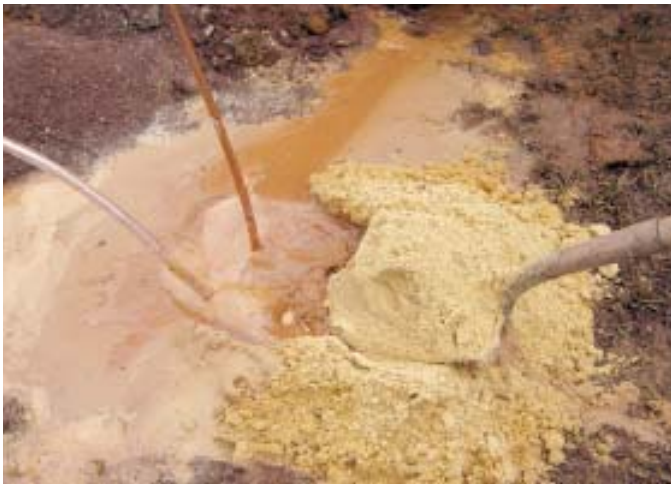
Figure 2. Rather than PEX tubing, which is used in conventional geothermal heating, direct-exchange systems use copper for a highly efficient heat transfer. (In some cases, corrosive soils may prevent installation.) Normally, the copper is protected by sand, which is installed in a slurry to ensure good coverage and optimum heat transfer. In areas where excessive groundwater might pipe away the sand, a special grout is used instead.
