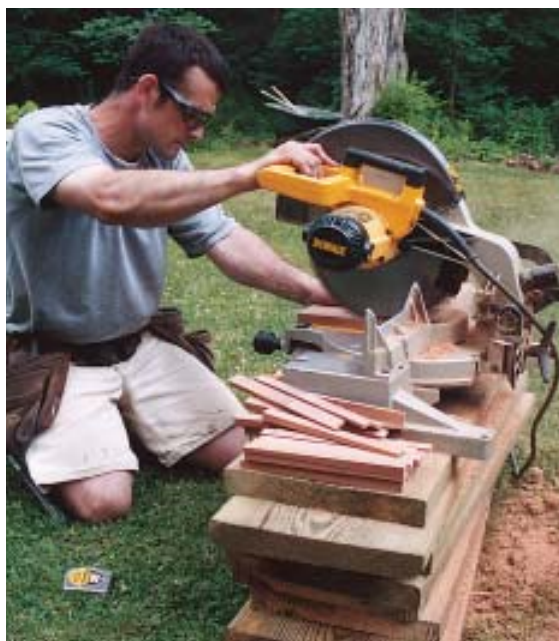
Figure 4. Cut from 9-inch-long scrap riser material, the wedges are beveled at 4 degrees, which is done by setting the saw to 2 degrees and flipping the stock end-for-end at each cut. The carpenter eyeballs the cuts so that the sharp ends of the wedges measure about \frac{3}{16} inch.
