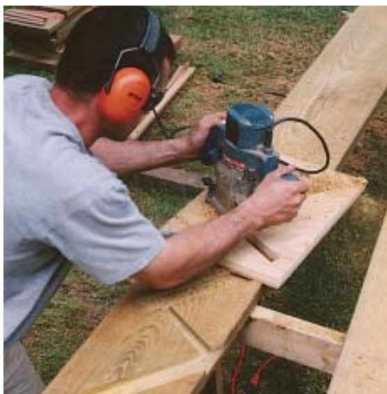
Figure 3. Using a plunge router with a \frac{3}{4} -inch-diameter pattern routing bit, the carpenter cuts \frac{1}{2} -inch-deep mortises in two passes. The jig is clamped to the stringer so that the top of the tread and the front of the riser align with the layout marks.
