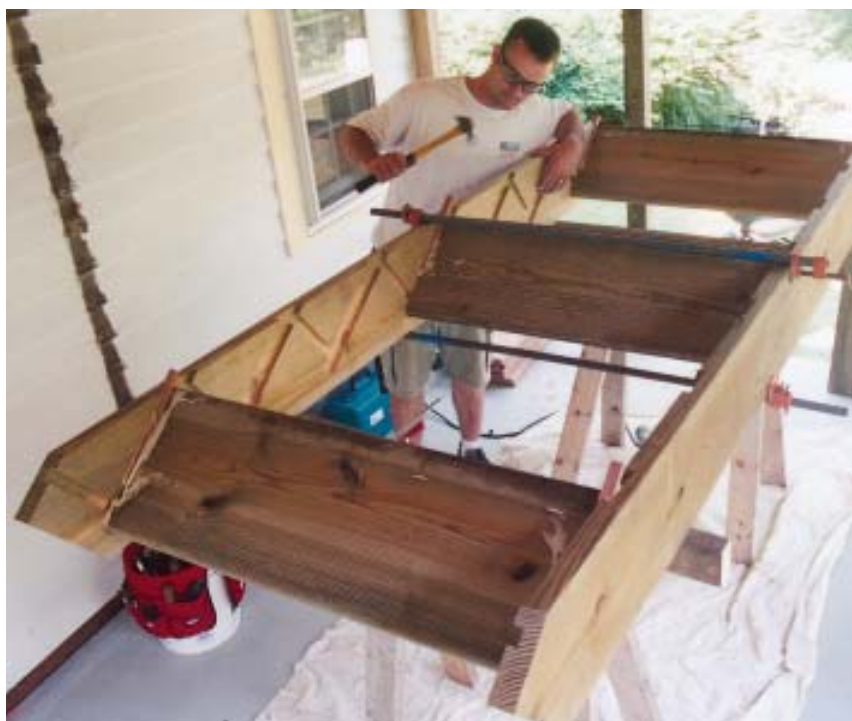
Figure 5. With the tread seated and the stringers bar-clamped together, the carpenter drives home a heavily glued wedge on each side.
