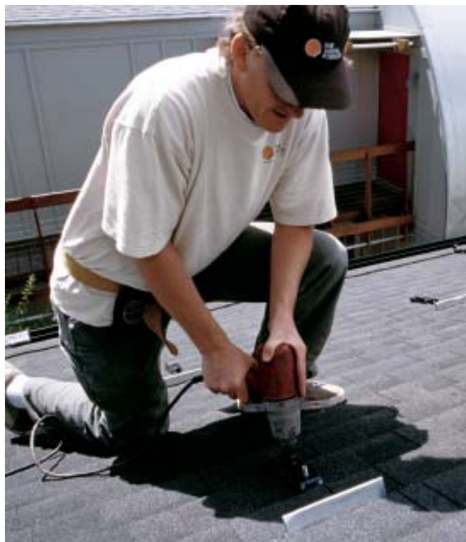
Figure 4. It's common to retrofit systems to buildings with existing shingle roofs. In the photo above, an installer caulk the back of a Tile Trac mounting bracket before bolting it through the shingles to the rafter below. Metal flashings (right) are installed upslope to divert rainwater from the penetration.
