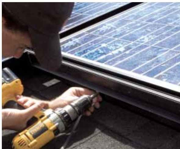
Figure 8. Modules should be grounded to each other and to the rack with a continuous ground wire. On this project, the installer is using a length of tinned copper braid to ground the array.
