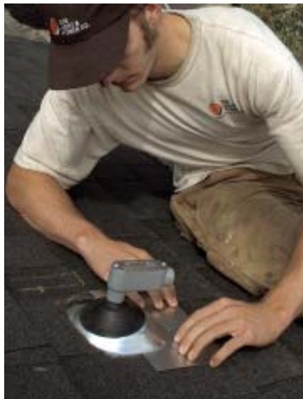
Figure 6. The crew uses a standard roof flashing with a self-sealing collar to waterproof the opening where electrical conduit penetrates the roof.
