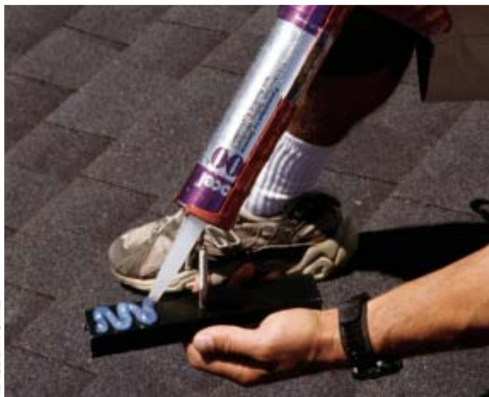
Figure 4. It's common to retrofit systems to buildings with existing shingle roofs. In the photo above, an installer caulk the back of a Tile Trac mounting bracket before bolting it through the shingles to the rafter below. Metal flashings (right) are installed upslope to divert rainwater from the penetration.
