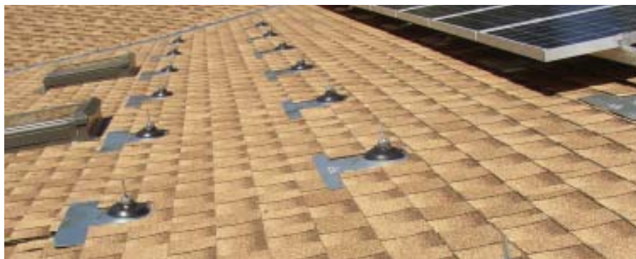
Figure 3. Post mounts are designed for new construction and should be installed, flashed, and shingled over before the rails and modules go on. Rails and modules are already attached to the mounts upslope and will soon be bolted to the mounts at left in this photo.
