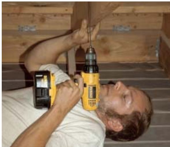
Figure 5. An installer locates the first roof mount by drilling a pilot hole next to a rafter. Other rafters are located from above by measuring off the protruding bit. To prevent leaks, the installer fills the hole with sealant and covers it with the mount.
