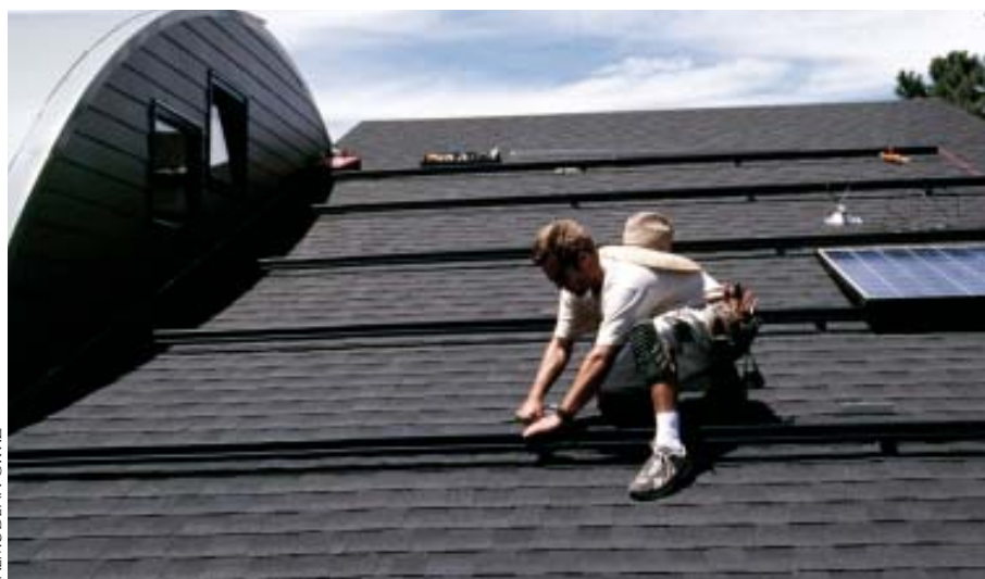
Figure 1. Here, an installer bolts a mounting rail to the roof. Modules usually sit on top of rails, but with this low-profile rack they will drop between rails and be a couple of inches closer to the roof than is typical.
