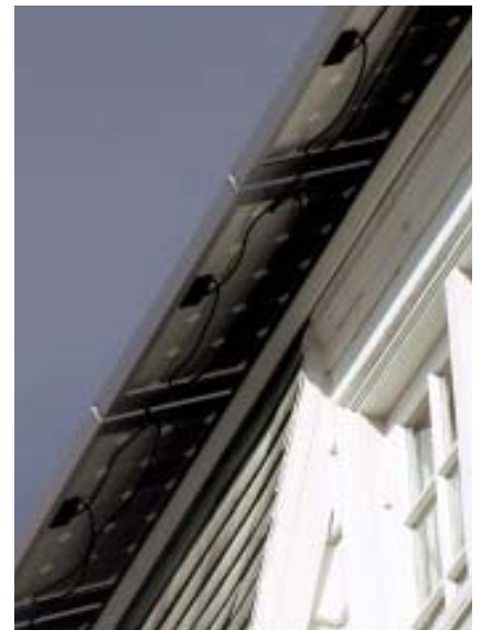
Figure 7. On a series-connected system, adjoining modules are connected positive to negative in much the same way as batteries in a flashlight.
