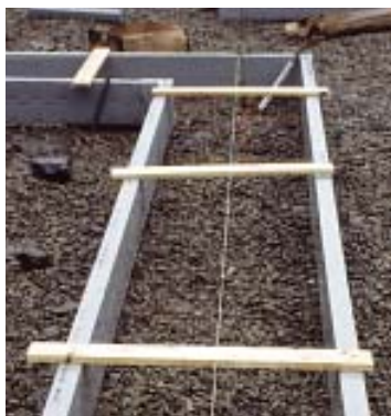
Figure 5. Once one side of the form is positioned, spacer straps automatically locate the opposite side (above). Pieces of strapping secured with drywall screws (right) are a good solution when you don't have the right size, or for nonstandard footing widths.
