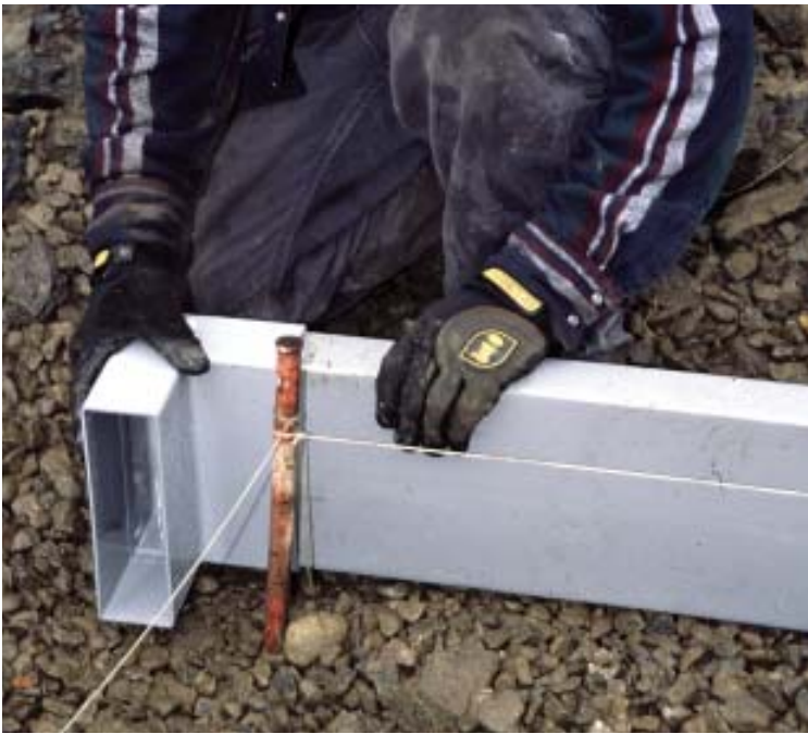
Figure 2. The author determines the footing location by measuring from a string representing the outside of the foundation wall (left). At footing corners, short rebar pins driven into the ground hold corner forms in place. A knockout hole in the bottom of the corner (above) receives the pin.
