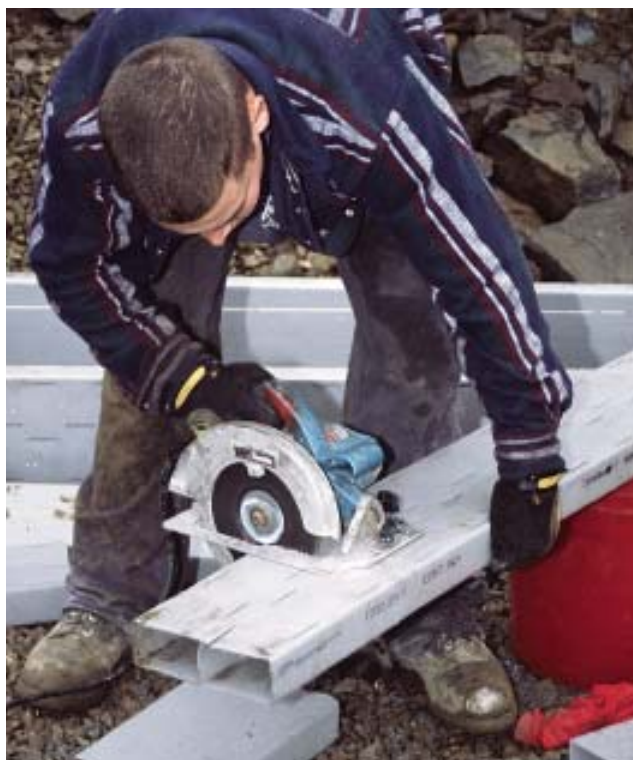
Figure 4. A circular saw equipped with a cutoff blade produces a fast, clean cut (left). Lengths of Form-A-Drain are divided into two chambers (above); this adds rigidity, and is useful for radon control applications in which the upper chamber is connected to a vent system powered by an in-line fan.
