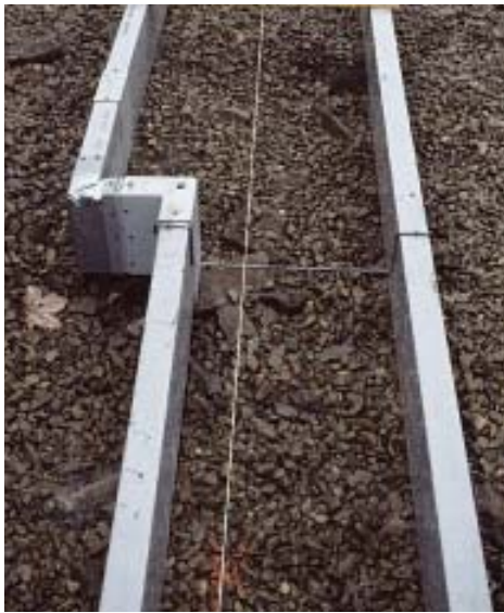
Figure 7. Where this footing transitioned from 16 to 24 inches (left), there wasn't enough room for two corners. A shortened corner patched with duct tape solved the problem (above).
