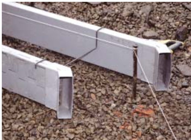
Figure 1. A worker secures a preformed corner with drywall screws (right). Preformed 45-degree bends are also available (below). Vertical 90s and tees are handy for stepped footings (bottom).
