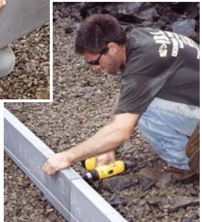
Figure 3. Lengths of Form-A-Drain are joined with slip couplings and drywall screws.
