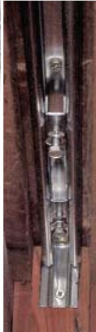
Figure 4. Here, the new track is in place, with the tab at the end secured to the stud at the back of the recess.
