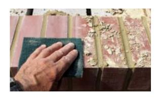
simply rub the face of the bricks lightly with my dry abrasive pad, being careful not to dig into the joints or use any water (above). This step is similar to the initial cleanup of freshly grouted tile.
