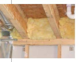
**Band Joist Batts.** Insulating the band joist is one of those important jobs nobody likes to deal with, so anything that makes the process faster and easier deserves a look. *SpeedyR Bandit* fiberglass insulation from CertainTeed is made specifically for
