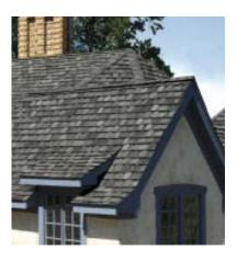
60 percent thicker than the layers in other premium asphalt shingles. The 7<sup>1</sup>/2-inch exposure should speed installation — provided you can get the shingles delivered and don't have to hump the seven-bundle squares up a ladder. The manufacturer claims that they cost a fraction of the price of cedar or slate.
