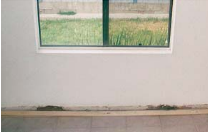
Figure 2. Water stains and mildew behind the baseboard underneath the window hint at the damage in the wall (above). Removing the drywall revealed the extent of the damage (right), including rotted framing and extensive termite infestation (below right).
