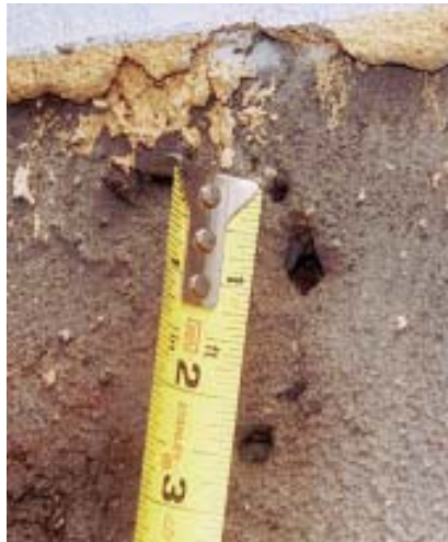
Figure 3. When the author directed his firm's spray rack at the window, water began pouring into the interior (above left). Once the trim was removed (above), it became obvious that holes blown through the stucco by the trim nails were the path for the water intrusion; some were 1/4 inch or more in diameter (left).
