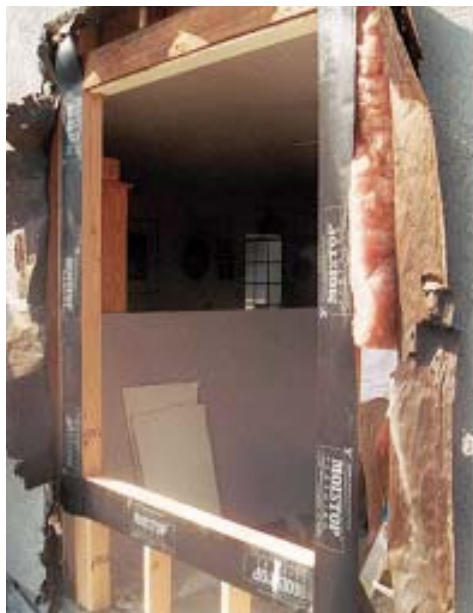
Figure 4. To repair the wall, the author replaced the damaged framing and added blocking (far left), which provided solid backing for Moistop waterproofing membrane. The Moistop was first applied to the sill and jambs (left); later, after applying sealant to the flanges, the crew installed the window (below left) and then applied Moistop over the head flange (below).
