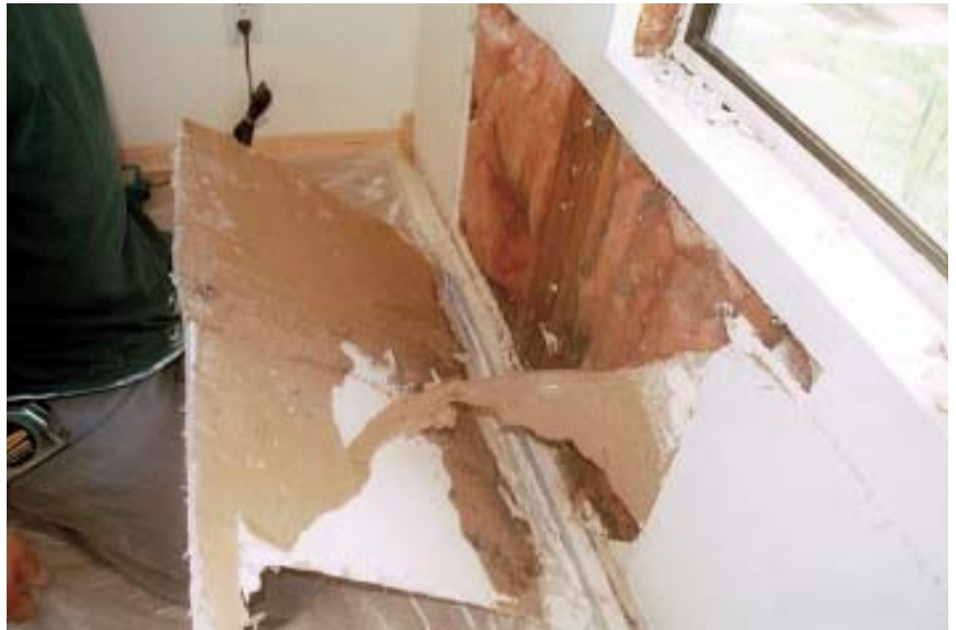
Figure 2. Water stains and mildew behind the baseboard underneath the window hint at the damage in the wall (above). Removing the drywall revealed the extent of the damage (right), including rotted framing and extensive termite infestation (below right).
