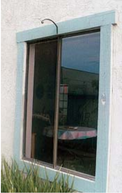
Figure 1. Though there was no obvious damage, the window of this Southern California condominium complex leaked every time it rained (left). Underneath the traditional three-coat stucco exterior, water had caused severe rot (above).
