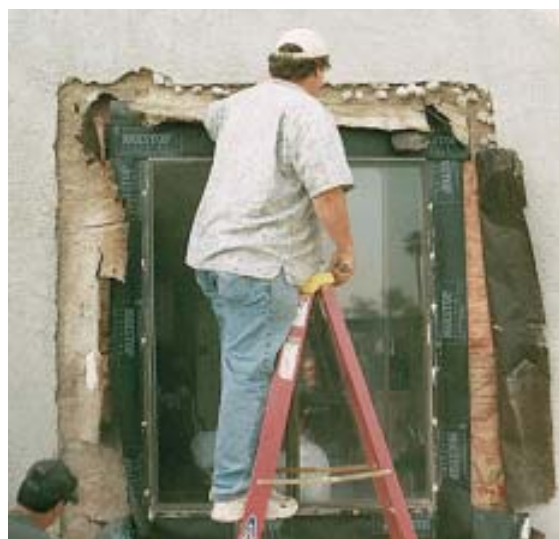
Figure 4. To repair the wall, the author replaced the damaged framing and added blocking (far left), which provided solid backing for Moistop waterproofing membrane. The Moistop was first applied to the sill and jambs (left); later, after applying sealant to the flanges, the crew installed the window (below left) and then applied Moistop over the head flange (below).
