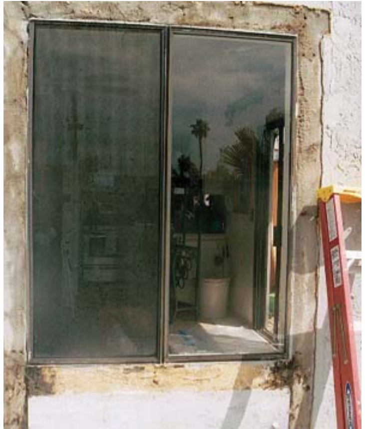
Figure 3. When the author directed his firm's spray rack at the window, water began pouring into the interior (above left). Once the trim was removed (above), it became obvious that holes blown through the stucco by the trim nails were the path for the water intrusion; some were 1/4 inch or more in diameter (left).
