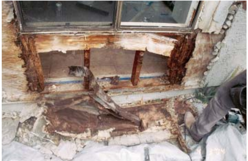
Figure 1. Though there was no obvious damage, the window of this Southern California condominium complex leaked every time it rained (left). Underneath the traditional three-coat stucco exterior, water had caused severe rot (above).
