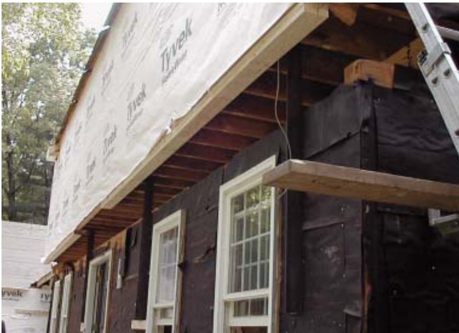
Figure 7. To prevent the upper story from being displaced when it was lifted, the author installed 4-inch steel angles to restrain it (above). At the overhanging front elevation (left), the crew cut L-shaped slots for the angles to pass through the second-story floor (below).
