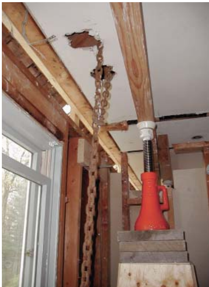
Figure 8. As a precaution against sudden strong gusts of wind, the crew tied the front and back of the house to the first story with a pair of heavy chains.
