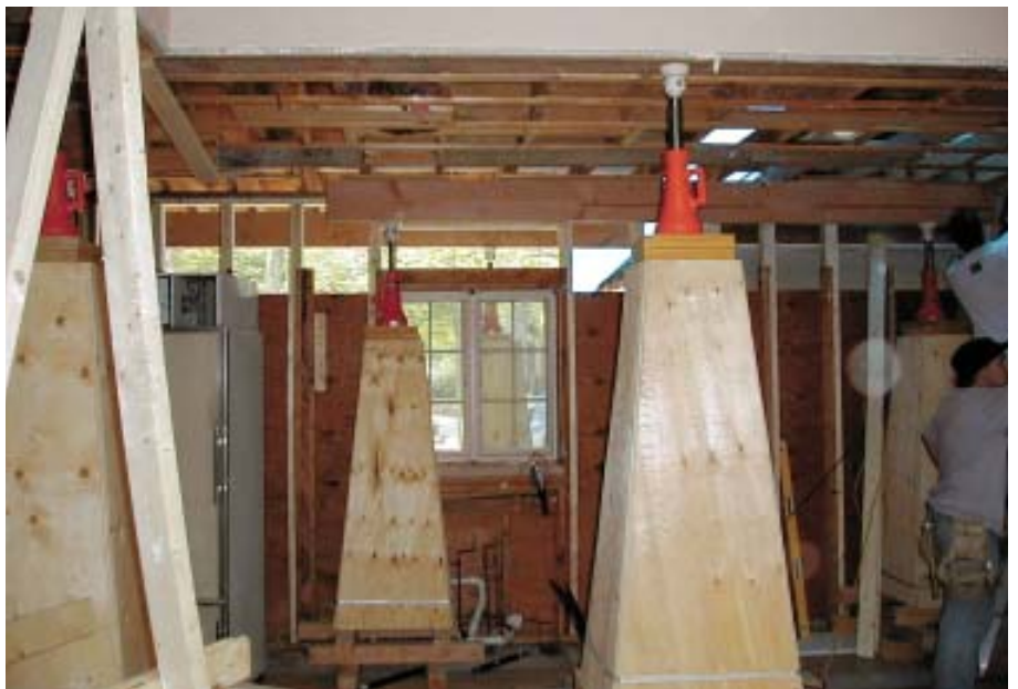
Figure 3. Site-built pyramidal jacking stands safely extended the screw jacks' reach to just below the lifting beams.
