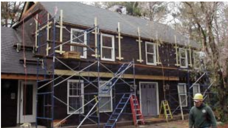
Figure 2. To maintain the original alignment and prevent the roof structure from shifting during lifting, the author's crew bolted 2x4 vertical struts to the tops of the walls around the house's perimeter.
