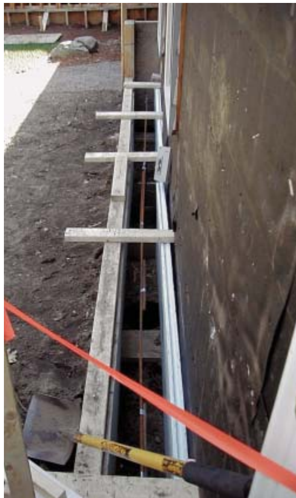
Figure 9. A new grade-beam concrete foundation, poured directly along the existing basement wall, and new wall framing provided direct support to eliminate the overhang of the second-story eaves wall.
