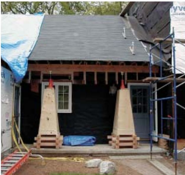
Figure 11. The screw jacks were limited to a 10-inch lifting range, so the jacking stands had to be supplemented with 4x4 cribbing placed in crosswise layers under the base.
