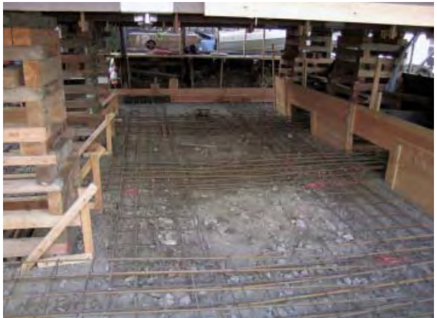
Figure 4. The concrete sub used a skid steer to excavate a flat surface for the grid to sit on (top). Next, his crew formed the perimeter (above), then laid and tied all the steel before forming the inner parts of the grid (right).
