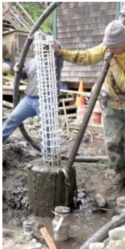
Figure 11. The crew pumped from the bottom up to prevent concrete from mixing with the water in the hole (left). The casing was pulled out as the concrete was poured. Below left, a welder cuts off a section that had just come out of the ground. The silt pouring out of the top indicates that this hole was nearly filled with concrete (below right).
