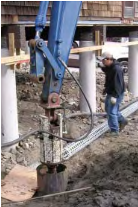
Figure 10. Before pouring a pier, the drilling contractor redrilled the bottom of the hole to make sure it hadn't filled up with silt (above). Like the columns, the piers were heavily reinforced with galvanized rebar cages (right).
