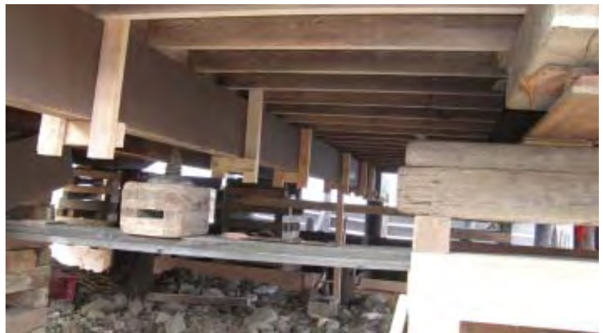
Figure 3. It was easier to install the beams before bringing the supports up from below. Here, the beam is hung from the joists before installation of the support columns.
