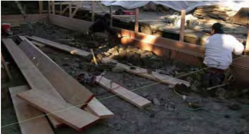
Figure 4. The concrete sub used a skid steer to excavate a flat surface for the grid to sit on (top). Next, his crew formed the perimeter (above), then laid and tied all the steel before forming the inner parts of the grid (right).
