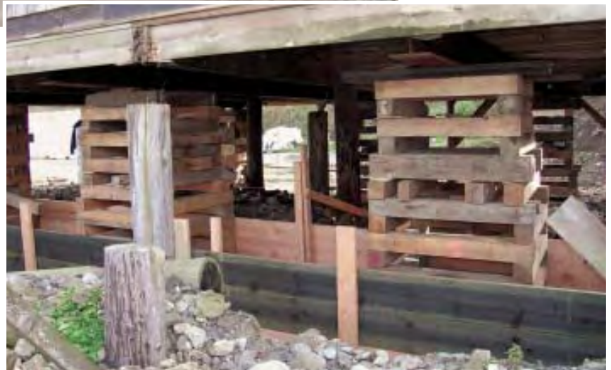
Figure 2. The crew members did not want to undermine the shoring when they dug down to repair damaged piles, so they excavated the areas where the cribbing would go, then built “forms” around the cribs to protect them from being buried if waves came under the house (below).
