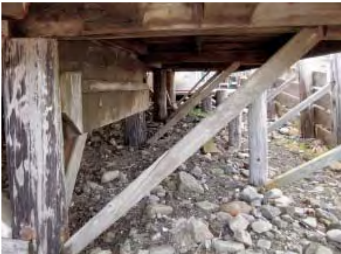
Figure 1. Creosote-treated wood piles supported the cottage 5 feet above the beach, so storm surge could flow under it. The decks were carried by shallow concrete piers (above left). About half of the piles showed signs of rot (left), as did most of the beams that carried the floor system and decks (above).
