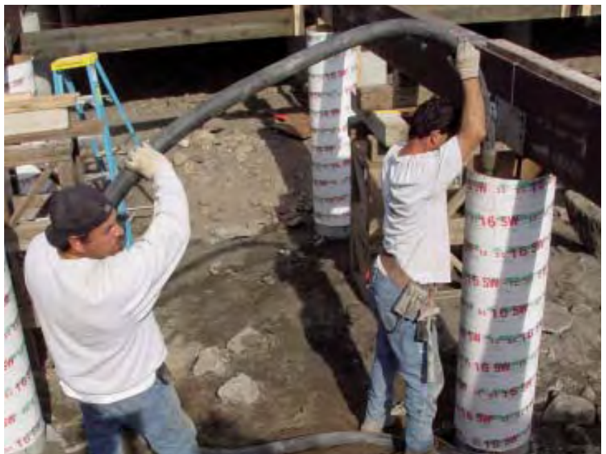
Figure 12. Once the piers were up to grade, members of the crew braced the deck support beams into position and installed the column caps (above). Then they formed up to the beam with Sonotubes and poured the rest of the way (right).
