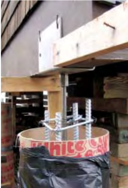
Figure 7. The threaded rod coming down from this column cap (above) is attached to a large nut and washer that will be embedded in the concrete. The Sonotube was lifted to within an inch or two of the beam before the concrete was poured, and the gap was later packed with grout. Because the column received a stuccolike waterproof coating, it's not possible to see the joint between the concrete and the grout (right).
