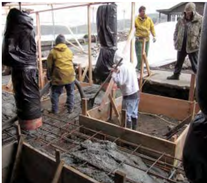
Figure 6. Access was poor, so the crew used a pump to place concrete for the grid (above) and columns (right).
