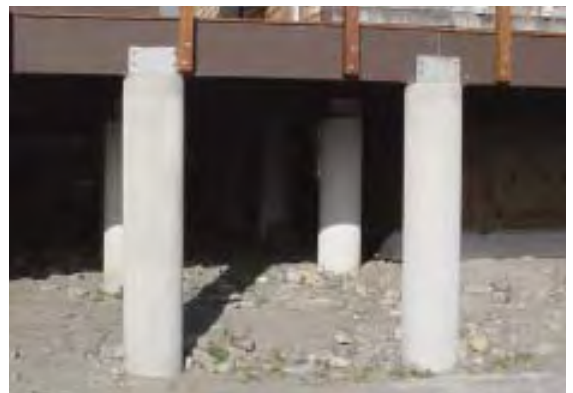
Figure 8. In the photo at left, the grid and columns are both visible. Once the foundation was backfilled, only the columns could be seen (above).
