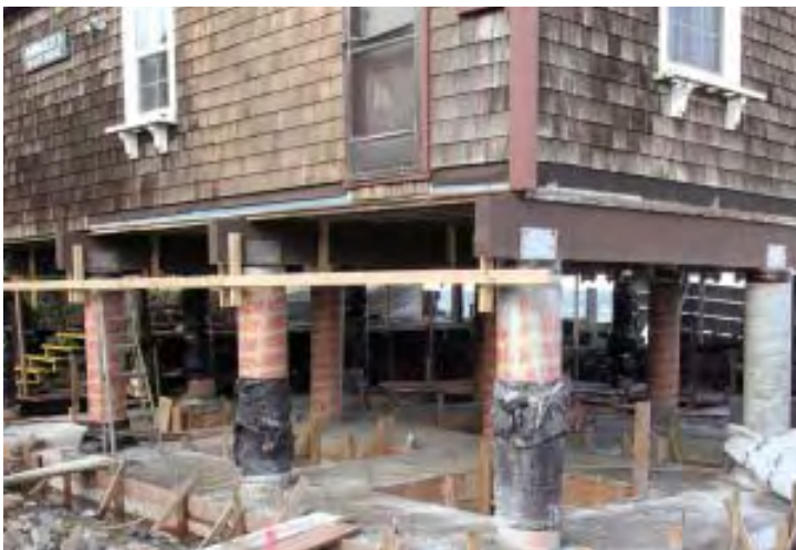
Figure 8. In the photo at left, the grid and columns are both visible. Once the foundation was backfilled, only the columns could be seen (above).
