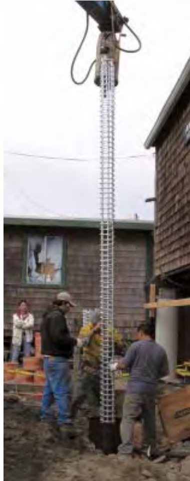
Figure 10. Before pouring a pier, the drilling contractor redrilled the bottom of the hole to make sure it hadn't filled up with silt (above). Like the columns, the piers were heavily reinforced with galvanized rebar cages (right).
