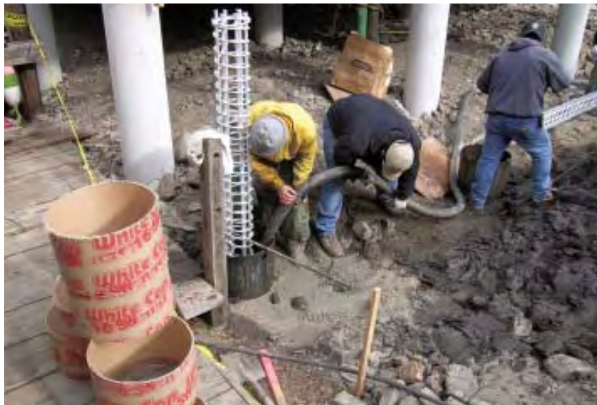
Figure 11. The crew pumped from the bottom up to prevent concrete from mixing with the water in the hole (left). The casing was pulled out as the concrete was poured. Below left, a welder cuts off a section that had just come out of the ground. The silt pouring out of the top indicates that this hole was nearly filled with concrete (below right).
