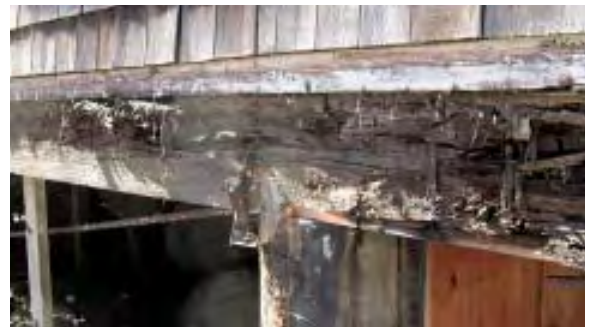
Figure 1. Creosote-treated wood piles supported the cottage 5 feet above the beach, so storm surge could flow under it. The decks were carried by shallow concrete piers (above left). About half of the piles showed signs of rot (left), as did most of the beams that carried the floor system and decks (above).
