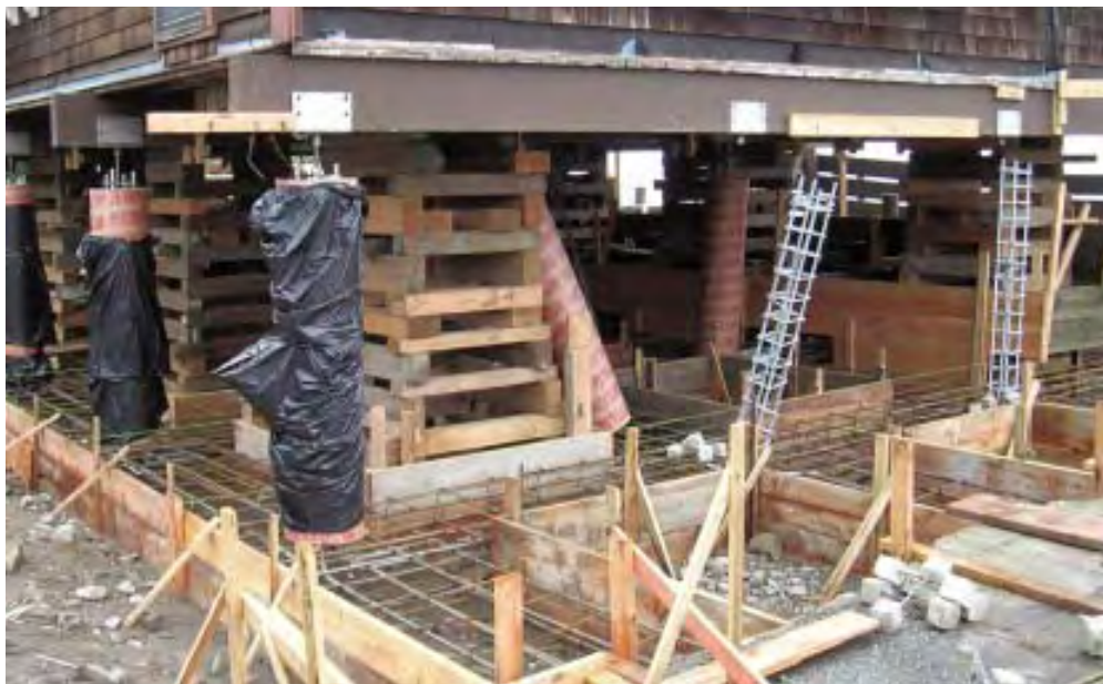
Figure 5. Once the steel was tied, crew members finished the formwork by boxing out the grid openings with 2-by-lumber, then installed the rebar cages for the columns. They wrapped the Sonotubes with plastic to protect them from exposure to heavy rain.
