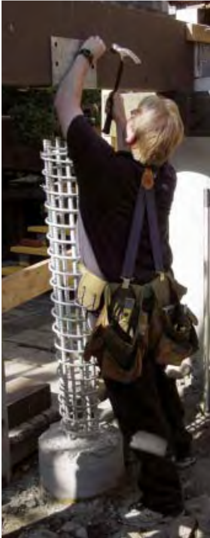
Figure 12. Once the piers were up to grade, members of the crew braced the deck support beams into position and installed the column caps (above). Then they formed up to the beam with Sonotubes and poured the rest of the way (right).
