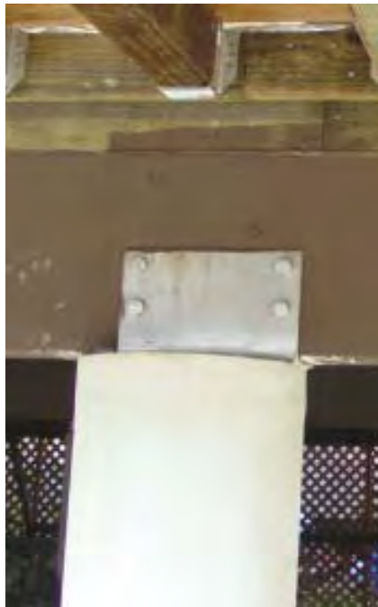
Figure 7. The threaded rod coming down from this column cap (above) is attached to a large nut and washer that will be embedded in the concrete. The Sonotube was lifted to within an inch or two of the beam before the concrete was poured, and the gap was later packed with grout. Because the column received a stuccolike waterproof coating, it's not possible to see the joint between the concrete and the grout (right).
