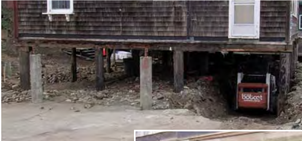
Figure 2. The crew members did not want to undermine the shoring when they dug down to repair damaged piles, so they excavated the areas where the cribbing would go, then built “forms” around the cribs to protect them from being buried if waves came under the house (below).
