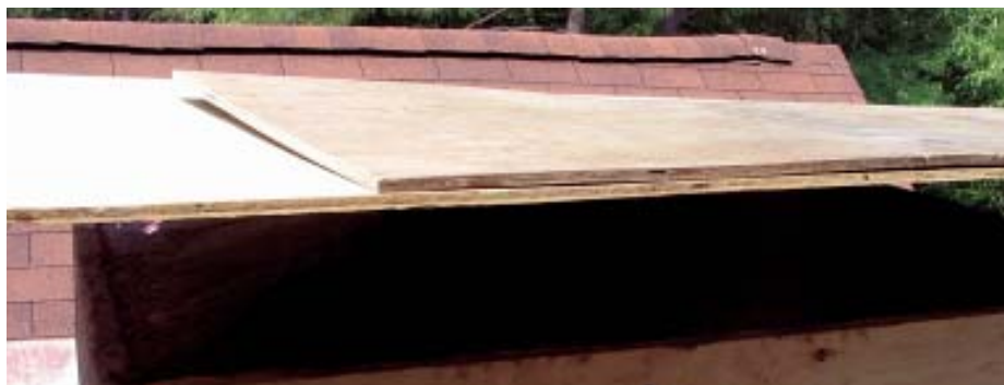
Figure 11. Plywood placed on top of the flue prevented the hot sun from accelerating the cure of the newly poured concrete cap (left). After the initial set, the author covered the cap with wet burlap (below left), then wrapped the top with plastic held in place with bar clamps (below), a procedure repeated for three successive nights to promote proper curing of the concrete.
