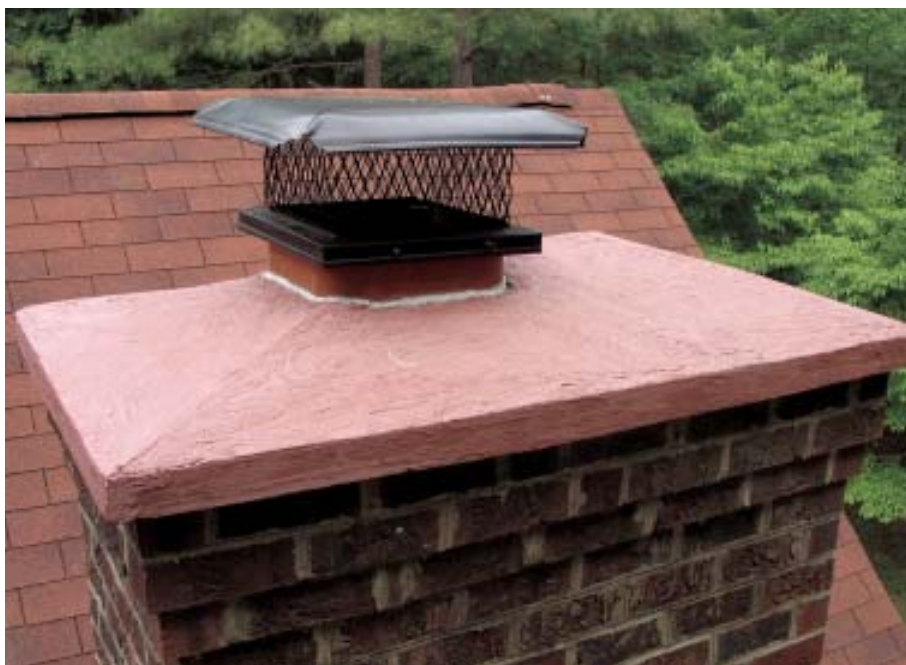
Figure 12. Rubbed with a colored cement-and-sand slurry that was applied with an abrasive stone, the finished chimney cap has a textured finish. It should last as long as the chimney it protects.
