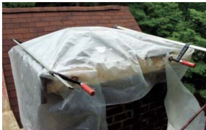
Figure 11. Plywood placed on top of the flue prevented the hot sun from accelerating the cure of the newly poured concrete cap (left). After the initial set, the author covered the cap with wet burlap (below left), then wrapped the top with plastic held in place with bar clamps (below), a procedure repeated for three successive nights to promote proper curing of the concrete.
