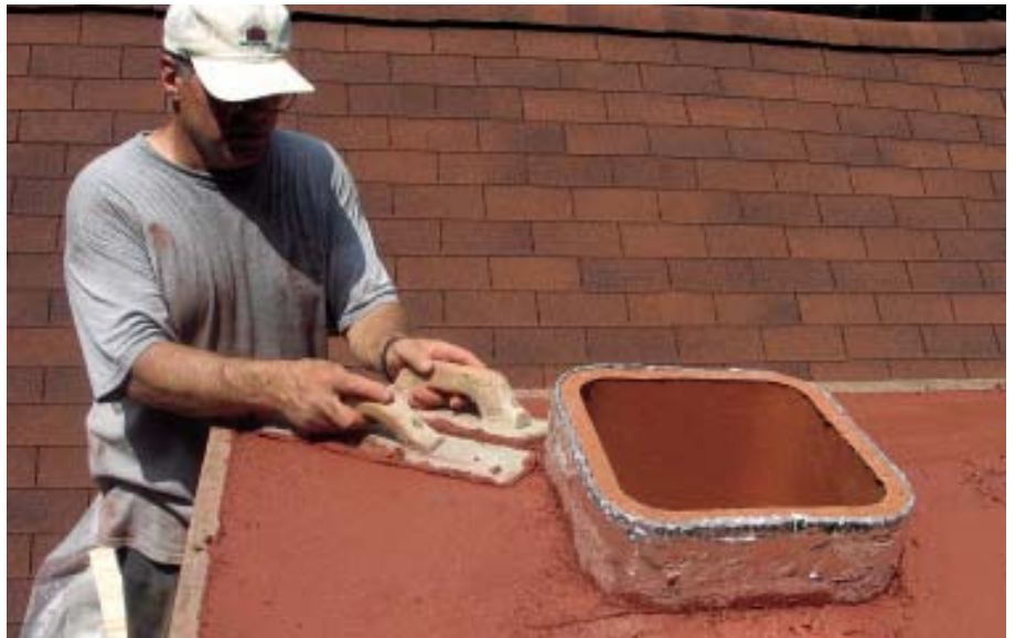
Figure 10. To create the hips of the chimney cap, the author used two floats. He pushed the concrete into position and smoothed out high and low spots so that the cap would easily drain water away from the flue.
