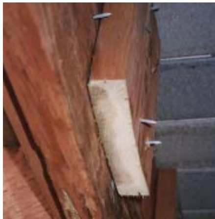
Figure 1. Pressure-treated hem-fir lumber is incised to increase penetration, but often the colored preservative barely soaks in at all, as is evident on this piece of blocking. The end cut should have been coated with preservative; the brown staining visible on the end grain is a sign of rot.
