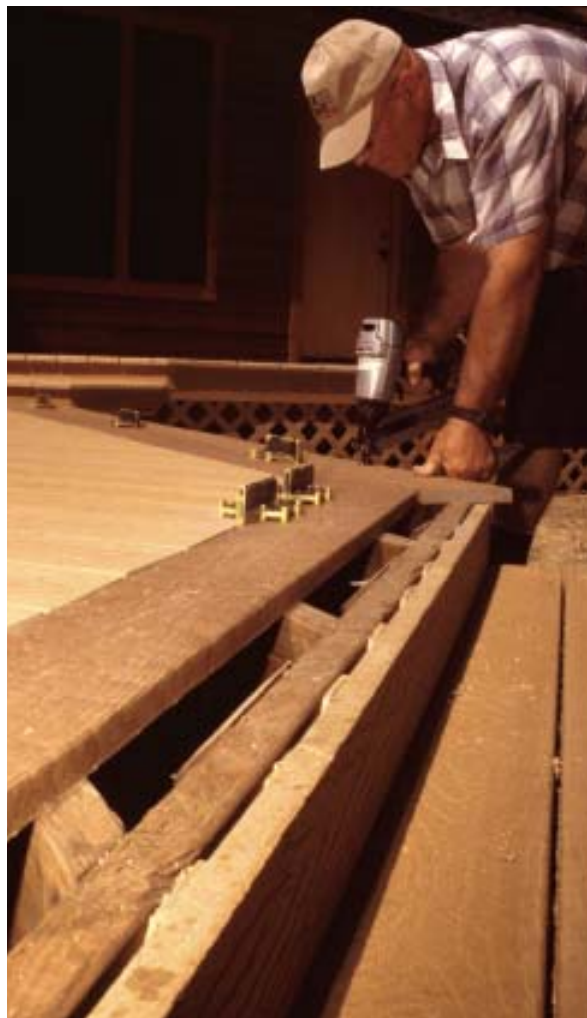
Figure 2. On this deck (above), water got between the fascia and rim, partially rotting the fascia and completely destroying the rim. When the fascia was removed, the rim collapsed. Here (right), the author installs composite decking on a pressure-treated frame that will completely cover the fascia and rim, avoiding this potential collection zone. The lattice separating the fascia and rim joist will also help to drain away water.
