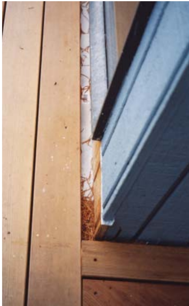
Figure 4. Although it's common practice to bring an L-shaped flashing down the wall and kick it out over the ledger, the resulting pocket can collect debris and rot both the decking and the siding above.
