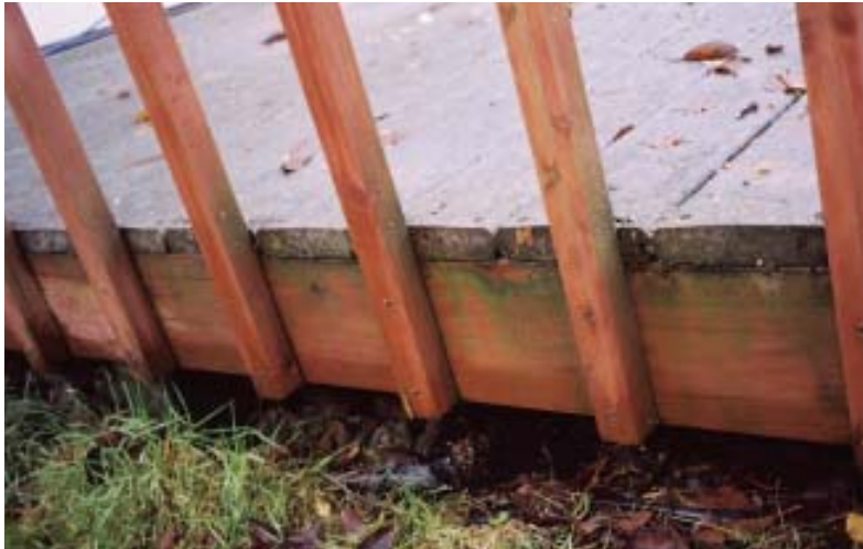
Figure 7. Nailing balusters to the rim joist creates pockets that trap moisture and debris, which can cause rot (below).
