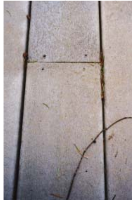
Figure 6. Most carpenters space deck boards too tightly (above), leaving enough room for debris to get in but no way to clean it out. On this deck, organic matter collected at every gap and joint (above left), as well as between a rim joist and blocking that landed under a gap in the deck boards (left).
