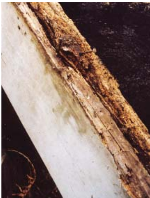
Figure 2. On this deck (above), water got between the fascia and rim, partially rotting the fascia and completely destroying the rim. When the fascia was removed, the rim collapsed. Here (right), the author installs composite decking on a pressure-treated frame that will completely cover the fascia and rim, avoiding this potential collection zone. The lattice separating the fascia and rim joist will also help to drain away water.
