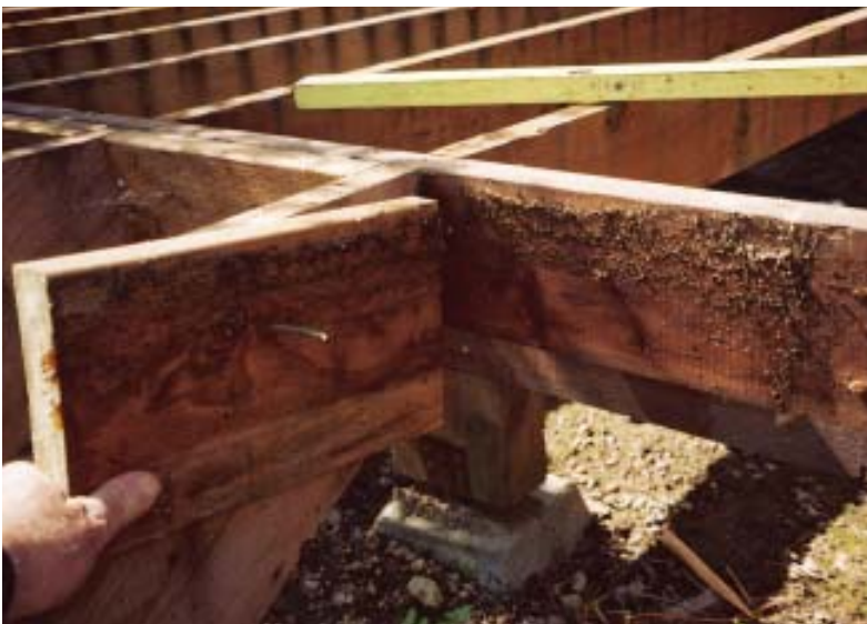
Figure 6. Most carpenters space deck boards too tightly (above), leaving enough room for debris to get in but no way to clean it out. On this deck, organic matter collected at every gap and joint (above left), as well as between a rim joist and blocking that landed under a gap in the deck boards (left).
