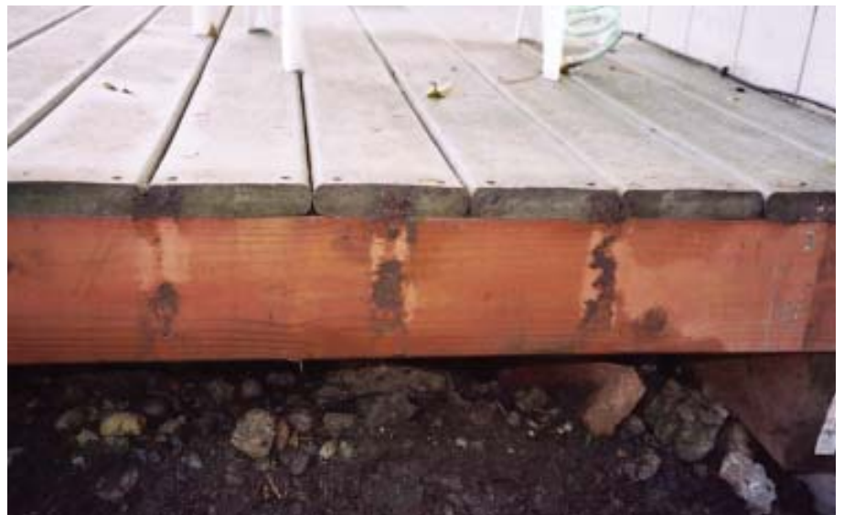
Figure 7. Nailing balusters to the rim joist creates pockets that trap moisture and debris, which can cause rot (below).
