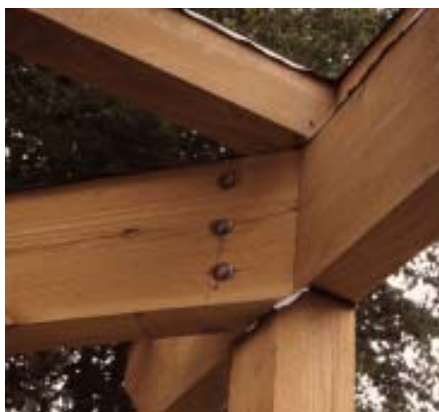
Figure 9. To keep this deck — which is framed with untreated lumber — from rotting, the author coated it with a borate preservative and covered the upper surfaces with torch-down roofing membrane.
