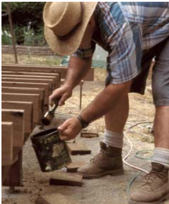
Figure 9. To keep this deck — which is framed with untreated lumber — from rotting, the author coated it with a borate preservative and covered the upper surfaces with torch-down roofing membrane.
