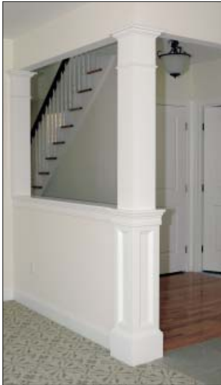
FIGURE 3: While durable on the exterior, PVC has advantages for interior woodwork as well. The author uses it for interior columns, preassembling a boxed column and then installing it around a structural post.
