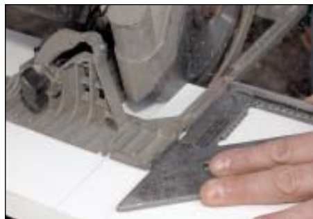
FIGURE 1: PVC trim stock cuts and routs much like wood. The dust tends to have a static cling, but it's not as fine or as abrasive as fiber-cement dust. PVC trim also won't dull blades any faster than wood.
