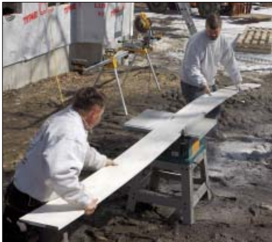
FIGURE 4: PVC trim stock is much more flexible than wood of comparable dimension. It will sag on a table saw, so two people are needed to rip it. To demonstrate the material's flexibility, the author ties a 1-inch-wide strip into a pretzel.
