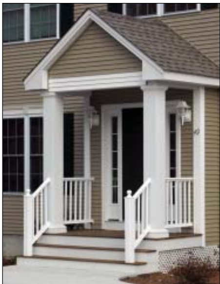
FIGURE 2: PVC material has no organic material, so it is not prone to rot. This makes it ideal for coastal homes. Not only will all exterior trim, including everything on this entry (above), hold up to wind and high humidity, but it also is an excellent material for outside showers (right). The author even shapes the soap dish from PVC.
