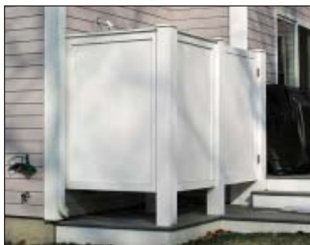
FIGURE 2: PVC material has no organic material, so it is not prone to rot. This makes it ideal for coastal homes. Not only will all exterior trim, including everything on this entry (above), hold up to wind and high humidity, but it also is an excellent material for outside showers (right). The author even shapes the soap dish from PVC.
