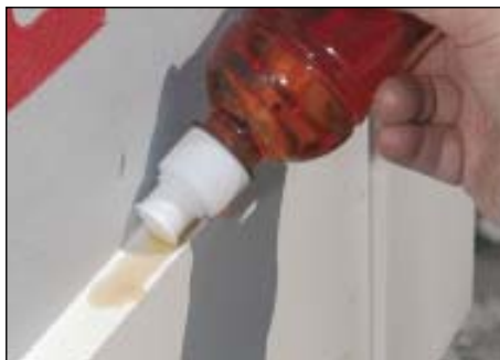
FIGURE 6: While plumber's PVC cement will bond trim stock, the author prefers Gorilla brand PVC glue — a water-based product that doesn't yellow, and gives about five minutes' working time. He buys it in bulk and uses a water bottle to apply it.
