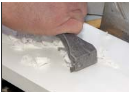
FIGURE 7: PVC trim holds paint much better than wood, and it will never require maintenance if left unpainted. Scratches, scuffs, and glue can be removed with a sharp scraper or light sanding.
