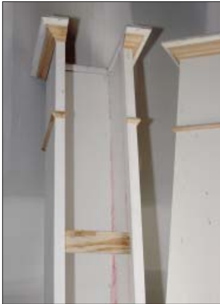
FIGURE 3: While durable on the exterior, PVC has advantages for interior woodwork as well. The author uses it for interior columns, preassembling a boxed column and then installing it around a structural post.
