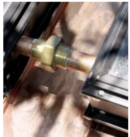
Figure 12. A pumped system typically contains more than one flat-plate collector (left). To allow for easy installation and repair, the author joins the collectors with unions (above).
