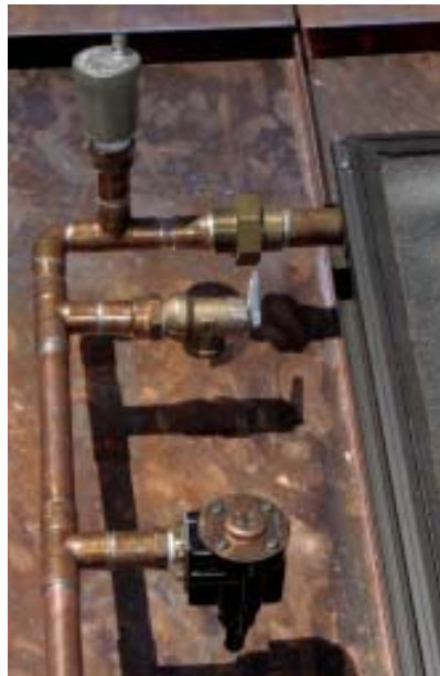
Figure 13. When this system is up and running, the gauges (top) will show how much heat the water gains as it passes through the collectors. Because the water may become too hot to safely use, the author always installs a tempering valve to prevent scalding (above left). A pressure-relief valve (in the center of the photo above right) opens if the collector itself gets too hot; the cylindrical valve at the top automatically bleeds air from the system.
