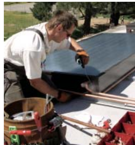
Figure 2. Integral collector storage — or ICS — units contain 4-inch-diameter pipes in which water is heated and stored (far left). Because of their weight, they are typically craned into place (left). Potable water enters through a pipe at the lower end, is heated by the sun, and exits through the upper end (above) when a hot-water tap is turned on.
