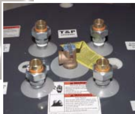
Figure 3. An installer plumbs an 80-gallon storage tank for a pumped system (left). The tank has taps for supply and return lines to and from the collector, plus a cold-water supply inlet and a hot-water outlet to the home (below).
