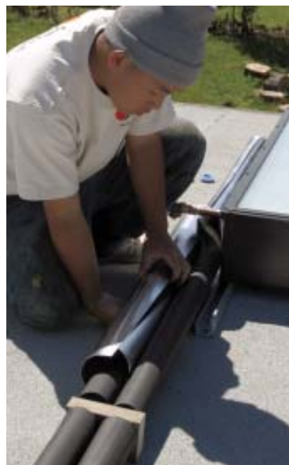
Figure 14. The author’s crew insulates every pipe that contains hot or warm water. Here, an installer protects the neoprene insulation with an aluminum jacket.
