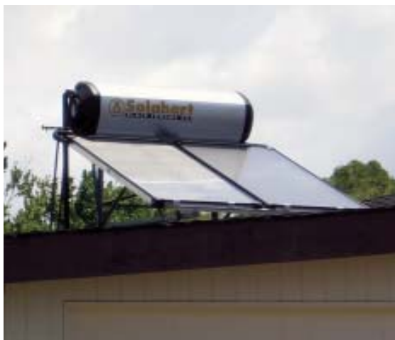
Figure 7. Because it's located in a warm climate, this thermosiphon unit contains potable water. Closed-loop thermosiphon systems containing glycol are also available for areas where freezing temperatures are common.
