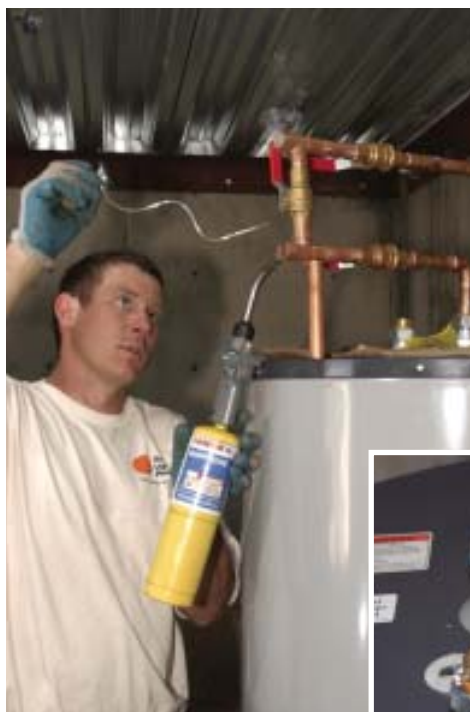
Figure 3. An installer plumbs an 80-gallon storage tank for a pumped system (left). The tank has taps for supply and return lines to and from the collector, plus a cold-water supply inlet and a hot-water outlet to the home (below).
