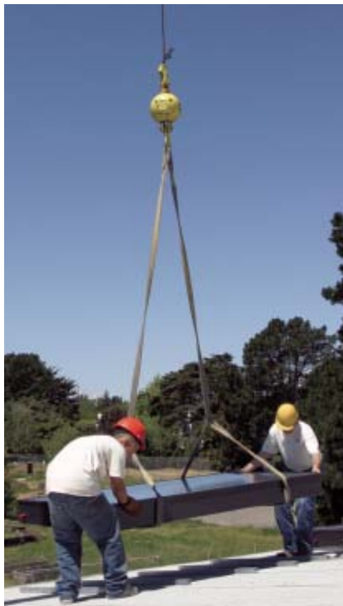
Figure 2. Integral collector storage — or ICS — units contain 4-inch-diameter pipes in which water is heated and stored (far left). Because of their weight, they are typically craned into place (left). Potable water enters through a pipe at the lower end, is heated by the sun, and exits through the upper end (above) when a hot-water tap is turned on.
