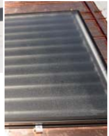
Figure 1. Flat-plate collectors range in size from 3 by 6 feet to 4 by 12 feet and are light enough to be carried by hand (above). Because the tubing inside is of small diameter, even a large collector might contain only a gallon or two of fluid.
