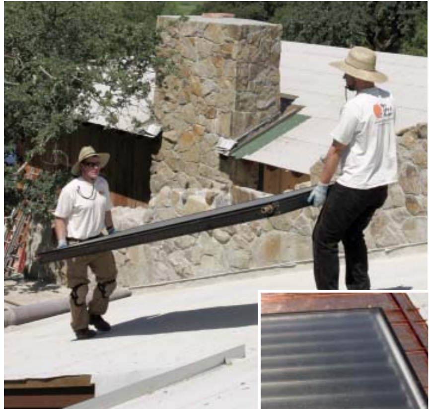
Figure 1. Flat-plate collectors range in size from 3 by 6 feet to 4 by 12 feet and are light enough to be carried by hand (above). Because the tubing inside is of small diameter, even a large collector might contain only a gallon or two of fluid.
