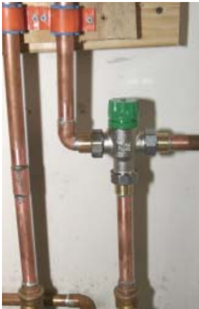
Figure 13. When this system is up and running, the gauges (top) will show how much heat the water gains as it passes through the collectors. Because the water may become too hot to safely use, the author always installs a tempering valve to prevent scalding (above left). A pressure-relief valve (in the center of the photo above right) opens if the collector itself gets too hot; the cylindrical valve at the top automatically bleeds air from the system.
