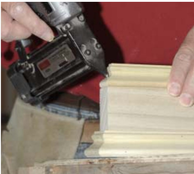
Figure 6. The 1x3 apron is wrapped with panel molding top and bottom (top). The author glues and pins the small pieces together with a 23-gauge headless pinner (above), then installs the apron in one piece (right).
