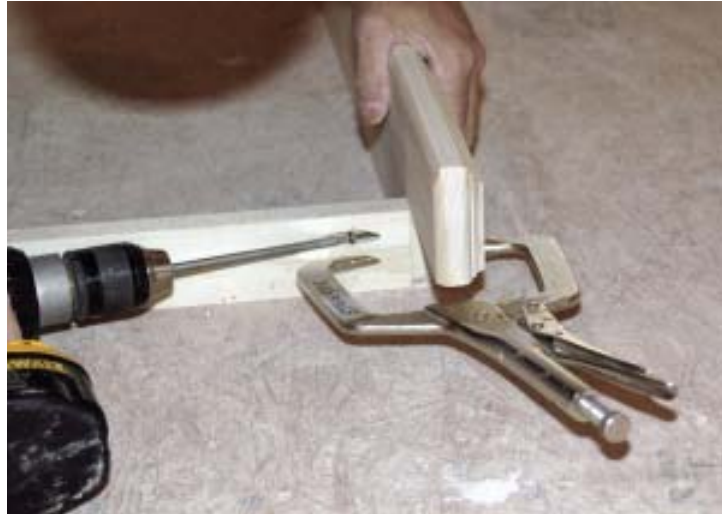
Figure 3. Pocket screws hold the jamb extensions together so they can be installed as a unit (left). On large windows the author attaches the stool with screws (below); on small ones he pins the stool to the side jambs from beneath.
