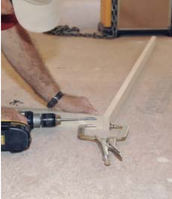
Figure 3. Pocket screws hold the jamb extensions together so they can be installed as a unit (left). On large windows the author attaches the stool with screws (below); on small ones he pins the stool to the side jambs from beneath.
