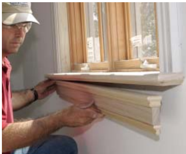
Figure 6. The 1x3 apron is wrapped with panel molding top and bottom (top). The author glues and pins the small pieces together with a 23-gauge headless pinner (above), then installs the apron in one piece (right).
