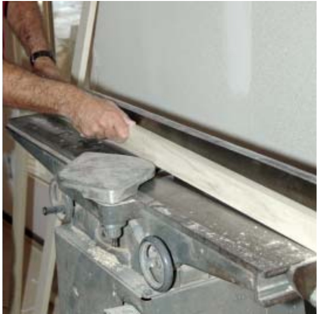
Figure 2. It helps to have the right tools: The author uses a table saw to cut the ears on the stool (left) and a jointer to taper the extensions so they match the plane of the drywall next to the window (below). A Kreg machine makes quick work of boring pocket holes (bottom).
